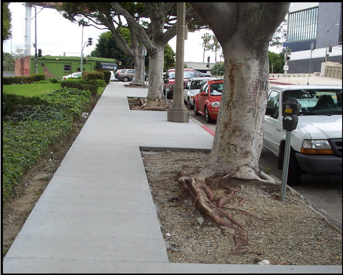
Figure 14 - The sidewalk cutout option can be used in some scenarios on downtown streets. The trees are shown before mulch was applied.
