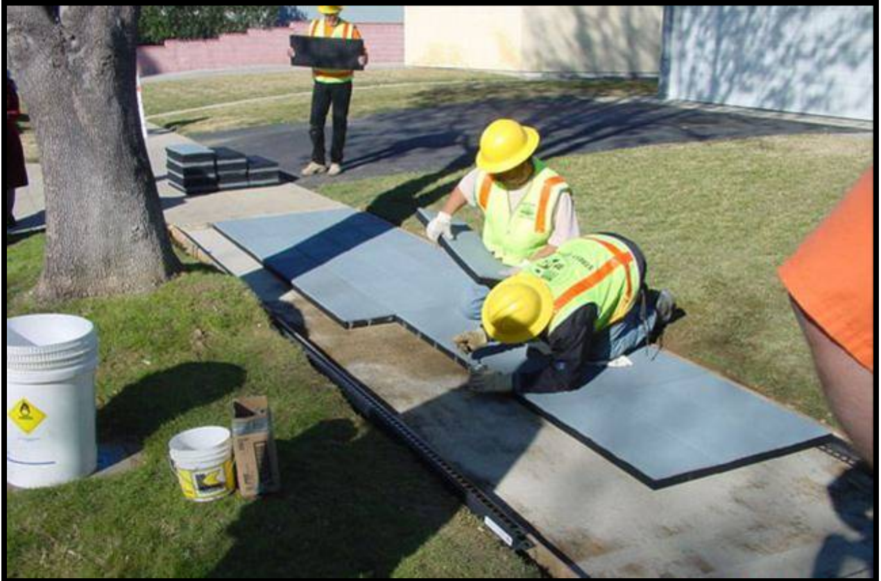
Figure 15 - Rubber sidewalk installation.
