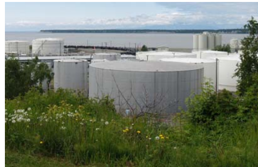
Tank farm at the Port of Anchorage
