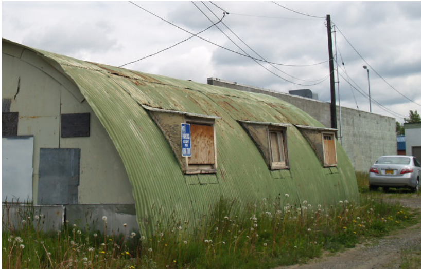
One of the original Quonset hut structures
