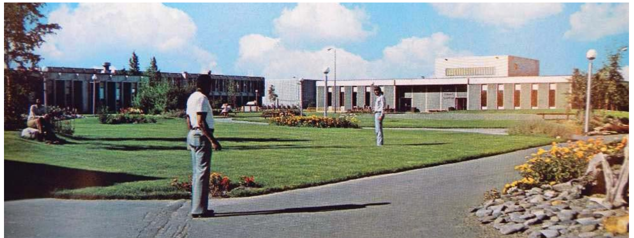
Figure 32. Original UAA campus buildings, 1978.
