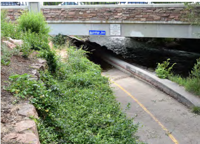
Grade separated crossing (undercrossing)
