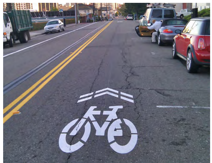
Shared use roadway/bicycle boulevard (sharrow)
