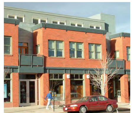
Use upper floor stepbacks, increased setbacks and wall offsets to vary a building’s massing.
