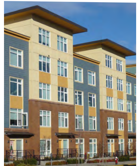
Use color changes, material changes and minor wall offsets to articulate a facade.
