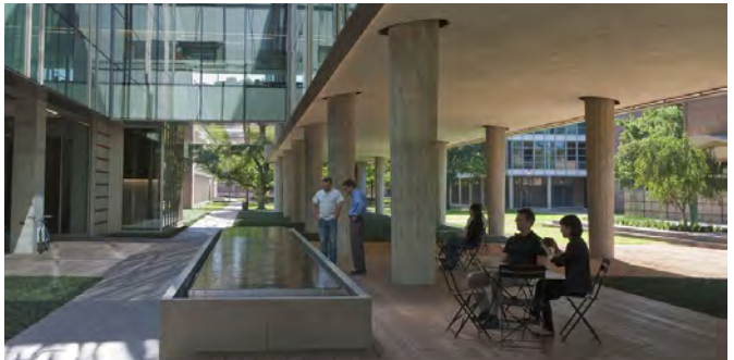
Multiuse building (outdoor courtyard and site circulation)
