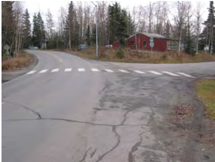
Before: 35th Avenue and McRae Road was a typical strip-paved “Spensard Street” with limited right-of-way and on-street parking. (photo courtesy of CRW Engineering Group)
