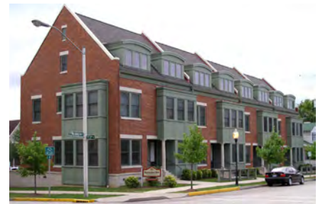
Use color changes, material changes and minor wall offsets to articulate a facade.
