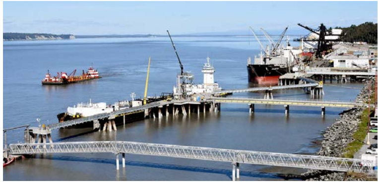
Figure 3. Port of Alaska Docks
