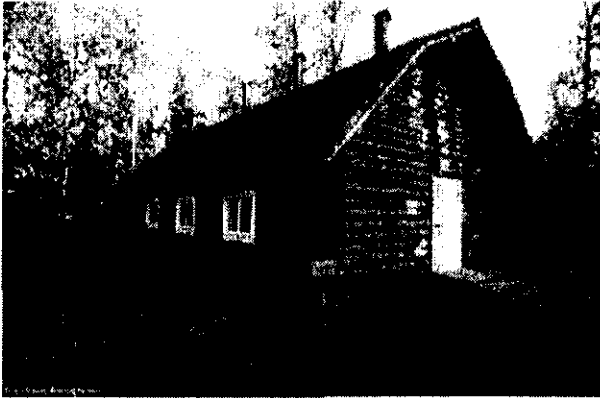
Rika's Roadhouse Restoration- Barn
