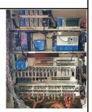
Traffic Signal Cabinet contains electrical equipment necessary for proper operation of signalized locations. Counters are installed inside cabinets.
