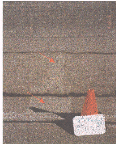
Photo 3 - 9th Ave., 4/18/96. Note sampling transect visible in street sweeping residue.
