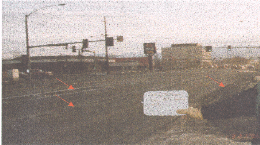
Photo 1 - 36th and Old Seward, 3/21/96. Note sediment concentrated in gutter, median, and between lanes.
