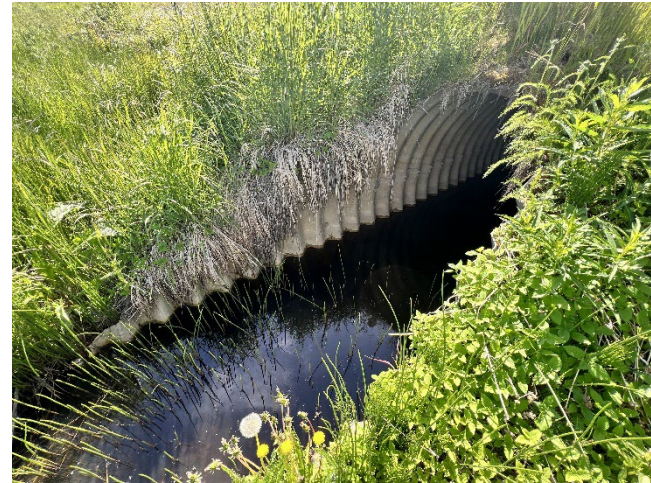
Culvert downstream of entire project area, where SWPPP team visually monitors discharge
