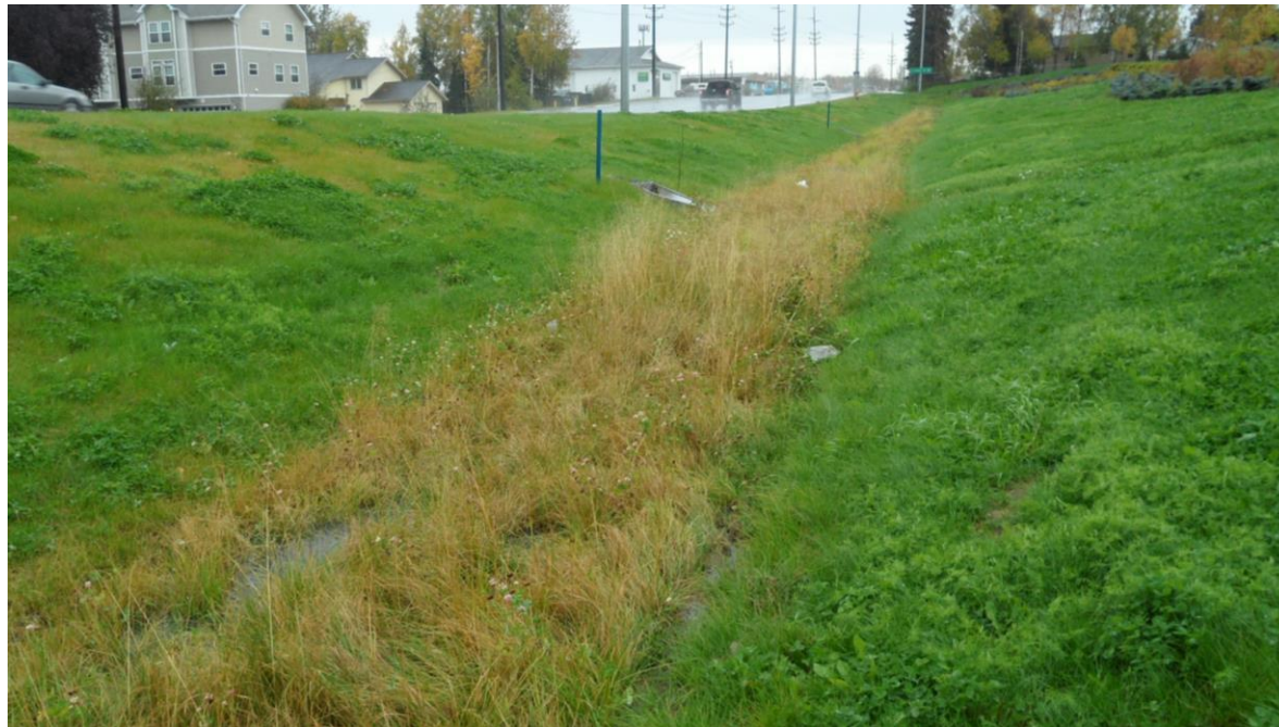
West Dowling Bioswale
