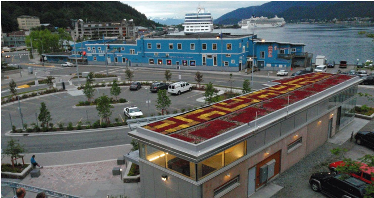
Juneau Transportation Center
