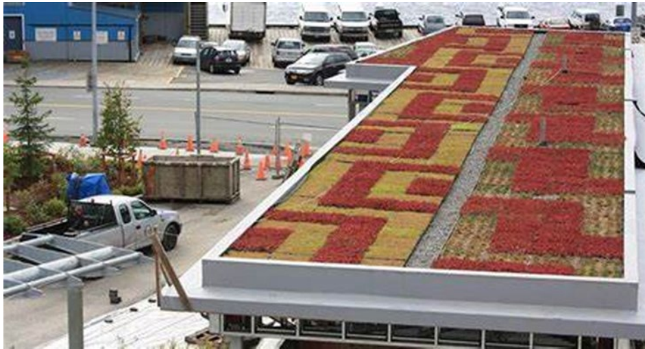
Juneau Transportation Center
