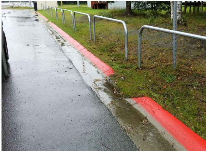
Above: Curb cut not functioning in Anchorage Upper Right: Stormwater Planter from the City of Salina, CA www.cityofsalinas.org/ Lower Right: Bioretention example from Chesapeake Bay Stormwater Network https://chesapeakestormwater.net/
