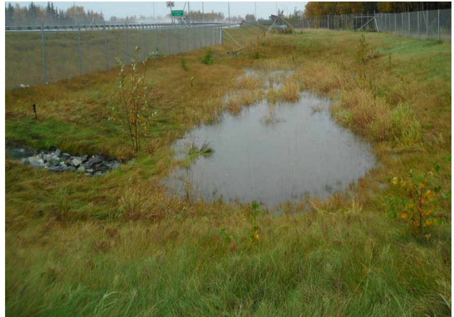
NSH/Alpenhorn infiltration facility. Accepting stormwater from nearly 7 acres of impervious surface.
