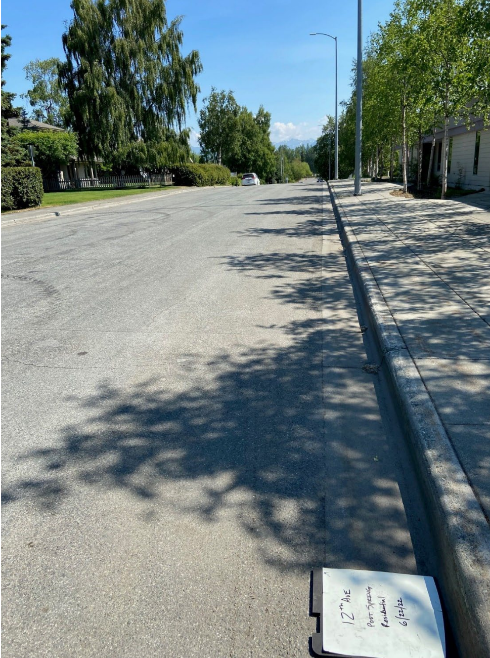
Figure 4-2 2022 'Visually Clean' Photo Example (Post Spring Sweep ARDSA 12thAve1)
