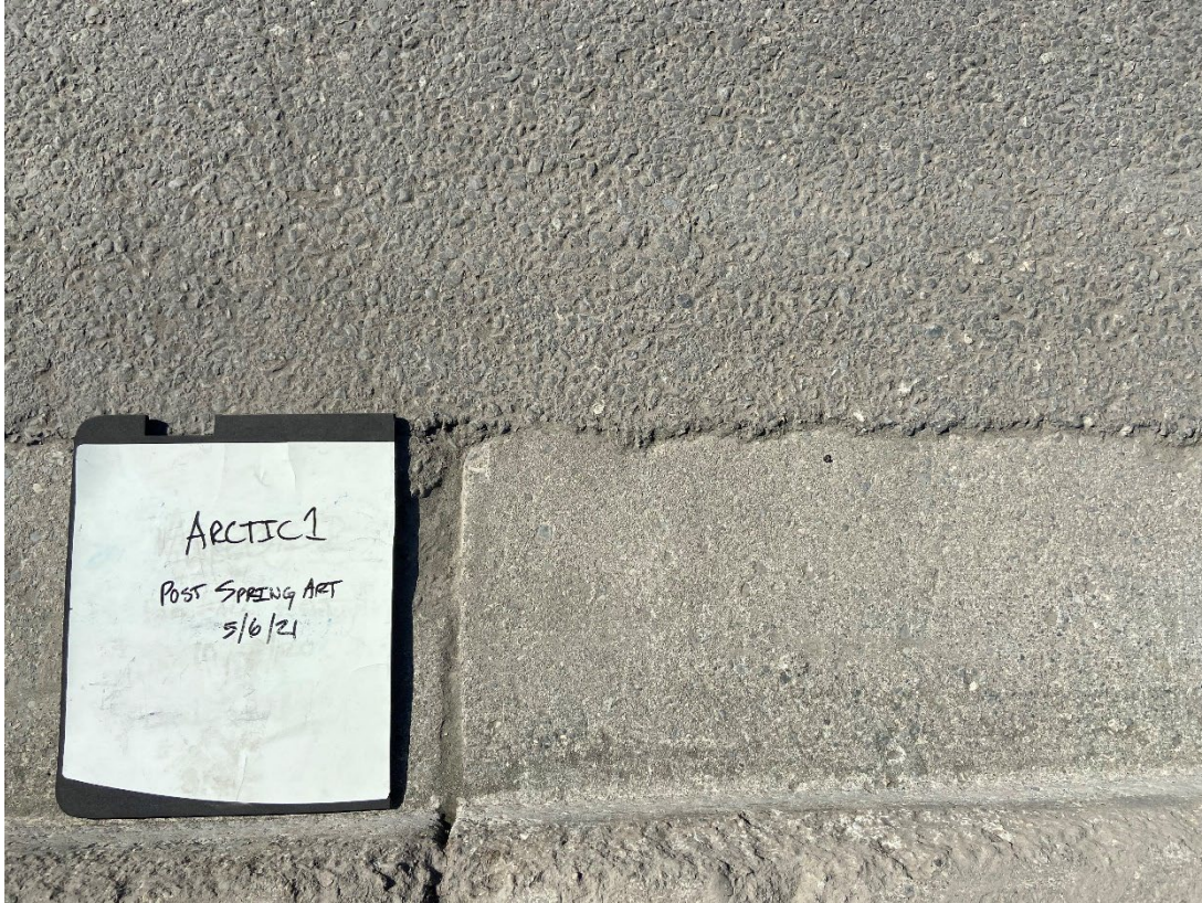
Figure 4-2 2021 'Visually Clean' Photo Example (Post Spring Sweep ARDSA Arctic1)
