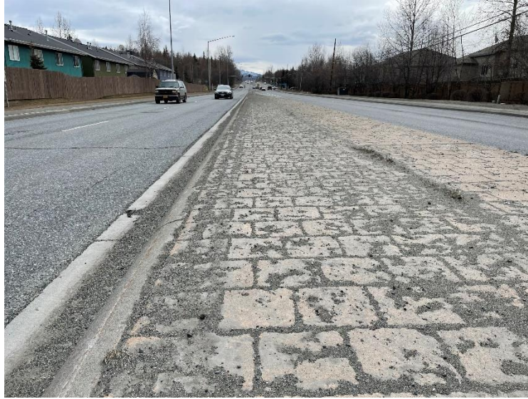
Figure 6.3 – Muldoon Rd before sweeping operations.
