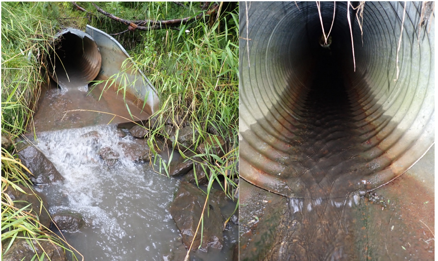
Photograph 10. Outfall SWM12 (1454-1), Lynwood Retention Basin.
