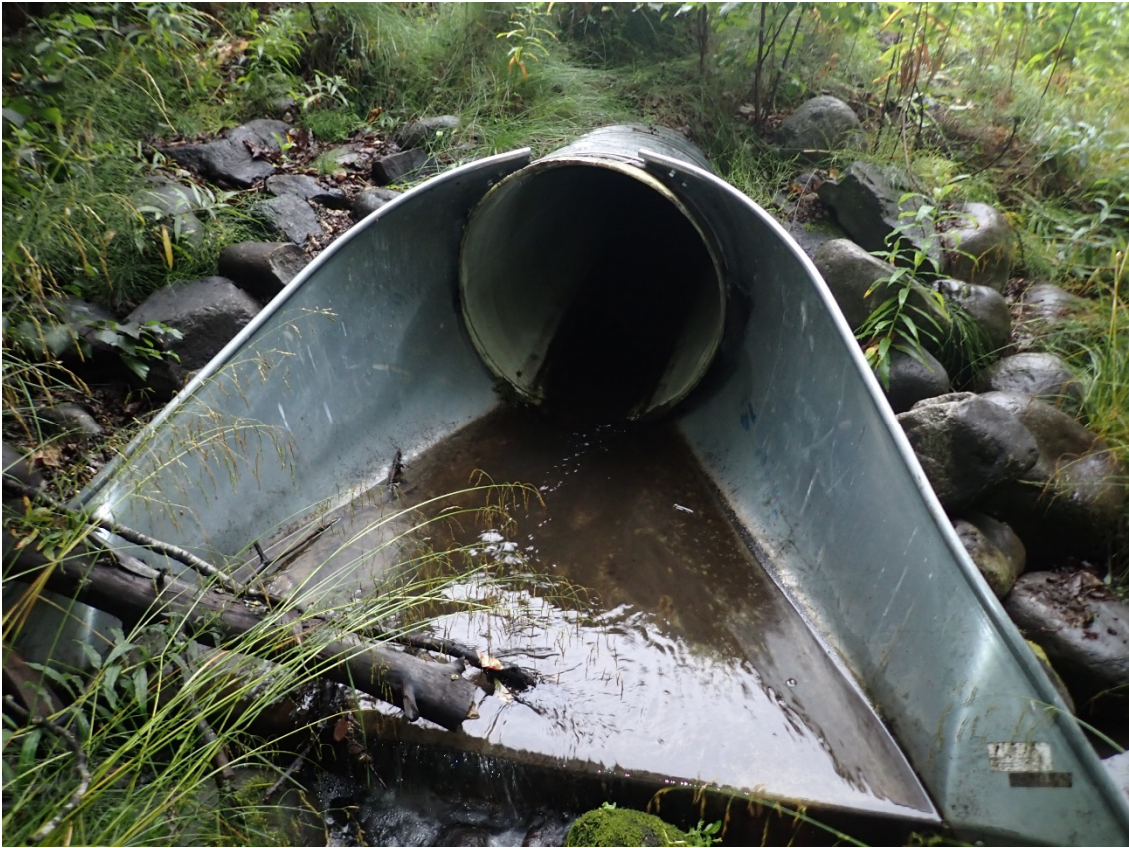
Photograph 1. Outfall SWM03 (1224-1), Fairweather Loop off Sylvan Drive.
