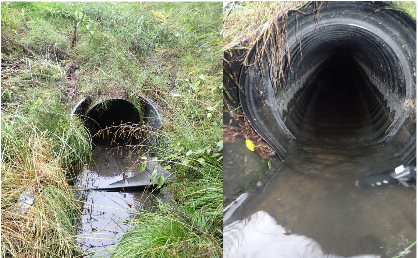
Photograph 2. Outfall SWM04 (1224-2), Fairweather Loop off Sylvan Drive.
