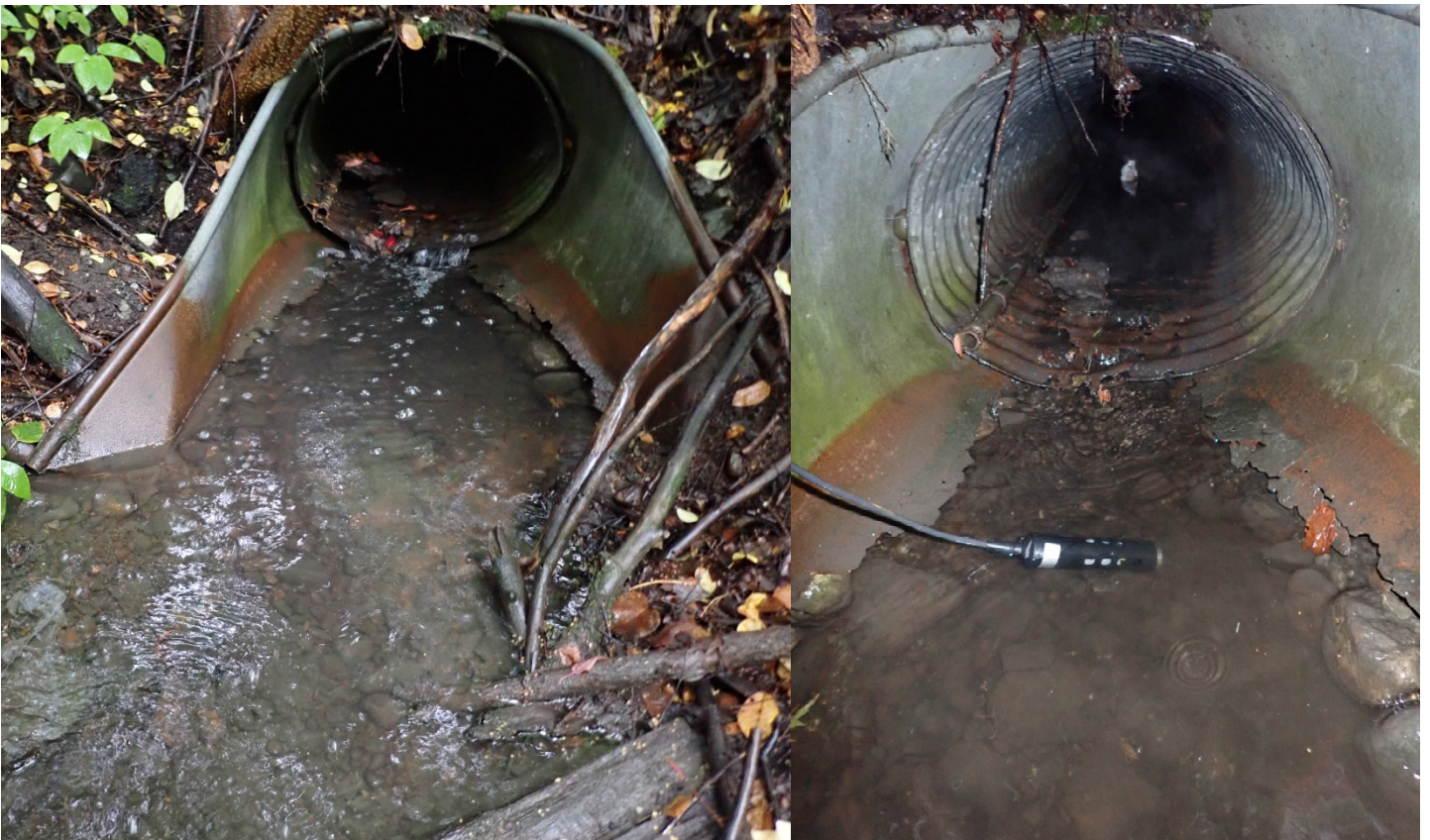
Photograph 4. Outfall SWM06 (314-22), Maplewood Street off of Northern Lights Boulevard.
