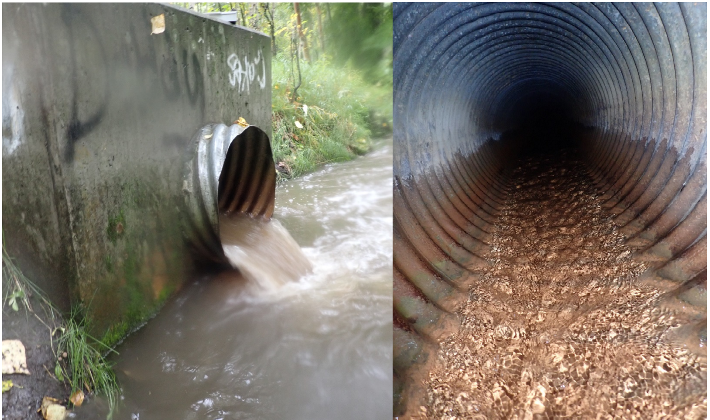
Photograph 8. Outfall SWM10 (525-2), Eagle Street at Chester Creek.
