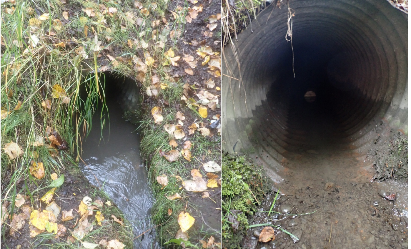
Photograph 7. Outfall SWM09 (499-1), Anchorage Football Stadium & Ben Boeke Ice Arena.
