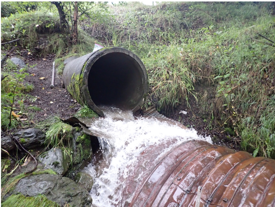
Photograph 6. Outfall SWM08 (86-1), New Seward Highway at Chester Creek.
