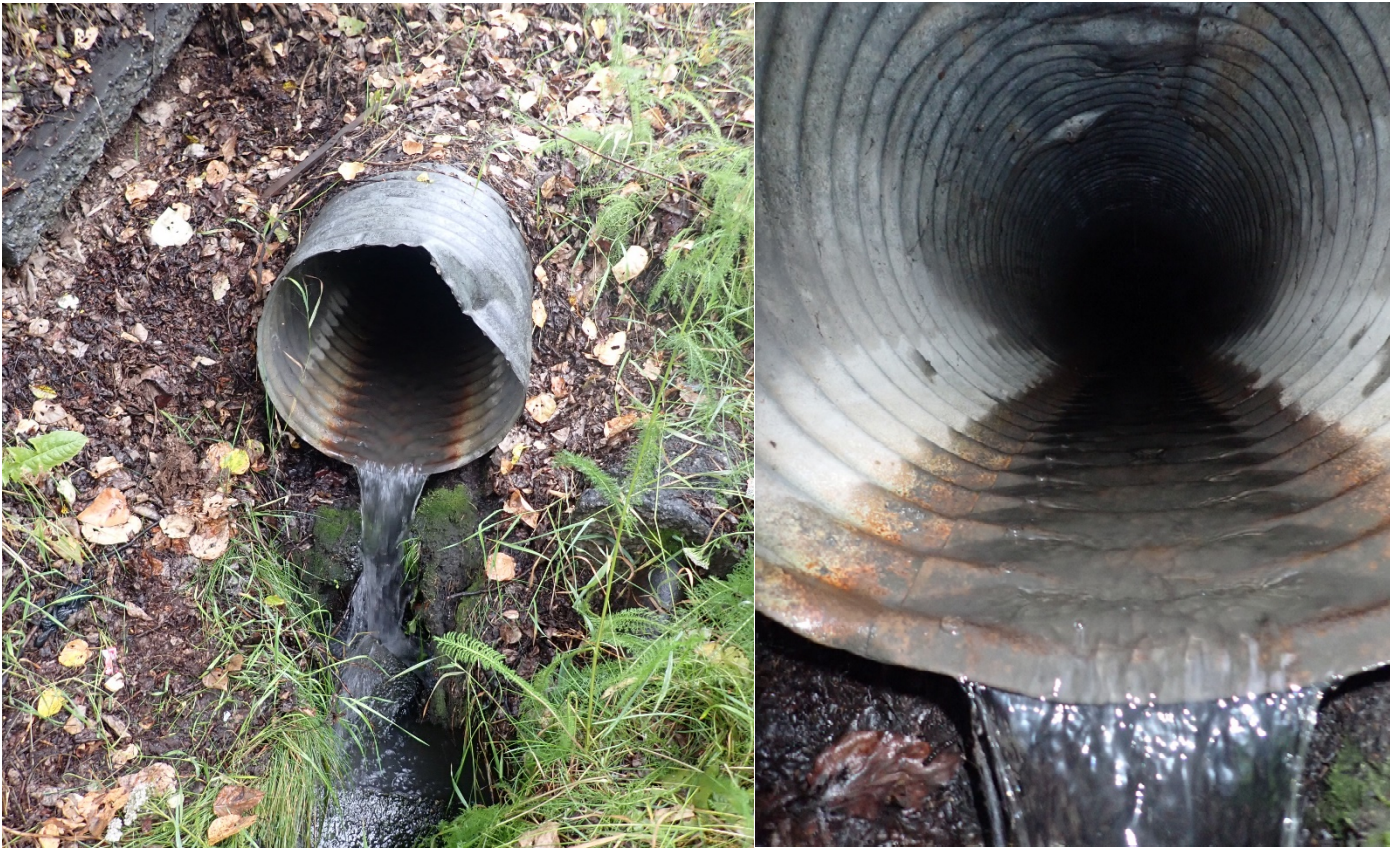
Photograph 5. Outfall SWM07 (484-1), New Seward Highway at Chester Creek.
