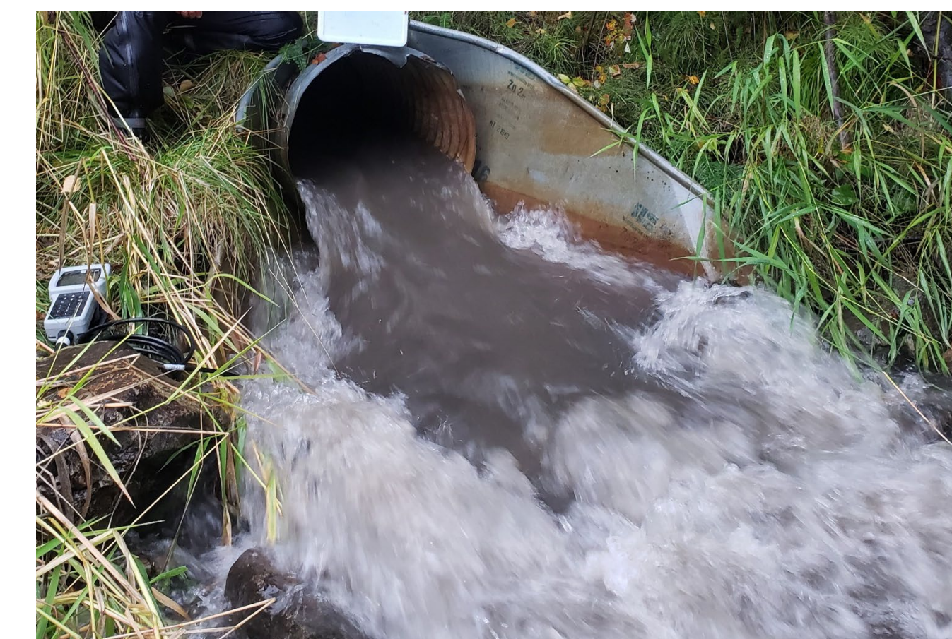
Outfall SWM12 (1454-1), Lynwood Retention Basin to Campbell Creek
