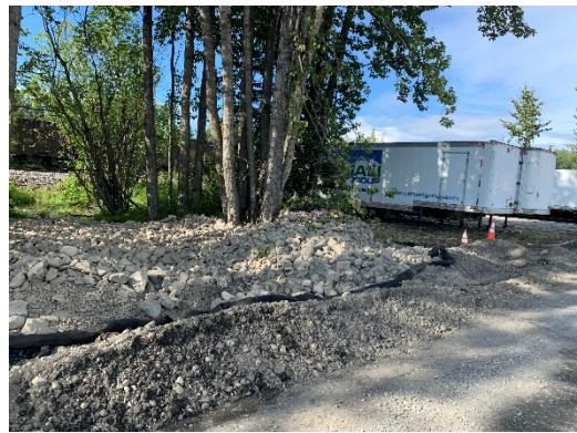
Composite Sock Used to Keep Sediment Off Vegetation
