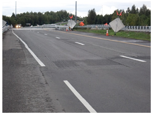
Milled, prepped for membrane and repaving; near Huffman Rd.
