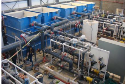
Homer Water Treatment Facility
