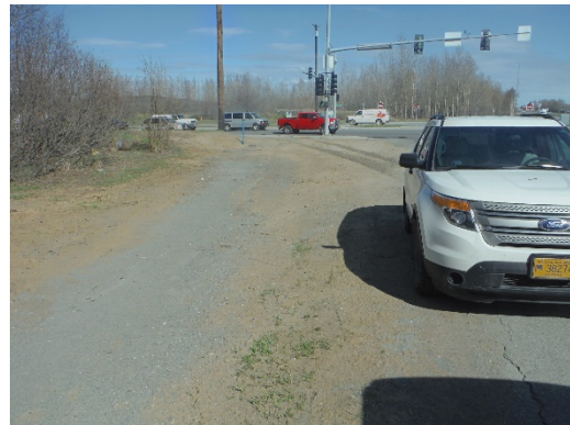
Active Construction Area, Will Be Seeded Later
