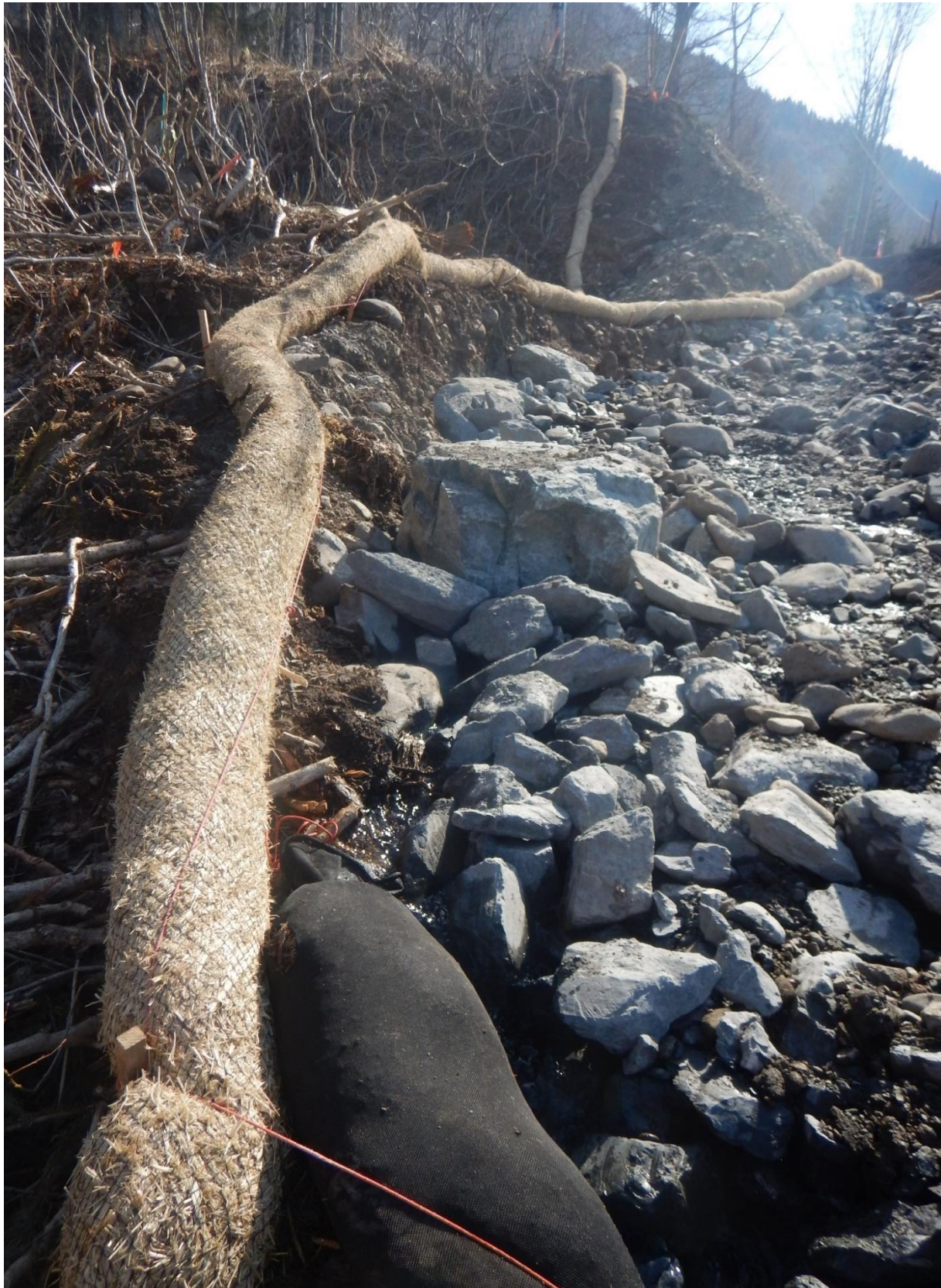
Figure 7. Subsurface flow in stream diversion adjacent to Indian Creek Bridge. View looking upstream.
