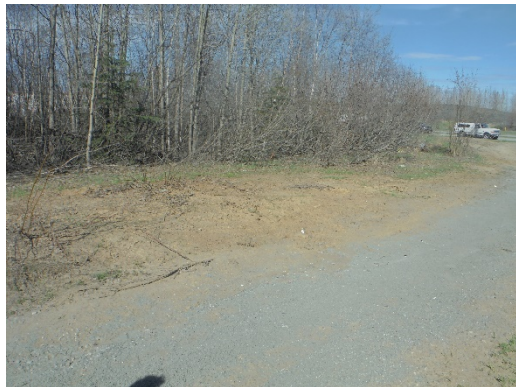
Mulch Laid Down As Winter Stabilization
