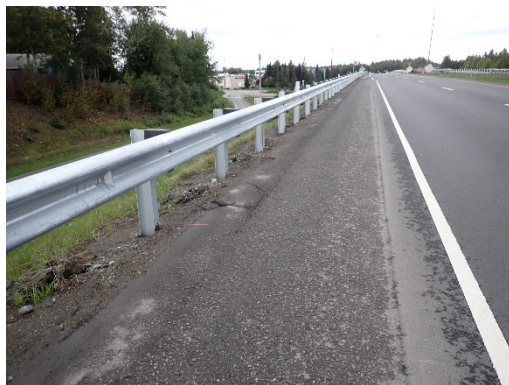
Repaved and guardrails replaced. Near O'Malley Rd.
