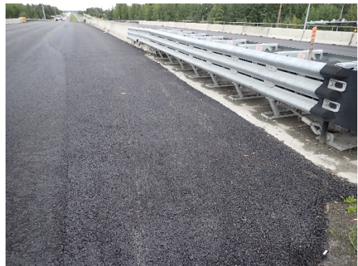
Repaved and guardrails replaced. Prepped for striping; near O'Malley Rd
