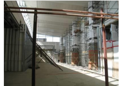
Anchorage International Airport Concourse C
