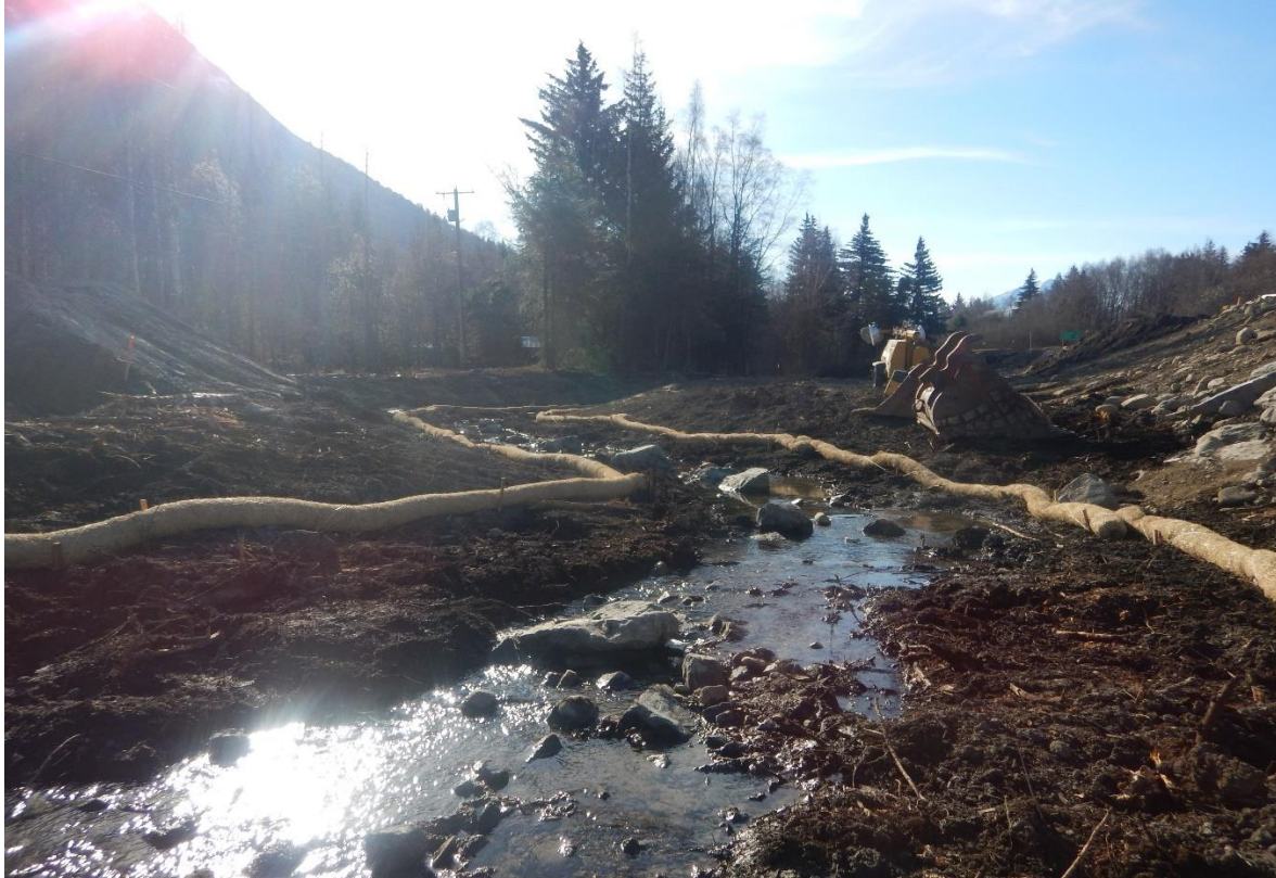
Figure 1. Bear Creek stream diversion upstream of Auriga Road. View looking upstream.
