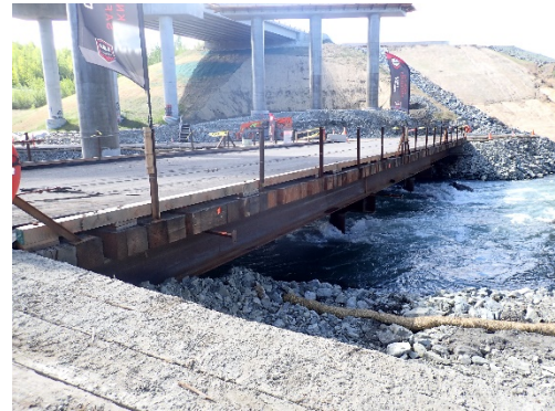
BMP Vehicle Dust Track Out Control – 18 of 20
