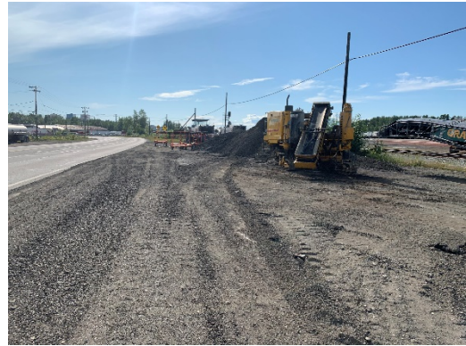
Entry Point, Ground Covered in RAP
