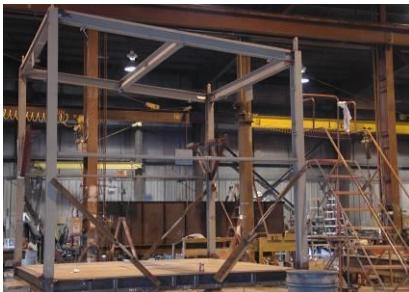
AES Fab Facility, Oilfield Piping and Module Inspection
