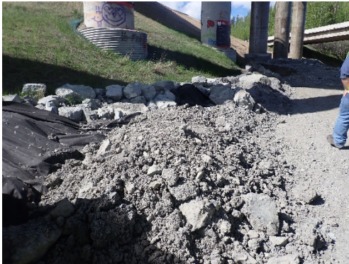
BMP Stockpile Stabilization Control – 17 of 20
