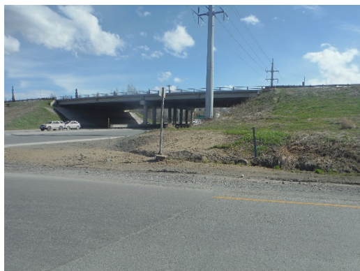
Hillside Track Walked And Mulched, Will Be Seeded Later
