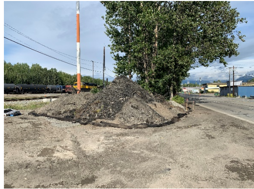
Stockpile with Composite Sock Wrapped Around Base
