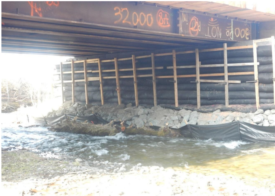
Figure 8. North bridge abutment on temporary bridge over Indian Creek.
