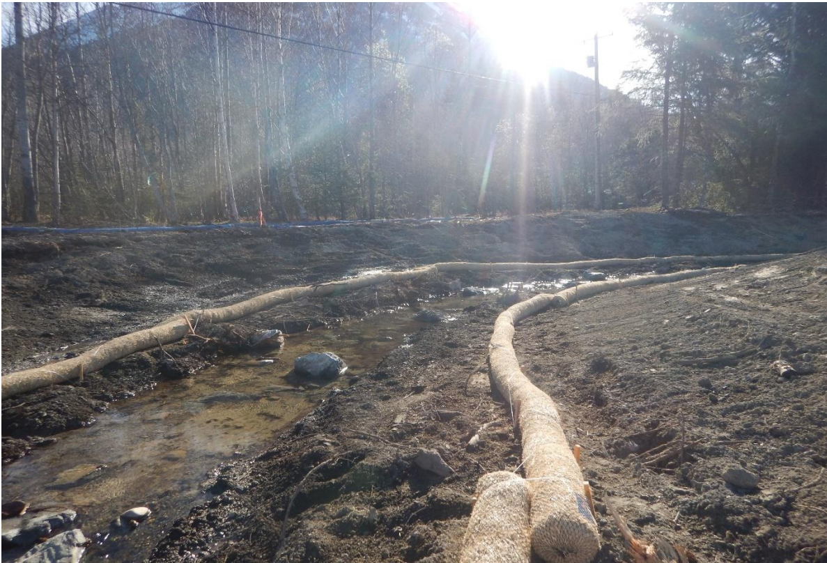
Figure 2. Bear Creek stream diversion upstream of Auriga Road. View looking upstream.
