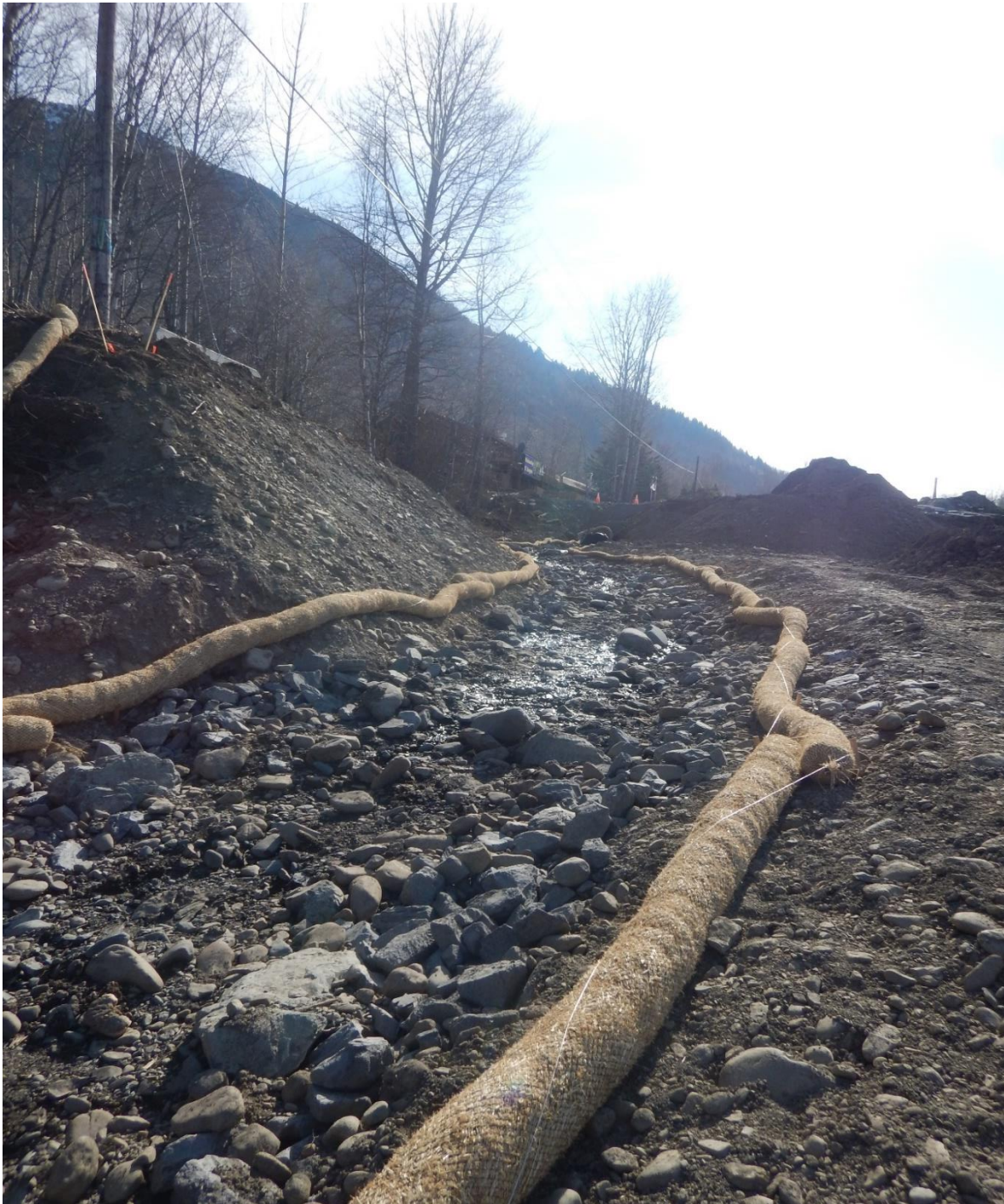
Figure 6. Subsurface flow in stream diversion adjacent to Indian Creek Bridge. View looking upstream
