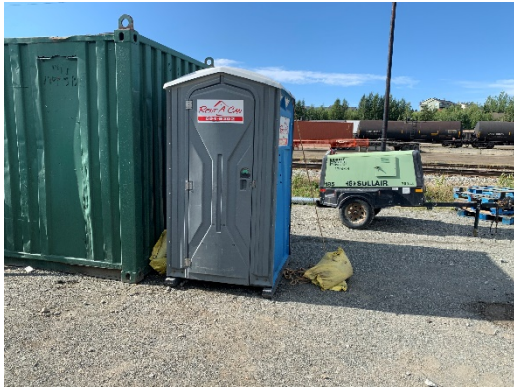
Porta-Potty, Secured and Far Removed From Water Body
