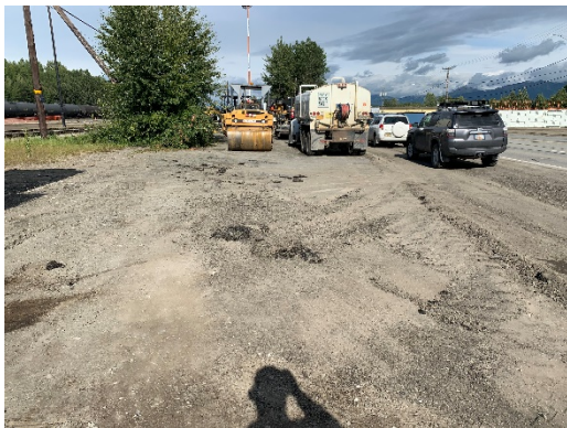
Entry Point, Ground Covered in Recycled Asphalt Pavement (RAP)
