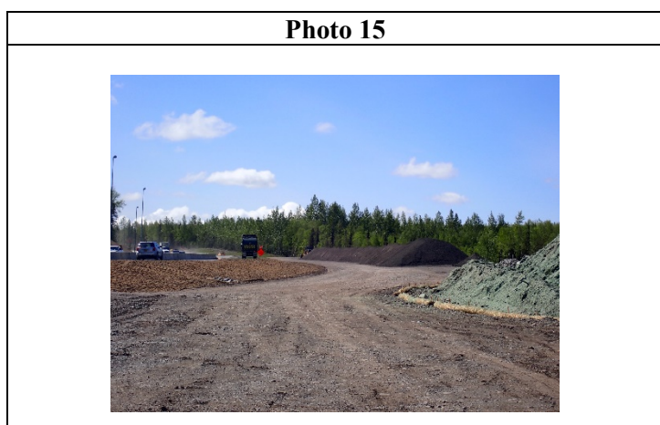
BMP Stockpile Stabilization Control – 15 of 20
