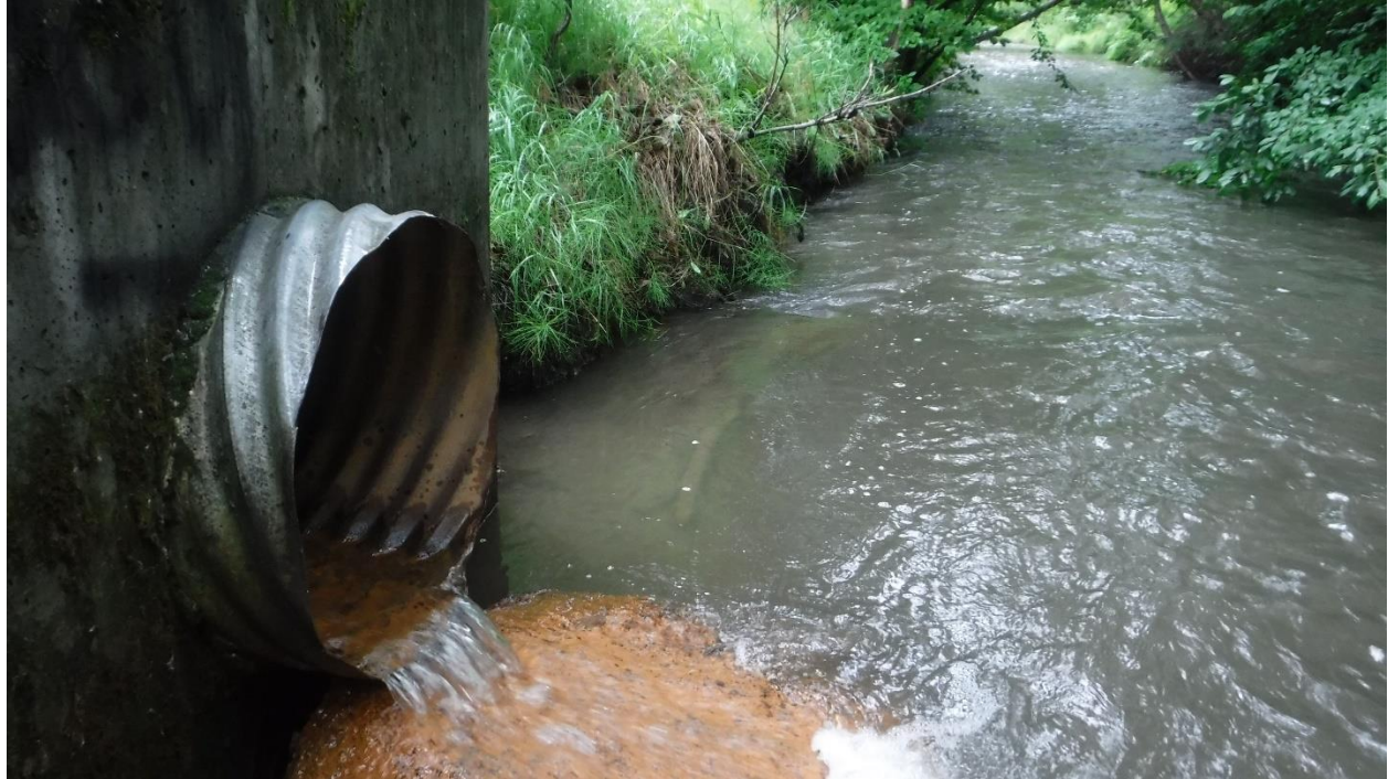
Photograph 10. Outfall SWM10 (525-2), Eagle Street at Chester Creek.
