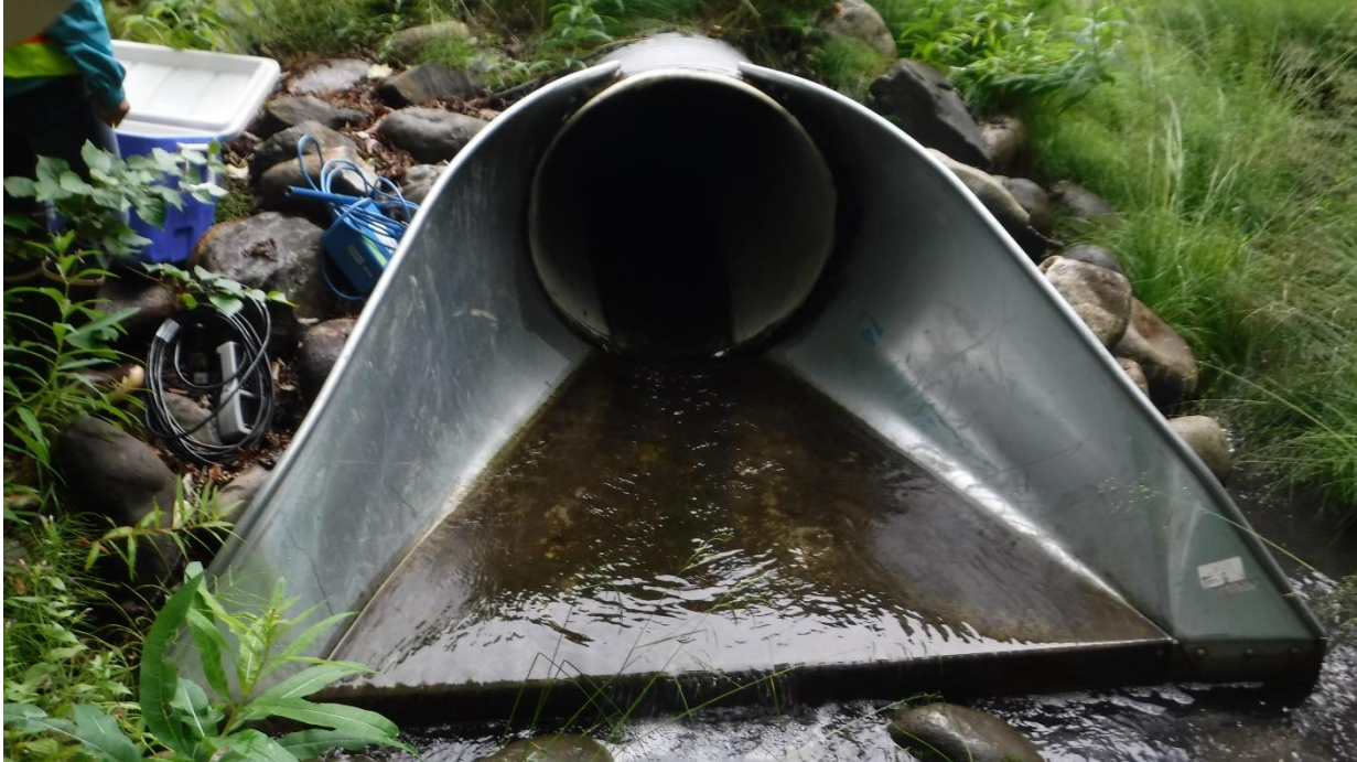
Photograph 3. Outfall SWM03 (1224-1), Fairweather Loop off Sylvan Drive.
