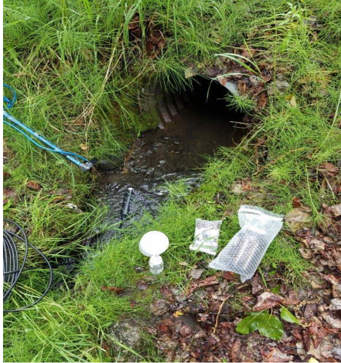
Photograph 9. Outfall SWM09 (499-1), Anchorage Football Stadium & Ben Boeke Ice Arena.
