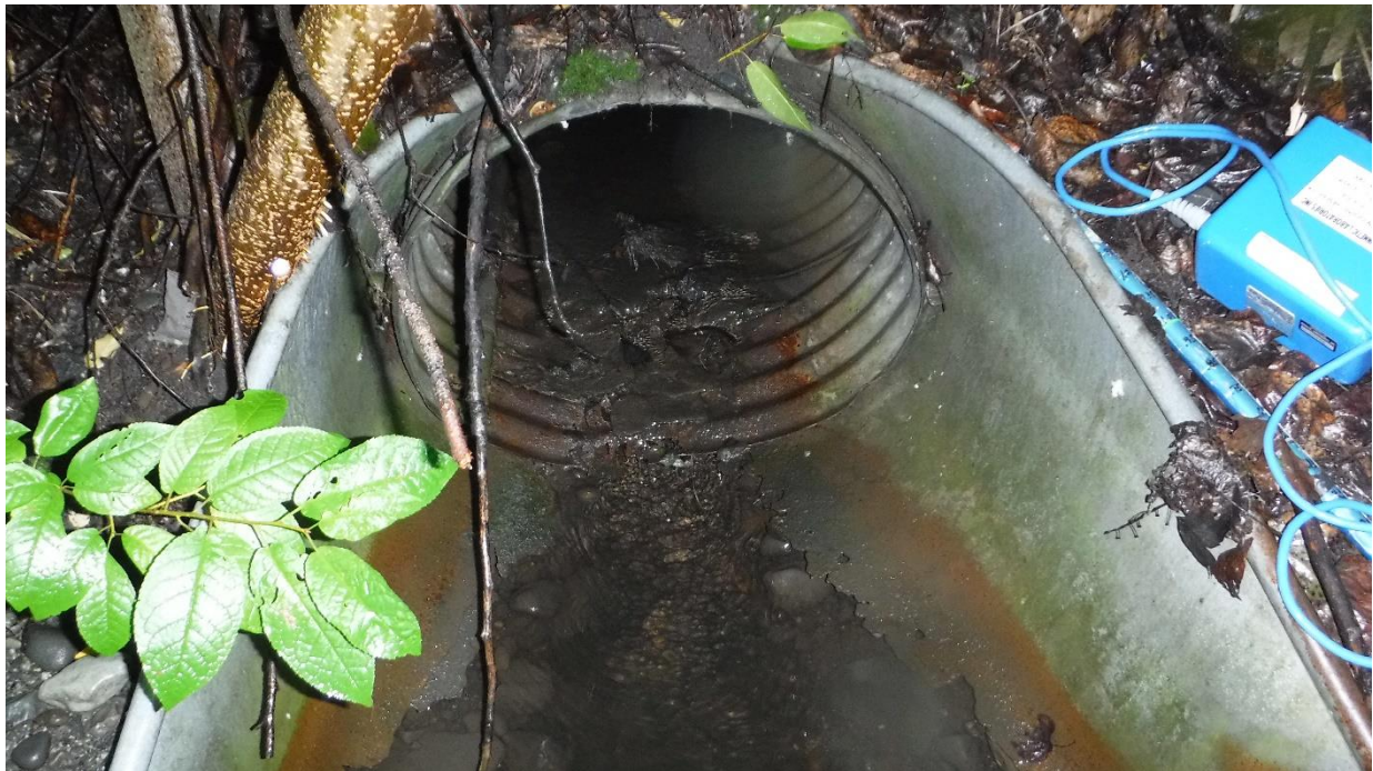
Photograph 6. Outfall SWM06 (314-22), Maplewood Street off of Northern Lights Boulevard.
