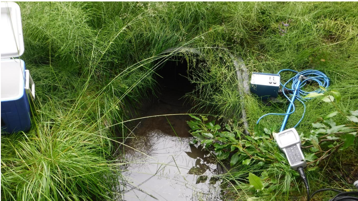
Photograph 4. Outfall SWM04 (1224-2), Fairweather Loop off Sylvan Drive.
