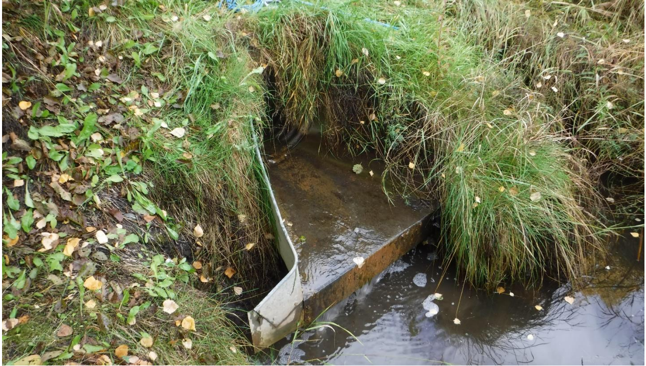
Photograph 5. Outfall SWM05 (207-1), East 56 th Avenue at Save School.
