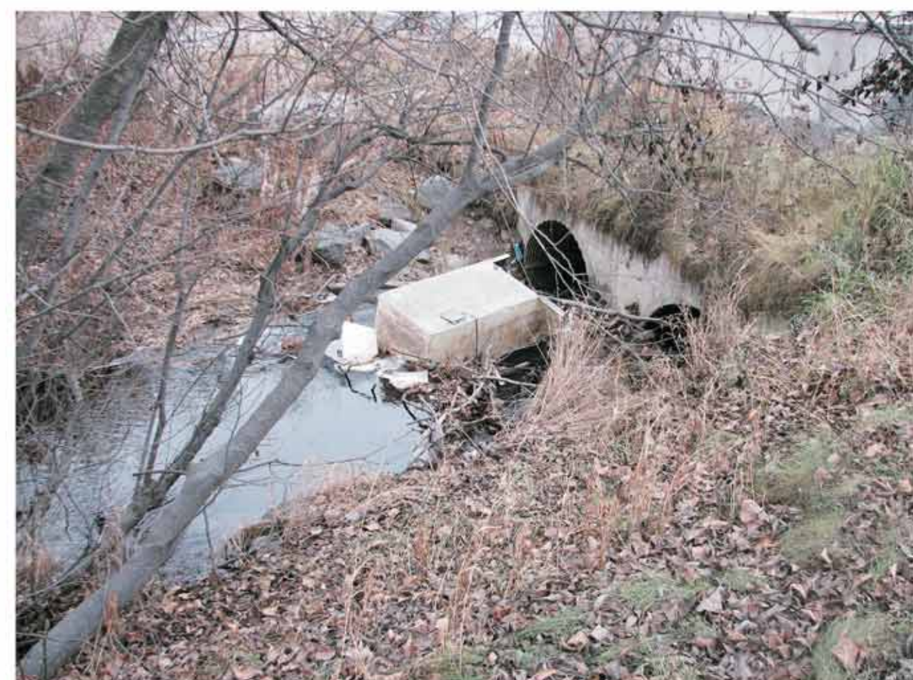
Original double culverts on S. Fork Chester Creek (east of Muldoon). Trash was typically found there which further compromised fish passage. (C. Northon, 2009)
