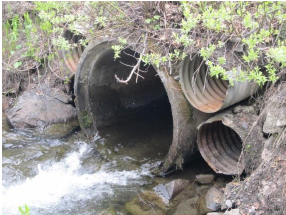
Figure 2 - Radio Tower culvert (ADF&G #20401888) Outflow (Photo by T. Eley 2017)
