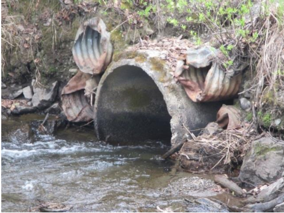
Figure 1 - Radio Tower culvert (ADF&G #20401888) Inflow (Photo by T. Eley 2017)
