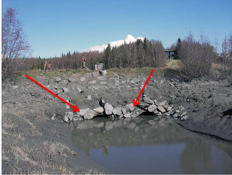
Figure 3 – Culverts (ADF&G 20401812) 750' west of the Campbell Lake spillway (Photo by ADF&G 6 , 2010)
