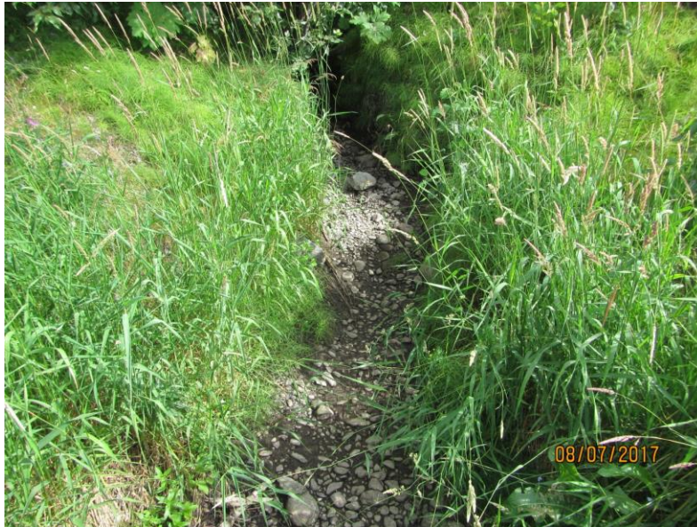
Figure 24. South Fork Little Campbell Creek adjacent to 8301 Petersburg Street showing the creek essentially dry. (Photo by T. Eley)
