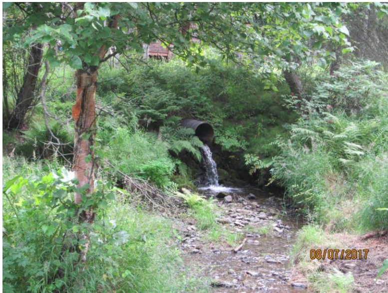
Figure 23. South Fork Little Campbell Creek as it exits the perched culvert east of Our Road and just before it enters the zoo. The flow is fairly normal for this time of the year. (Photo by T. Eley)
