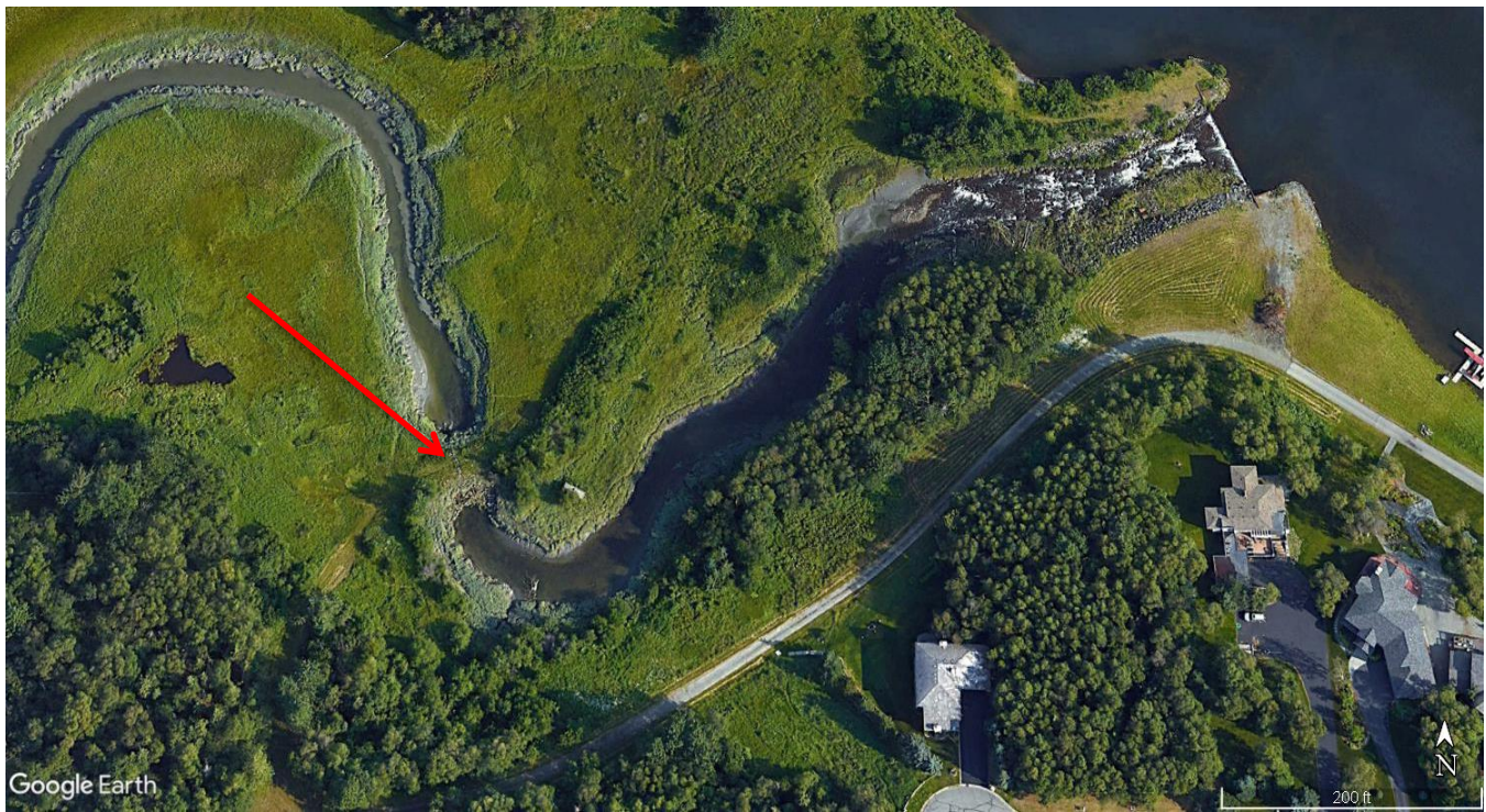
Figure 4 – Location of culverts by Campbell Lake (Image from GoogleEarth, 2014)
