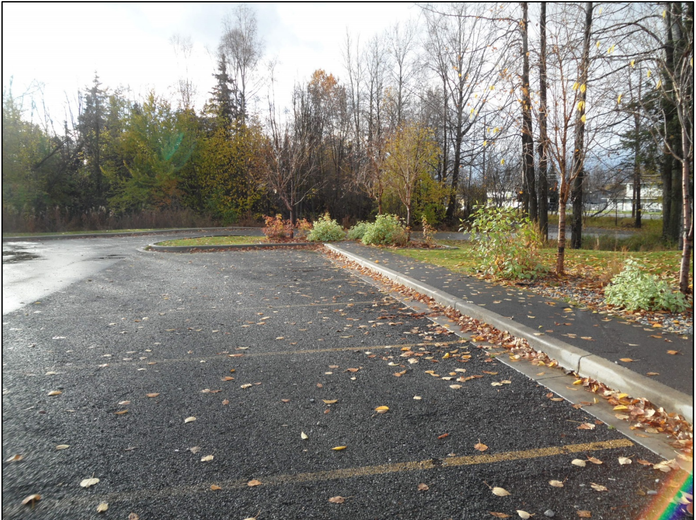
Figure 56: RJSP West Section of Porous Asphalt – October 16 Site Visit
