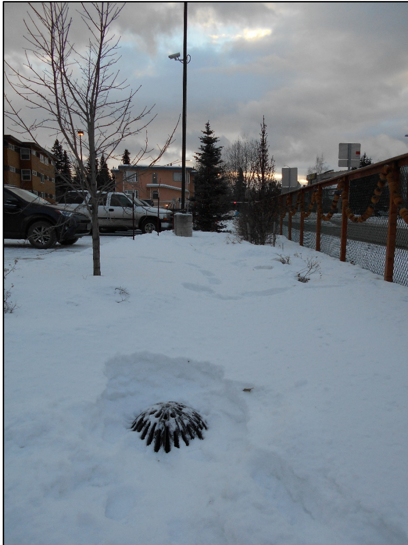
Figure 69: CFAB Rain Garden and Beehive Overflow – January 2019 Site Visit
