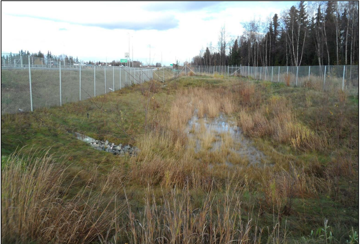
Figure 66: NSH Infiltration Basin – October 16 Site Visit
