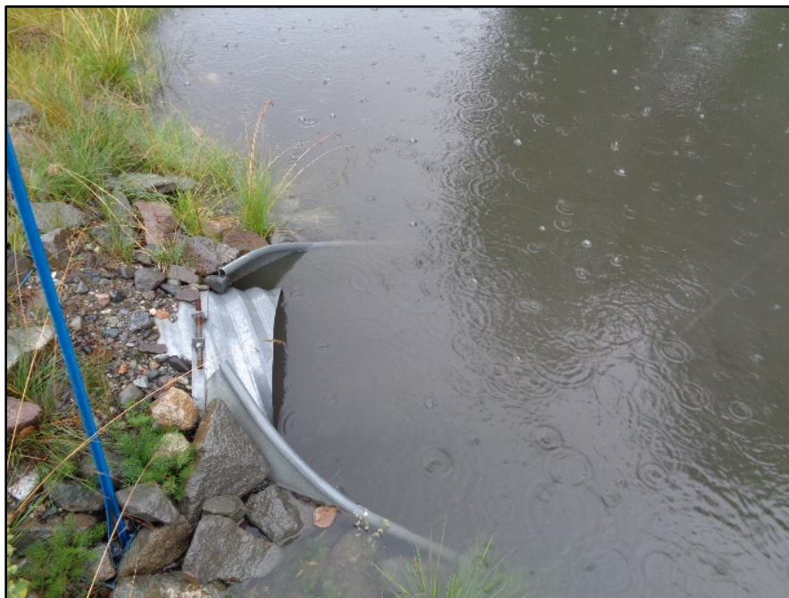
Figure 18: Infiltration Pond #1 Inlet, August 21, 2018
