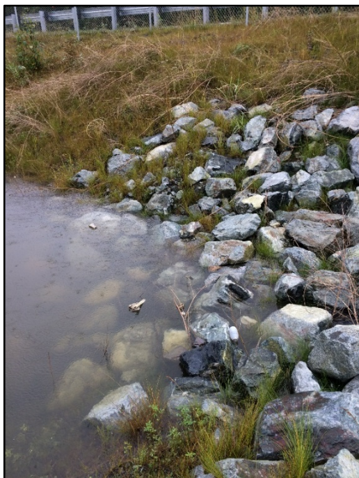
Figure 32: Outflow (left) and Submerged Inlet Culvert (right) – North Pond, August 21, 2018
