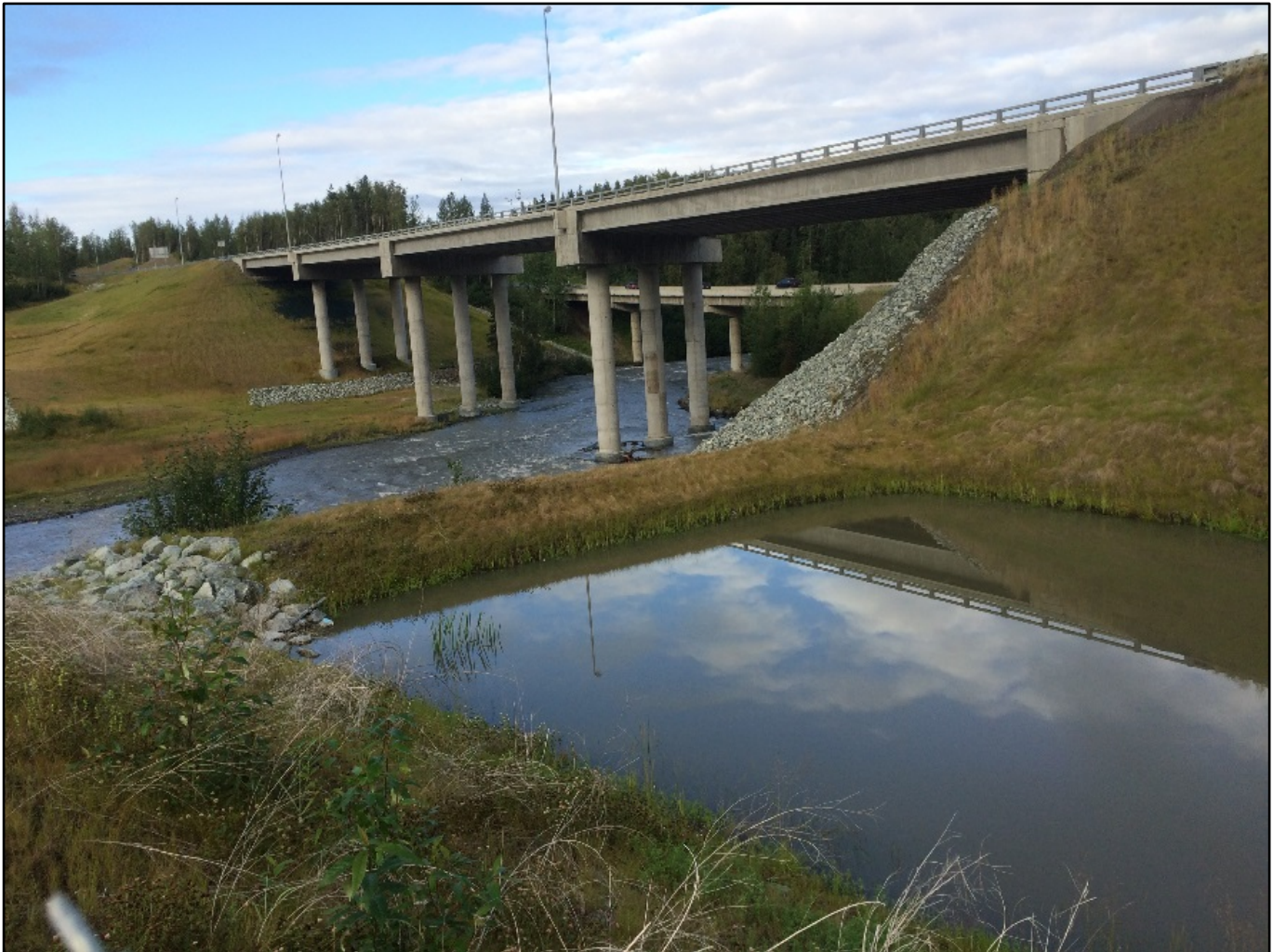
Figure 27: North Detention Pond Berm and Outfall
