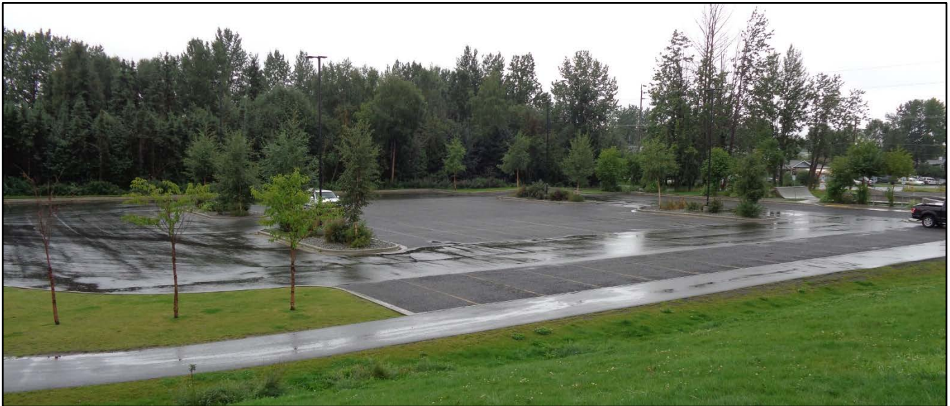
Figure 54: RJSP Parking Lot August 21 Site Visit
