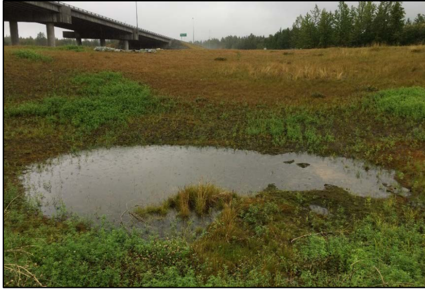
Figure 33: Standing Water in the South Detention Pond, August 21, 2018
