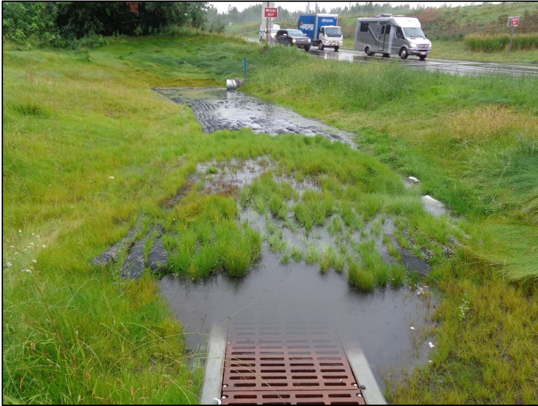
Figure 40: O'Malley Road Bioswale
