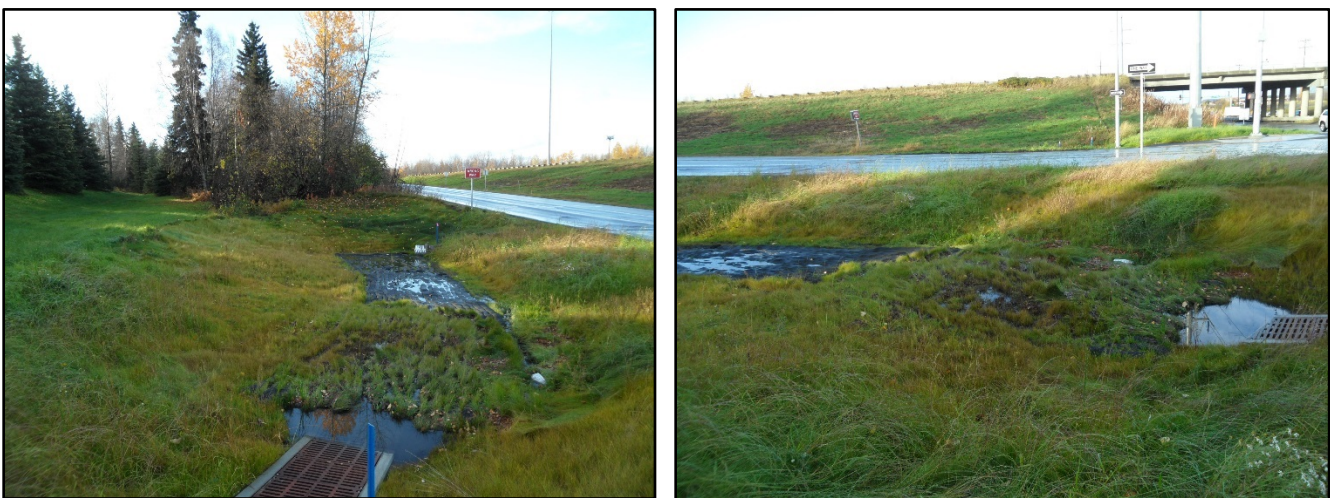
Figure 42: O'Malley Road Bioswale, October 16, 2018
