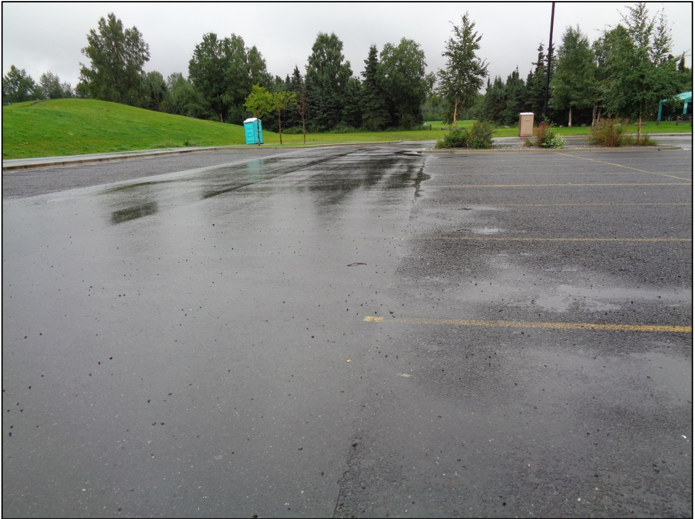
Figure 55: Porous/Traditional Asphalt Interface – August 21 Site Visit
