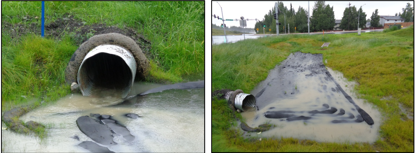
Figure 41: Bioswale Outlet and Bottom, August 21, 2018
