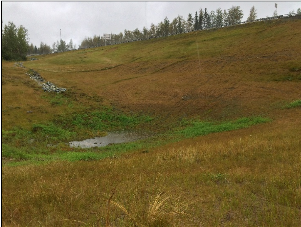
Figure 28: South Detention Pond Inlet Ditch (top) and Outfall (bottom)
