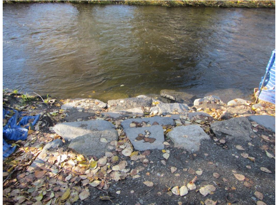
Creek Close-up of stone steps at Chester Creek along west bank (CW-4)
