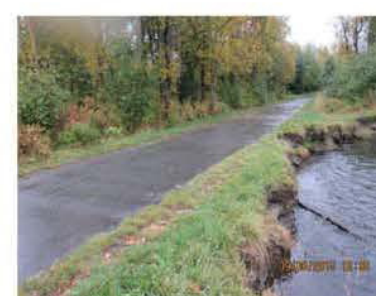
REALIGNMENT AND STREAM BANK IMPROVEMENTS
