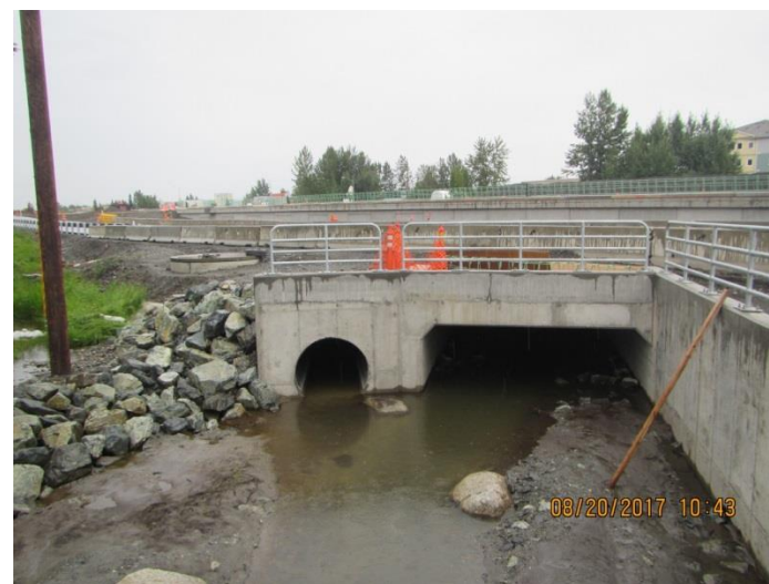
N. Fork Little Campbell Creek with new replacement culverts under the New Seward at 70 th and Homer looking east (August 2017)
