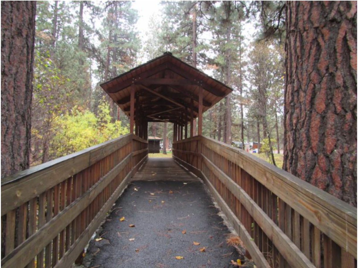
Covered foot bridge over Whychus Creek (photo by C. Northon)
