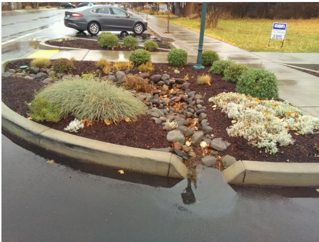
Stormwater runs through the curb cut into the bioswale, (photo by C. Northon).
