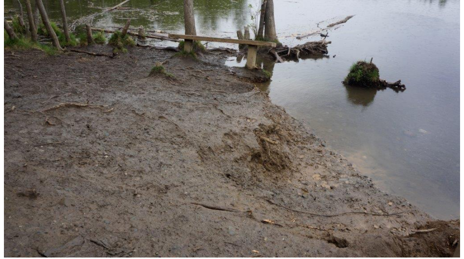
Bank erosion in 2016 near bridge across Chester Creek inflow
