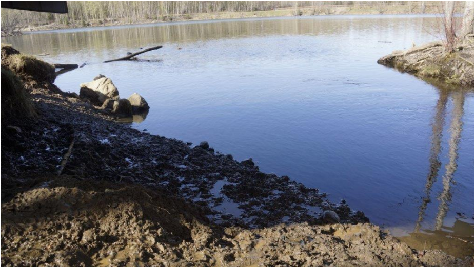
Bank erosion in 2016 near bridge across Chester Creek inflow
