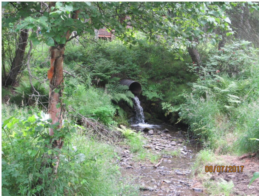
Photo 12. South Fork of Little Campbell Creek as it exits the perched culvert east of Our Road and just before it enters the zoo. The flow is fairly normal for this time of the year. (Photo by Thom Eley)
