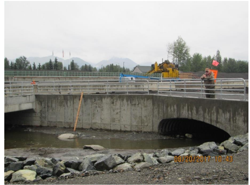
View of the flow of N. Fork Little Campbell Creek (looking southeast) running under the new driveway (August 2017)
