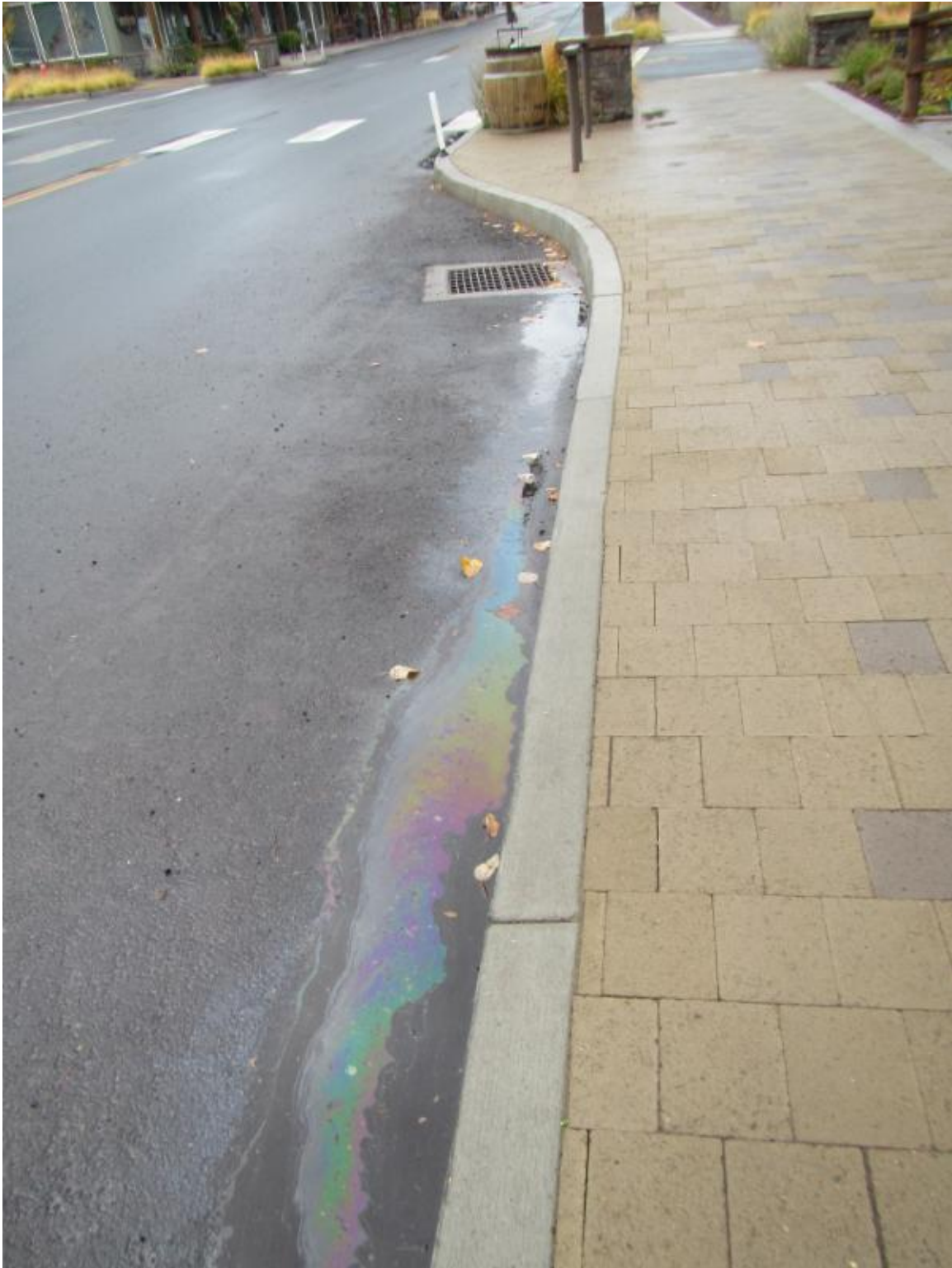
Oil sheen in stormwater heading to a stormdrain, Cascade St., (photo by C. Northon)
