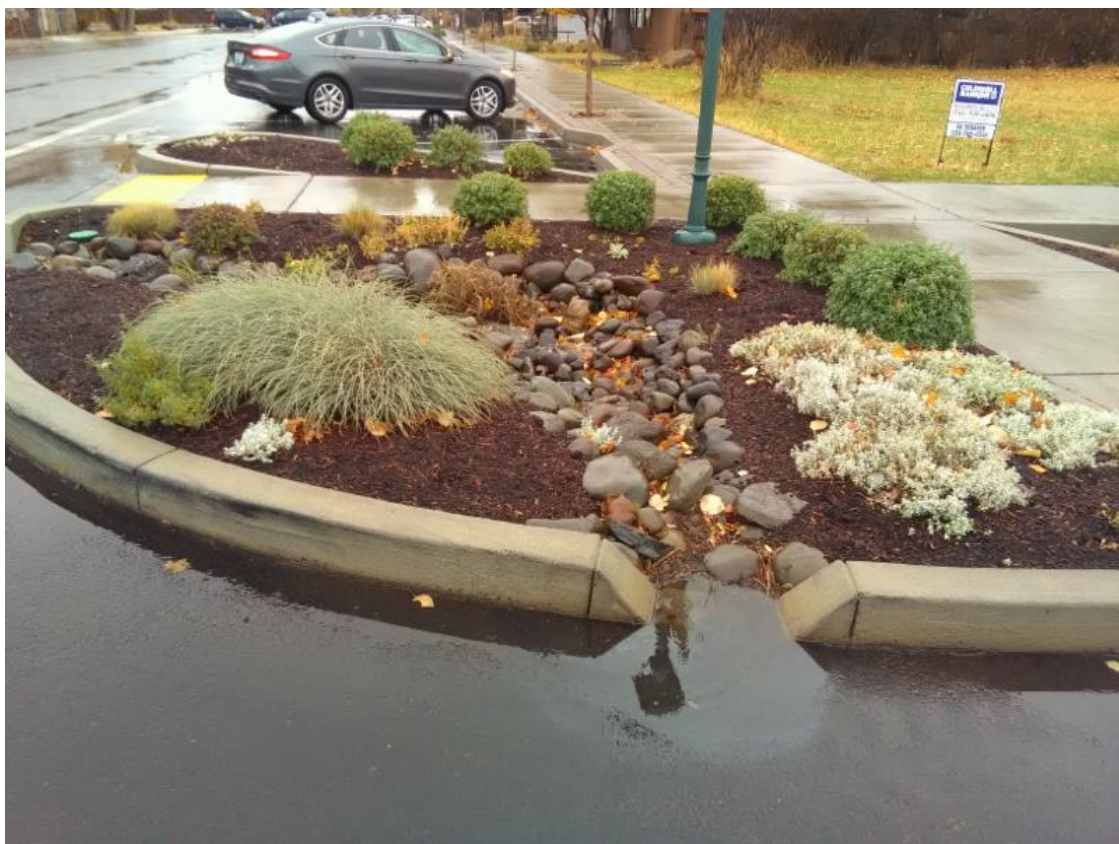
Stormwater runs through the curb cut into the bioswale, (photo by C. Northon).
