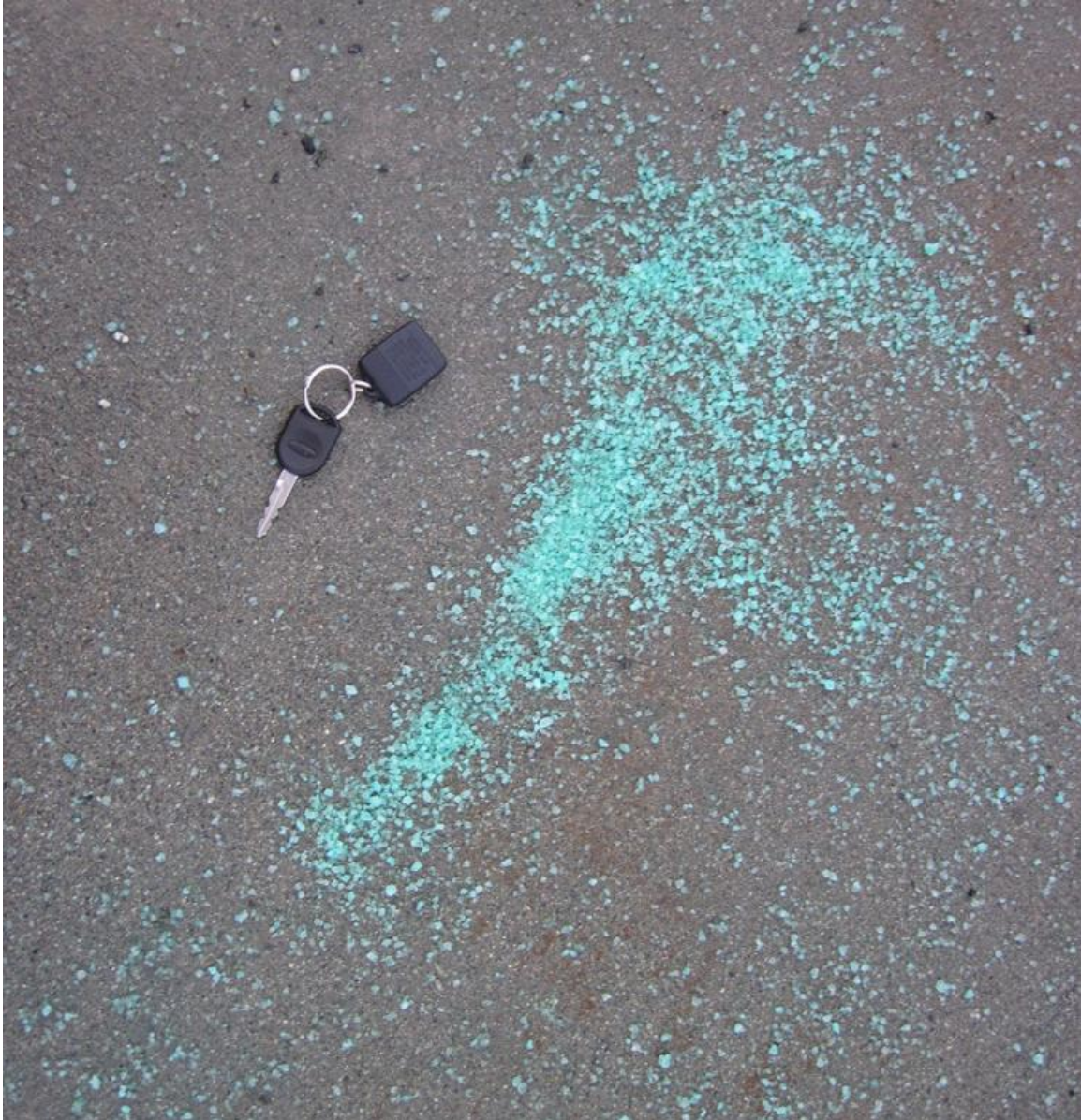
Ice/snow melt applied unevenly
