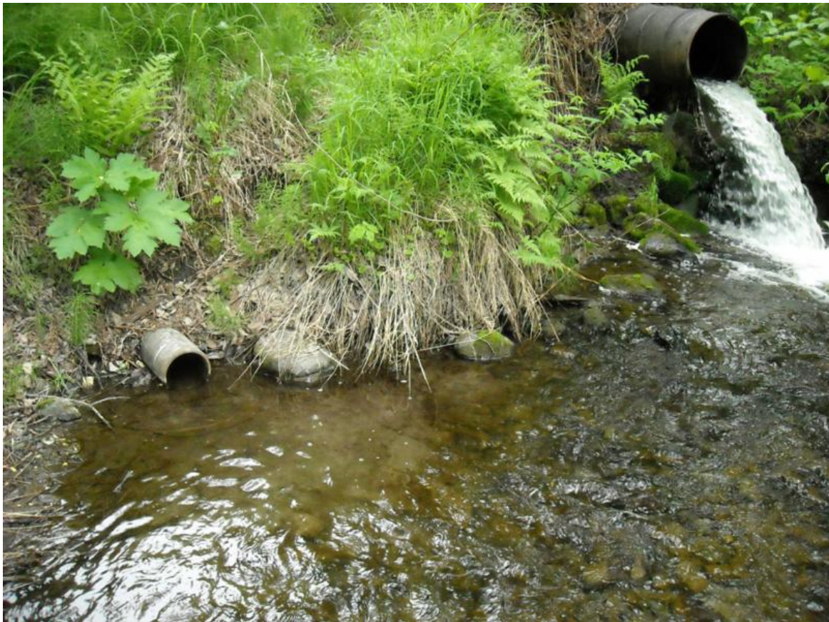
Stormwater sewer outfall from storm drains flows into Little Campbell Creek
