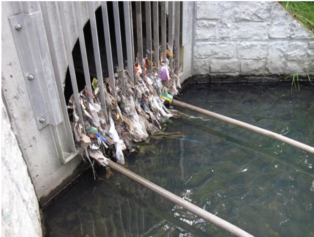
Stormwater outfall from C St. into Chester Creek—some trash is captured by a grate.
