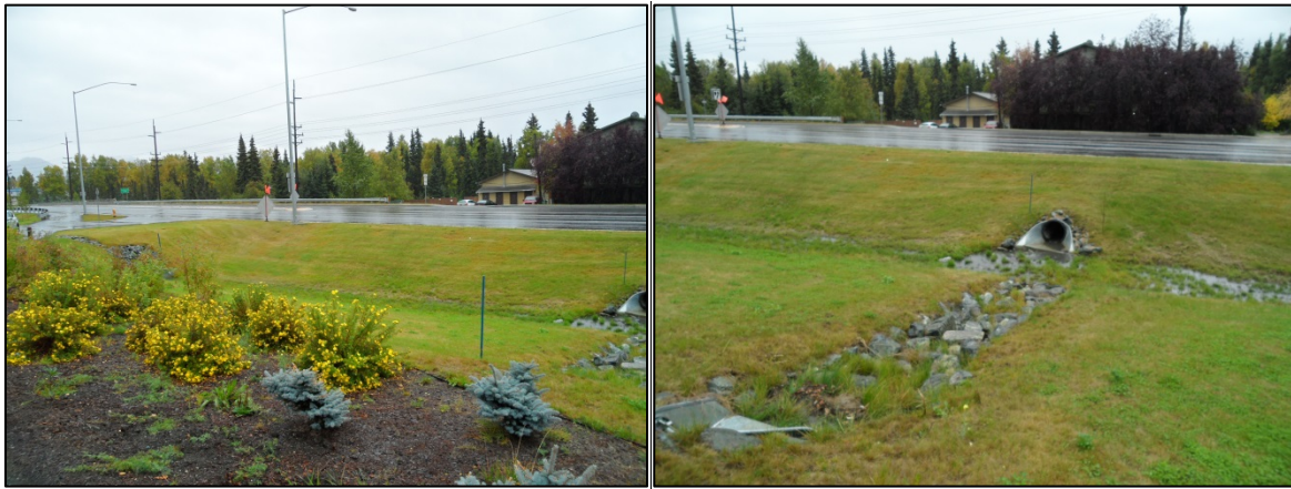
Overview and storm drain outfall to bioswale.
