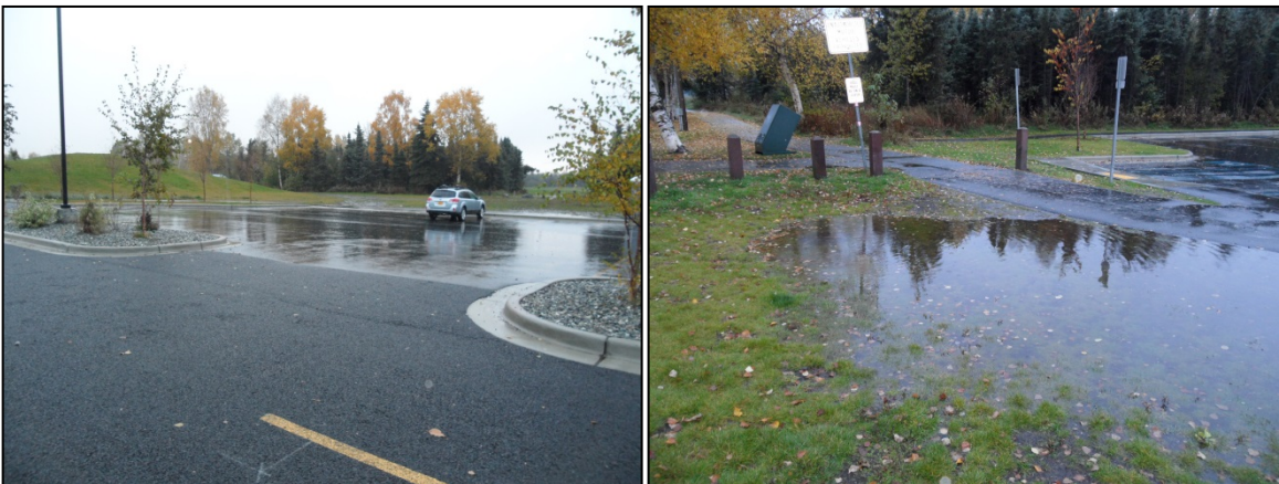
Left: East asphalt interface. Right: Ponding east of the parking lot.
