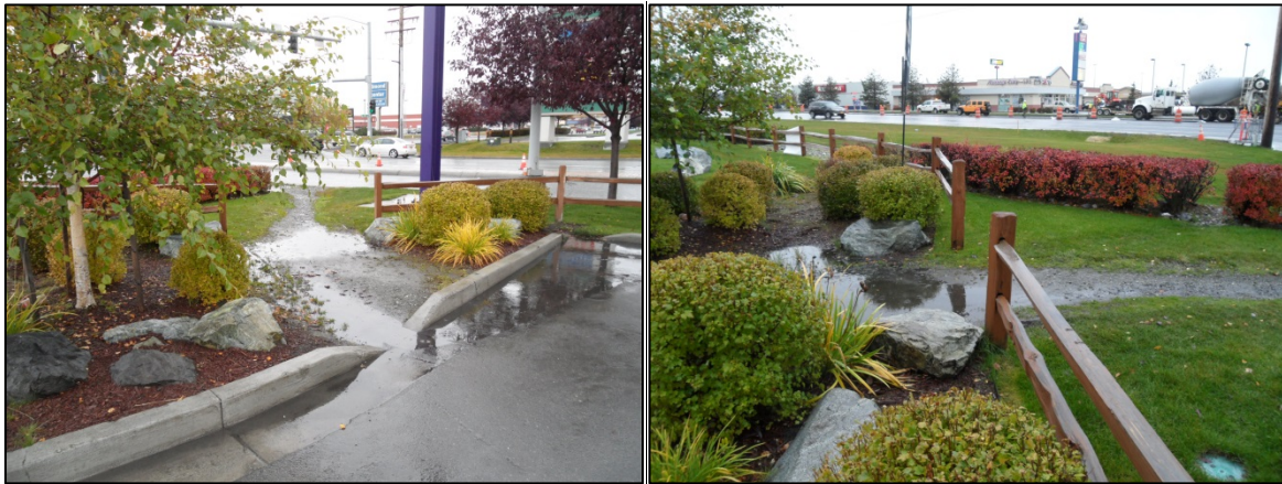
Taco Bell Parking Lot – North Side. Foot path not overflowing.
