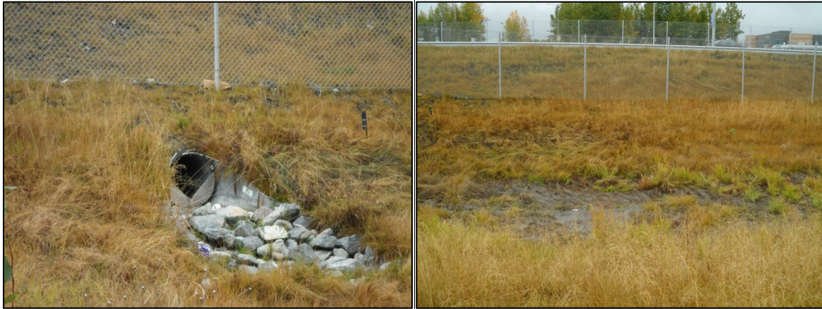
Left: Inlet Right: Ponding in the facility
