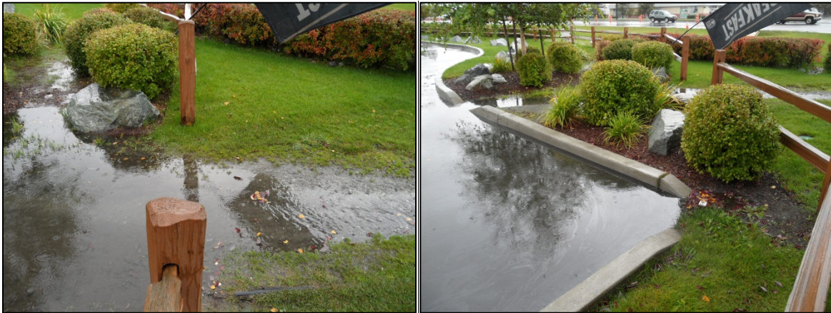
Left and Right: Water bypassing vegetation via footpath.
