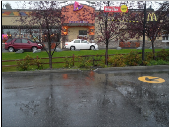
Left and Right: Water entering the vegetation from the parking lot via curb cuts.
