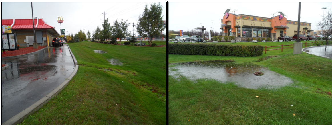
Left: Vegetated Swale. Right: overflow beehive. (It was not clear why the beehive isn't flowing. Another storm drain manhole with a top grate is located near this beehive.)
