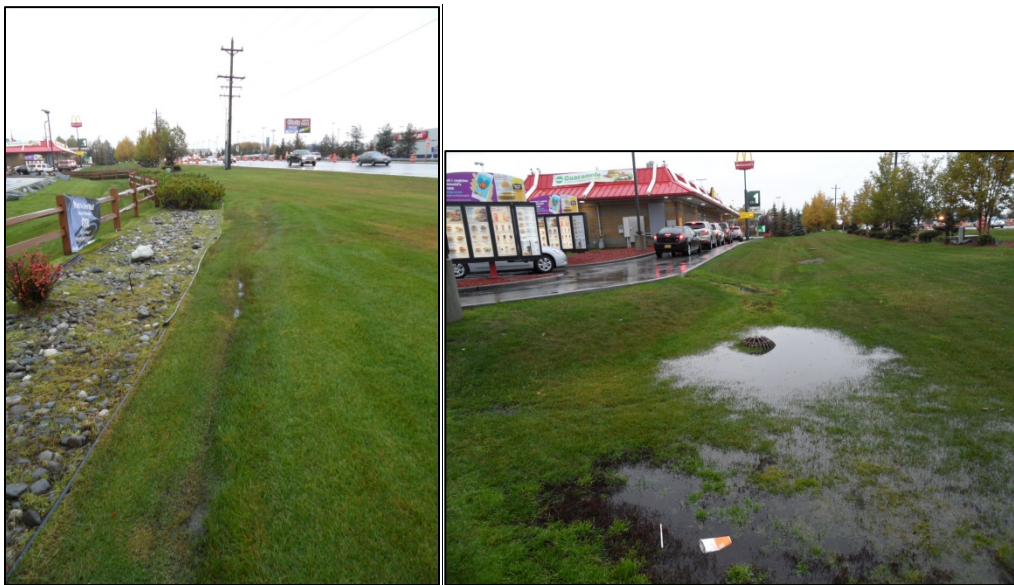
Left: Vegetated Swale, standing water visible. Right: overflow beehive that is not flowing.
