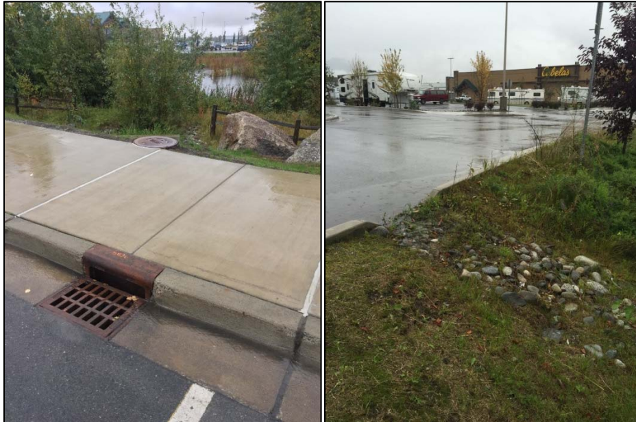
Figure 43: Inlets to Target Stormwater Pond
