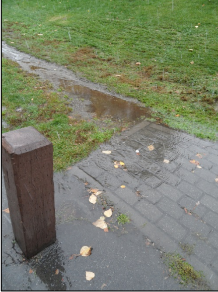
Left: Significant concentrated flow running toward the rain garden. Right: Outlet flow
