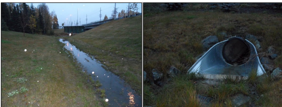
Left: Bioswale flow path to Campbell Creek. Right: Muddy water inflow.
