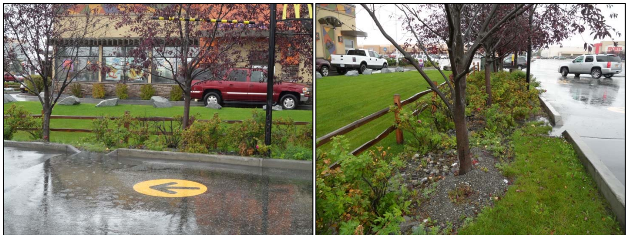
Figure 34: Curb Cuts Draining to Landscaping
