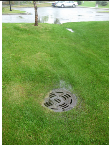
6 Close-up of field inlet area
