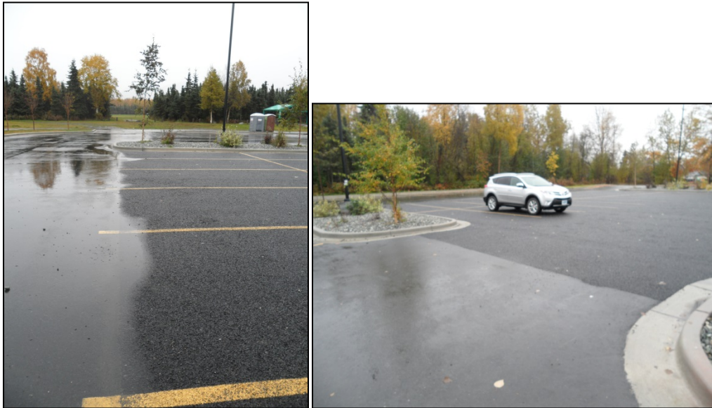
Left: North asphalt interface. Right: West asphalt interface
