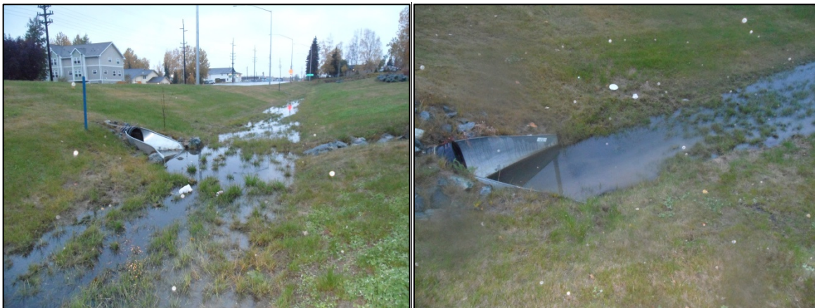
Left: Overview of bioswale. Right: Bioswale outlet.
