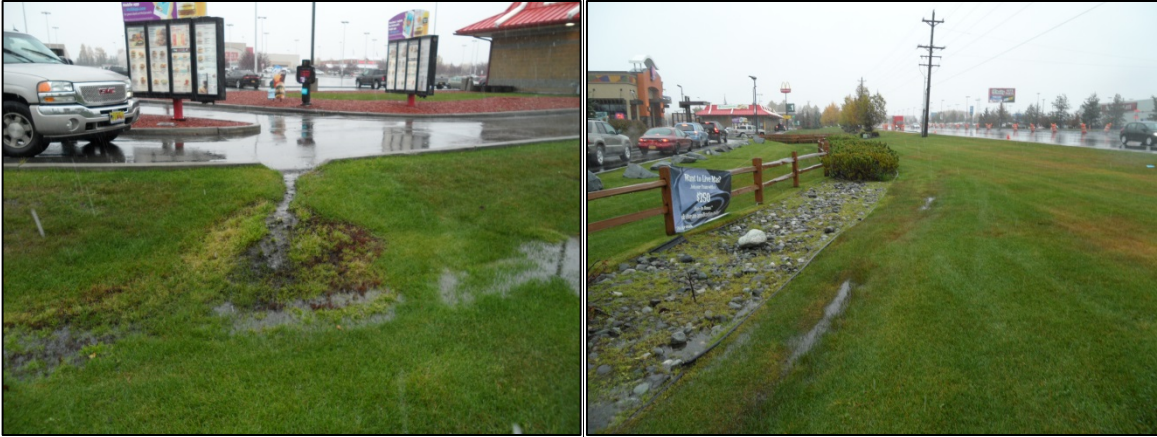
Left: Flow from the parking lot to the vegetated swale via curb cuts. Right: water ponded in the vegetated swale.
