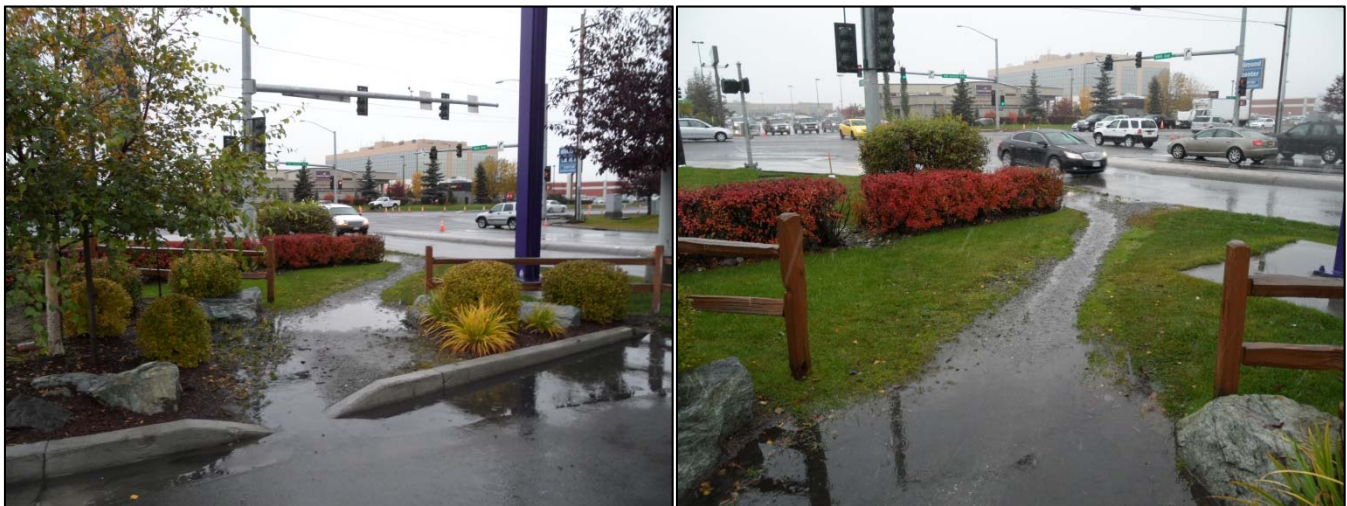
Figure 39: Pedestrian Pathway Drainage
