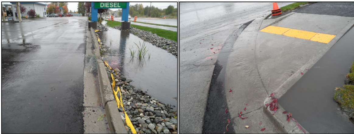
Above left: Water flowing into the facility via a curb cut. Above right: Overflow at the downstream end (north) Left: Facility Overview. Below: Parking lot
