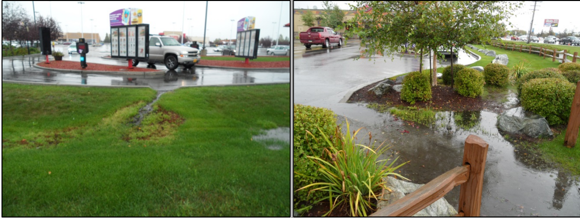
Left: Water entering swale from drive-through. Right: Water entering vegetation from parking lot.
