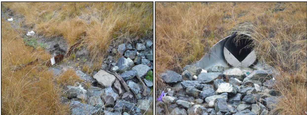
Figure 14: Infiltration Basin Outlet (left) and Inlet (right)
