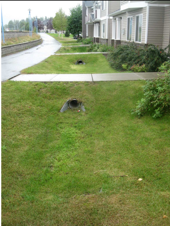
3 East portion of north east-west swale < some standing water in second cell from front >
