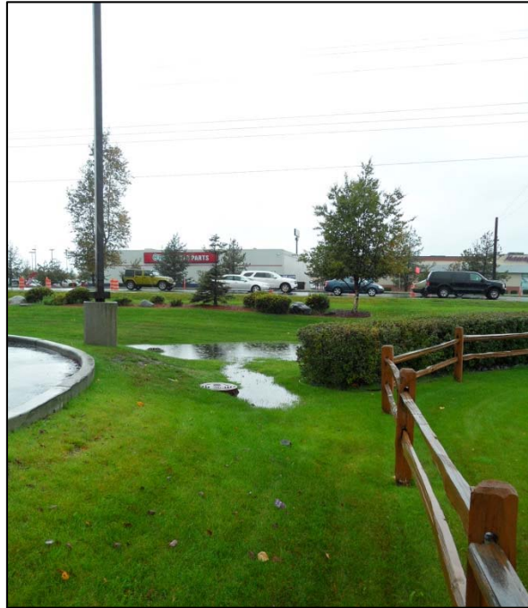
Figure 37: Elevated Storm Drain Inlet
