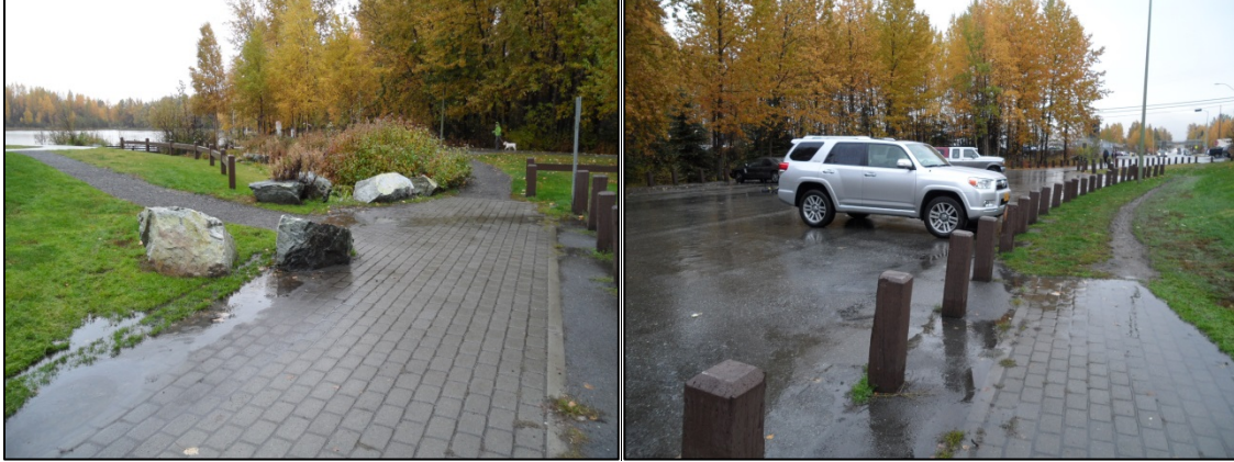
Left and right: Water flow toward the rain garden inlet.
