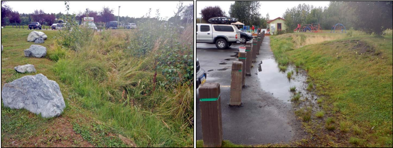
Figure 40: Westchester Lagoon Rain Garden and Parking Lot
