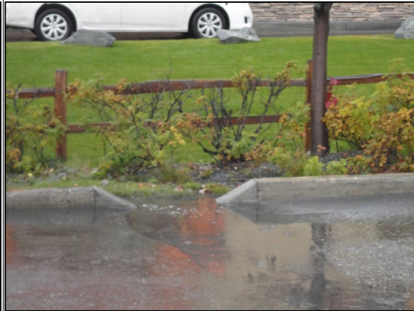
Left and Right: Water entering the vegetation from the parking lot via curb cuts.
