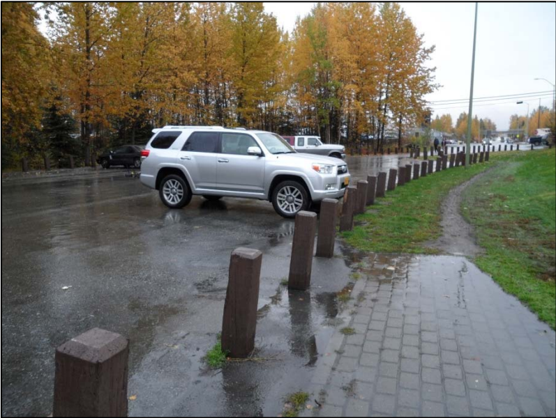
Figure 26: Concentrated Flow from the Parking Lot 9/28/15
