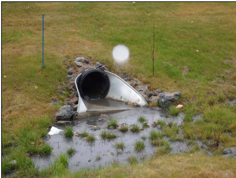
Figure 7: Outfall Discharging to Bioswale
