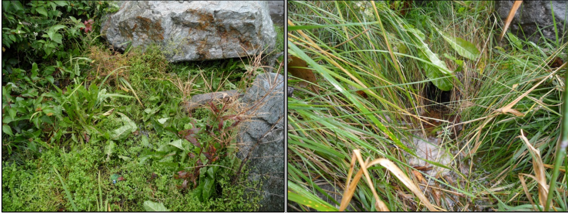
Left: Vegetation inside the rain garden. Right: Underdrain outfall
