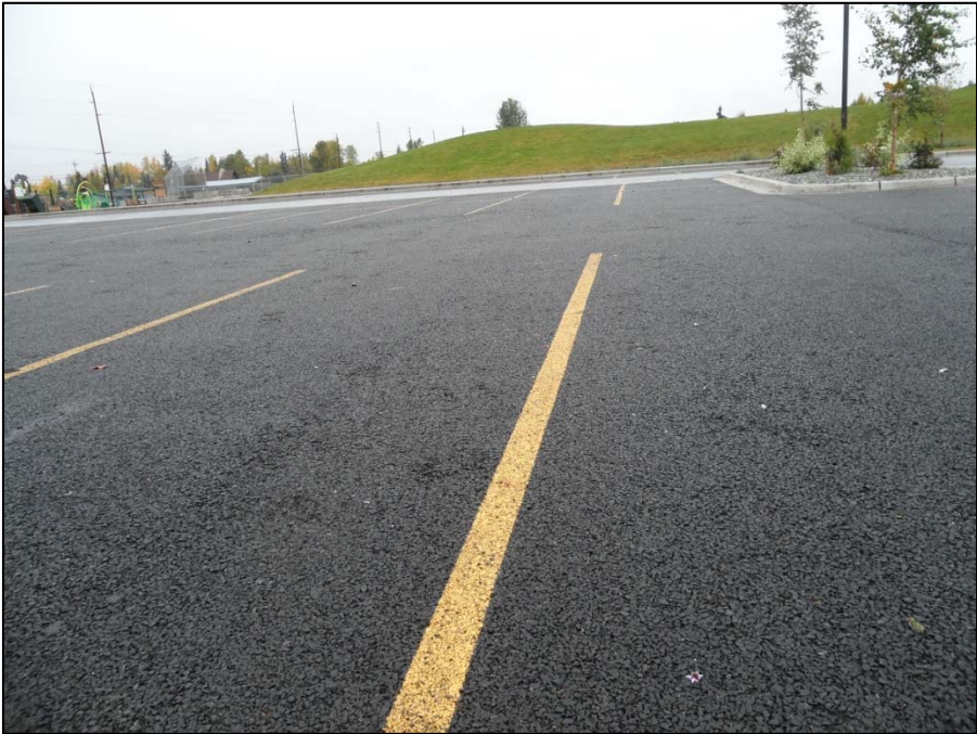
Figure 22: Loose Rocks Collecting on the Asphalt
