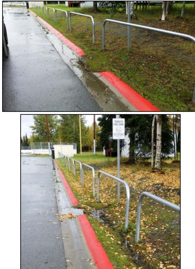
Figure 49: Rogers Park Elementary Debris Blockage Before (Top) and After (Bottom)
