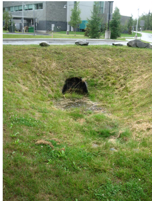
Outlet from Area #1
