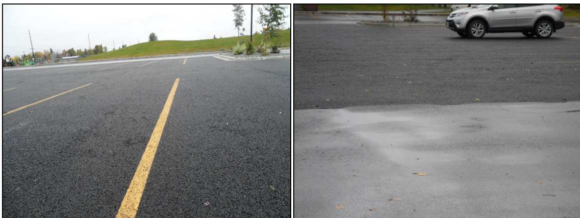
Left: Surface raveling. Right: Interface heaving
