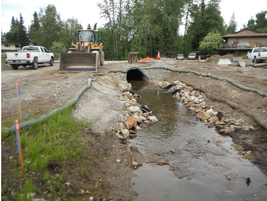
Fish Creek 1310-201 : New construction and new outfalls
