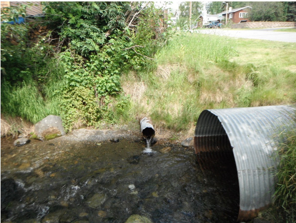
Eagle River 1375-99 : North bank; Chain of Rock Street and Teklanika Drive
