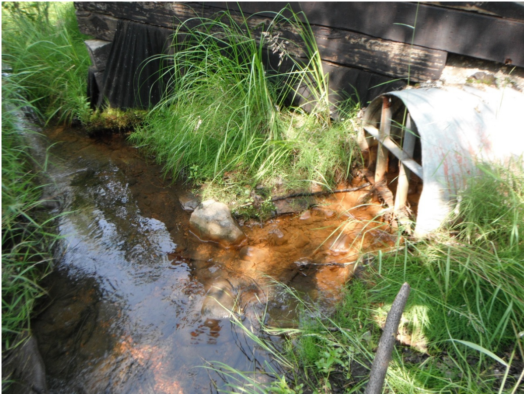
Campbell Creek 1056-117 : Southwest corner of Carriage Drive.
