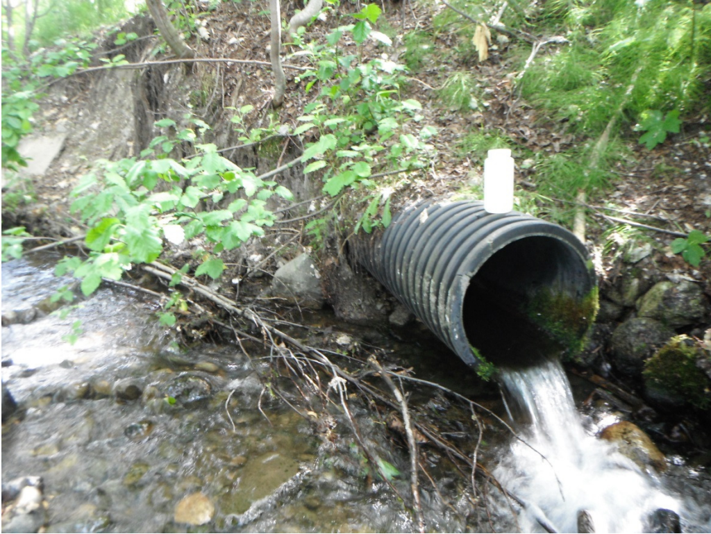
Eagle River 646-71 : South bank; Chain of Rock Street and Teklanika Drive.
