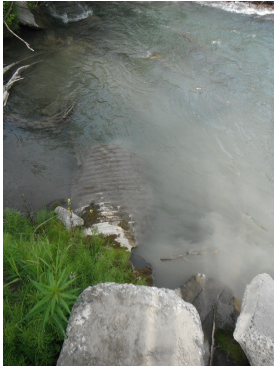
Ship Creek 189-1 : Submerged outfall
