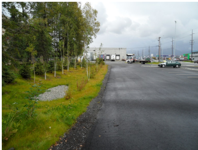
Figure 22: West Dowling Rain Garden and Parking Lot
