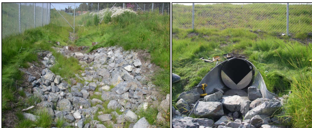
Figure 7: Retention Basin Outlet (left) and Inlet (right)
