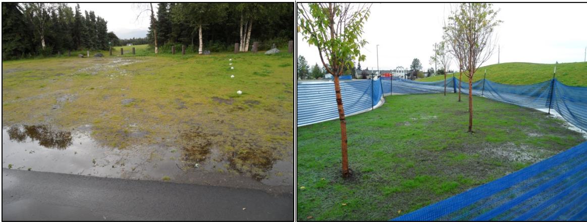
Left: Runoff from the area to the east of the parking lot. Right: Seeded area that replaced the mulch.
