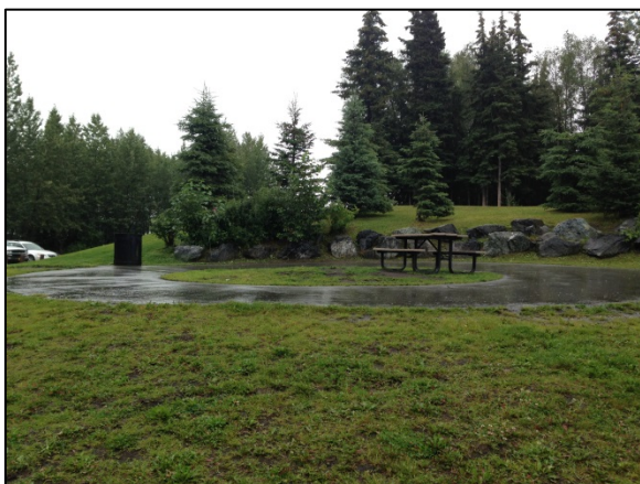
Runoff from adjacent walkway
