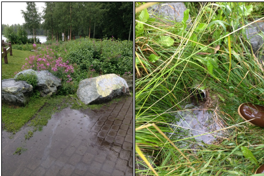
Water entering rain garden (Left) and rain garden outlet pipe (right)
