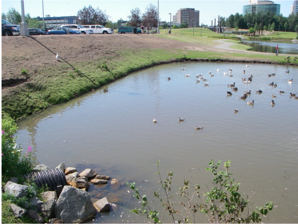
Fish Creek Cuddy Park 1287-1858-1 Inlet to pond at Cuddy Park. Not currently mapped as being connected to the MS4 network. Node code assigned based on location in the network.
