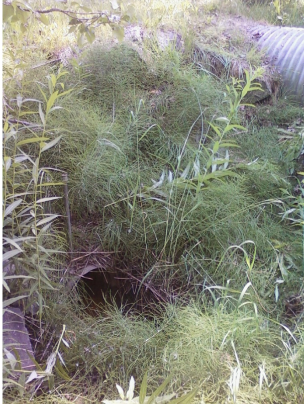
Fish Creek (1287-994) Small culvert in Hermit Park on Willow Street
