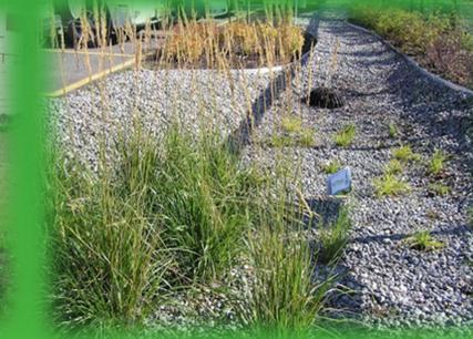
Left: This commercial bioretention area is collecting runoff from a parking lot of a local business. The area is designed with an overflow inlet for large rainfall events.
