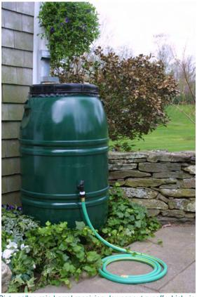
Sixty gallon rain barrel receiving downspout runoff which, in turn, provides water that can be directed onto vegetation.
