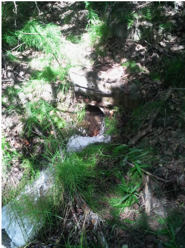
CHS 700-10 Outfall and drainage
