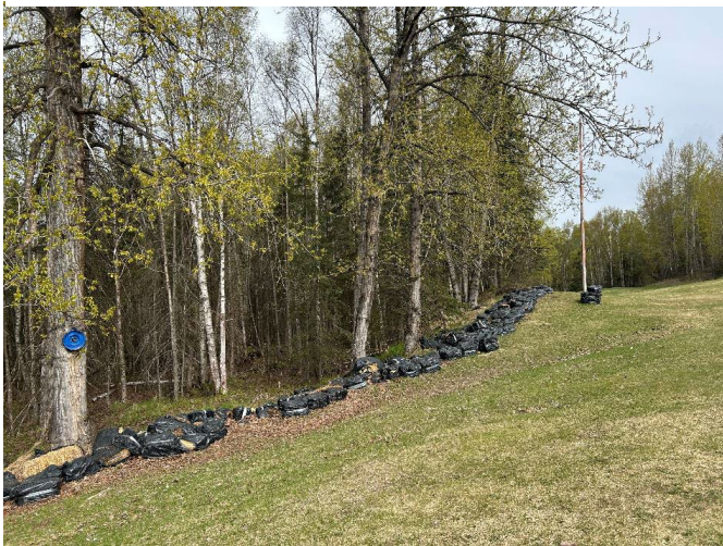
Above: Sledding hill runout zone with temporary safety intervention.
