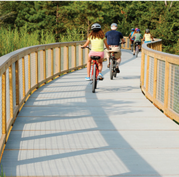
Figure 4.2 : Example of pedestrian bridge with wooden and composite elements from Cape Henlopen State Park. Image credit: Strongwell
