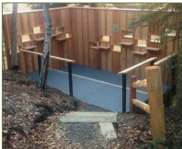
Sandhill Blind at terminus of Forest Trail: Inadequate yellow safety strip (may need to be done next spring now); trim piece between 5 th & 6 th window on south wall, loose and sitting in corner (needs to be screwed to wall); need warning sign on last post before deck about split level platform. Barbara Carlson, FAR, October 2013.
