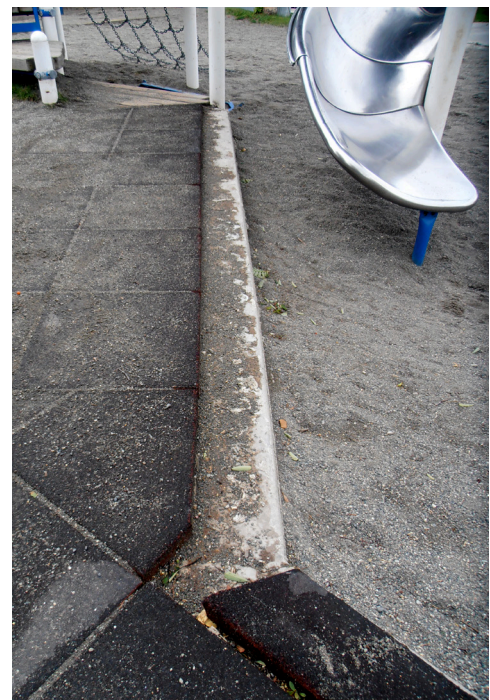
Figure 14 Dated fall surfacing and overflowing pea gravel
