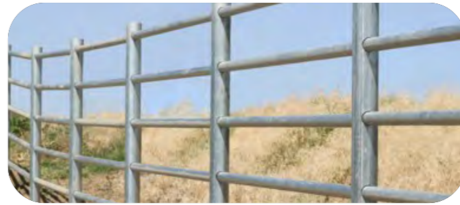
Safety Fencing Galvanized steel post and rail fencing system along trail.
