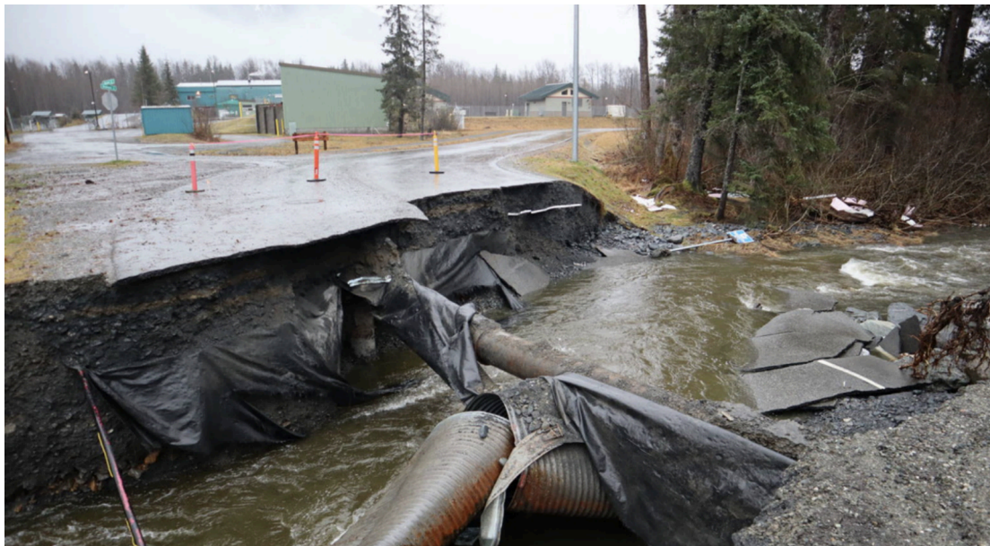
(P2) October 2021, Ruane Road culvert washout exposing sewer main after rain event
