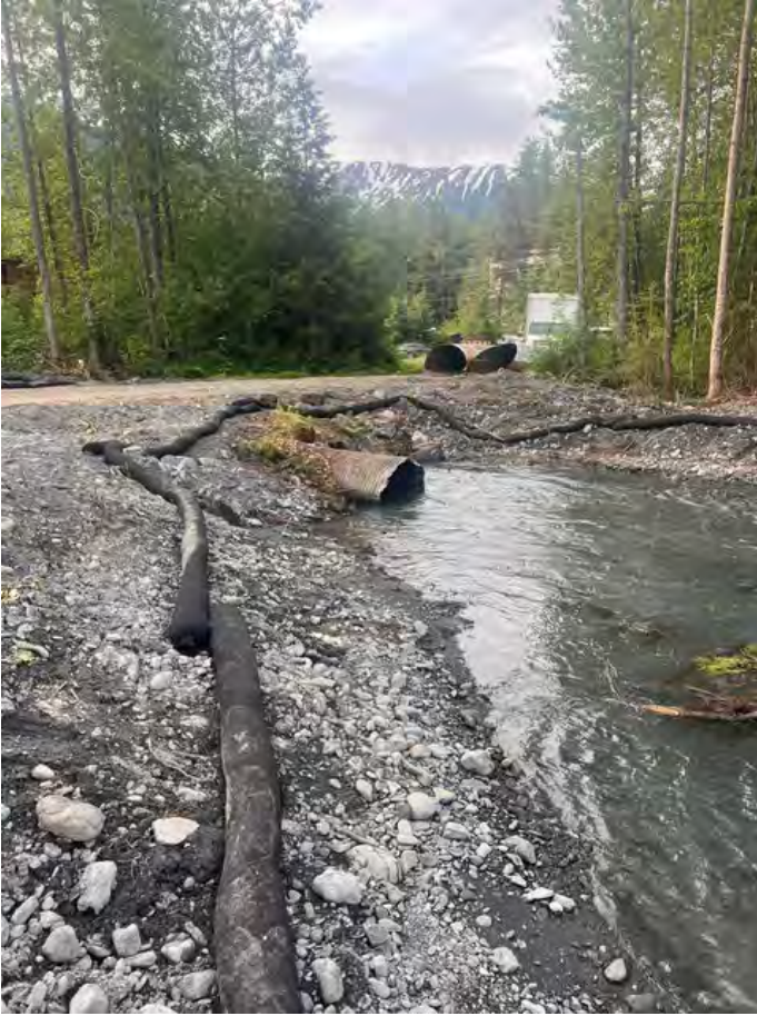
Alyeska Creek at Davos new Fish Passage project: Original culverts
