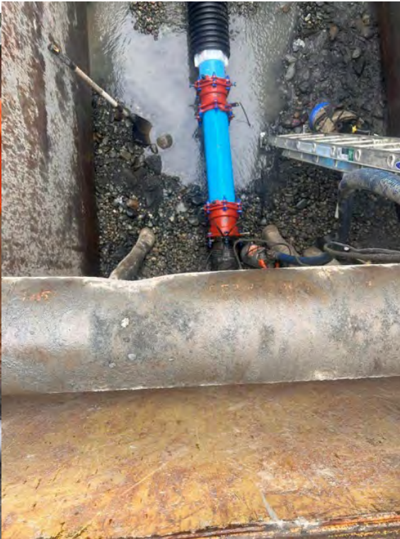
Lowering the water line for the new culvert installation
