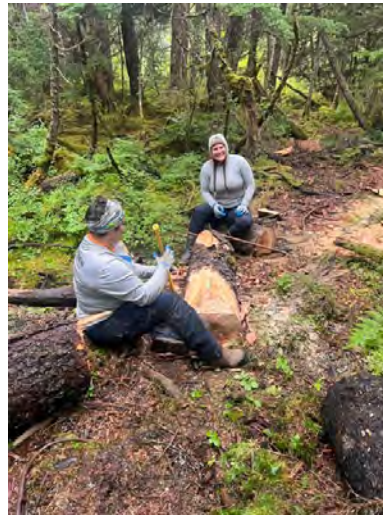
Alaska Trails Crew peeling logs for turnpike
