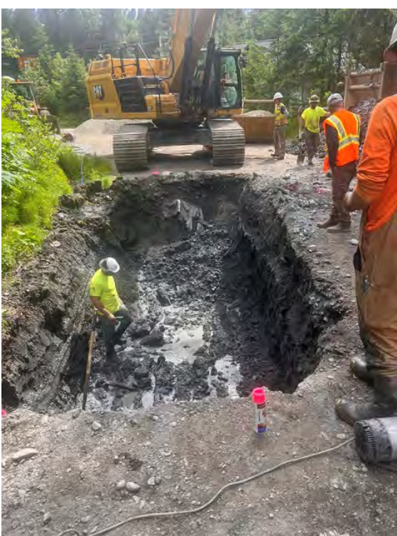
Lowering the water line for the new culvert installation
