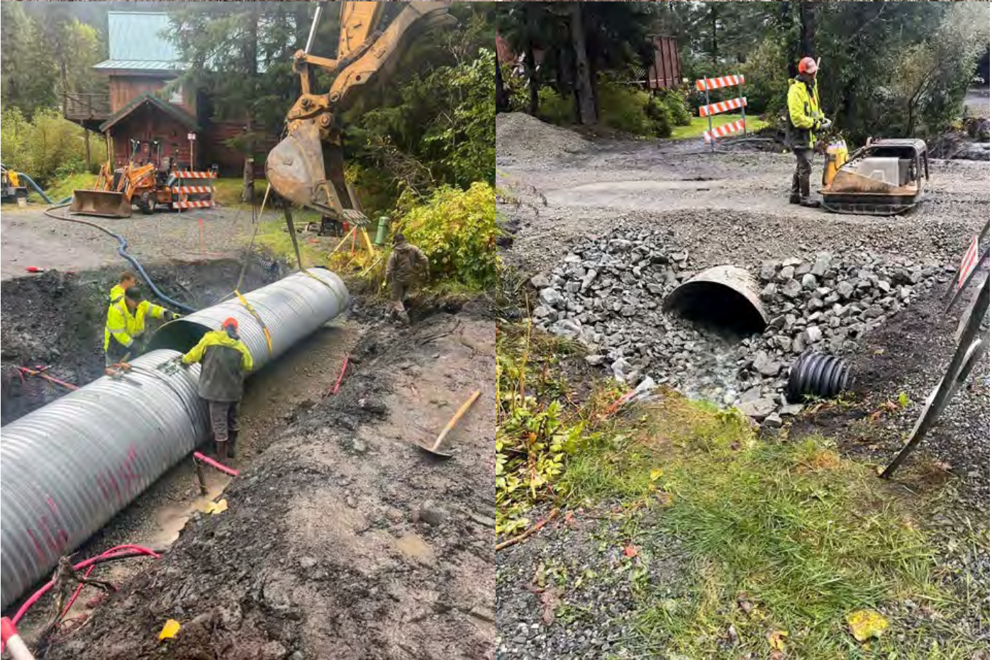
Installing new culvert around all the utilities and working on final product
