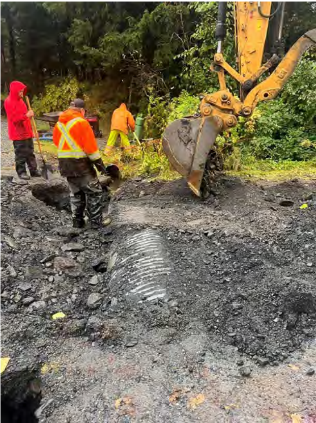
Removing old culvert
