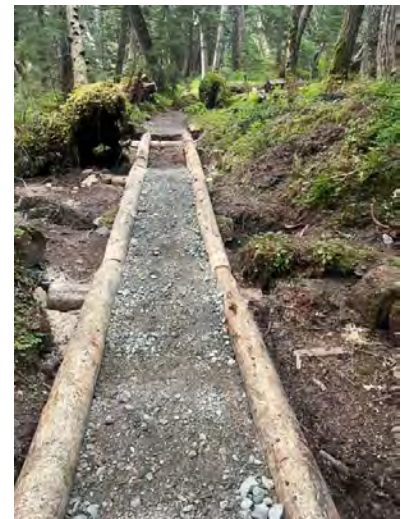
Lots of drainage work, turnpike and gravel by Alaska Trails
