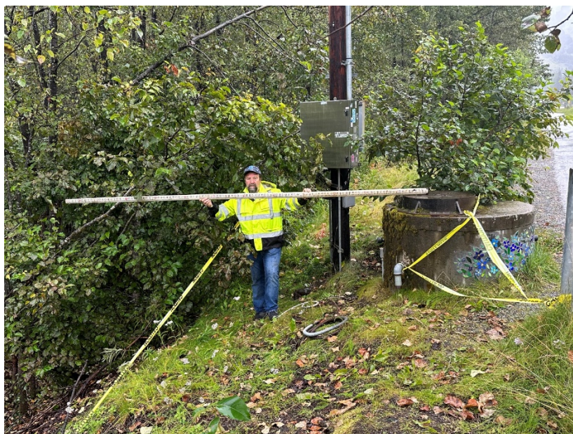
Picture 2 – Proximity of Air Vacuum Vault to Slope Failure
