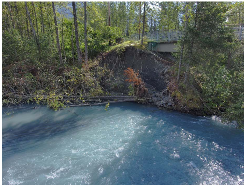
Picture 1 – Slope Failure at Glacier Creek
