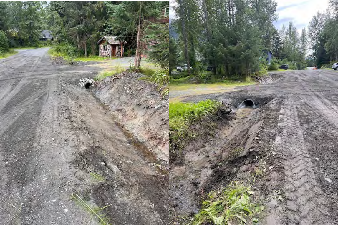
Arlberg Ditch cleaning and reshaping
