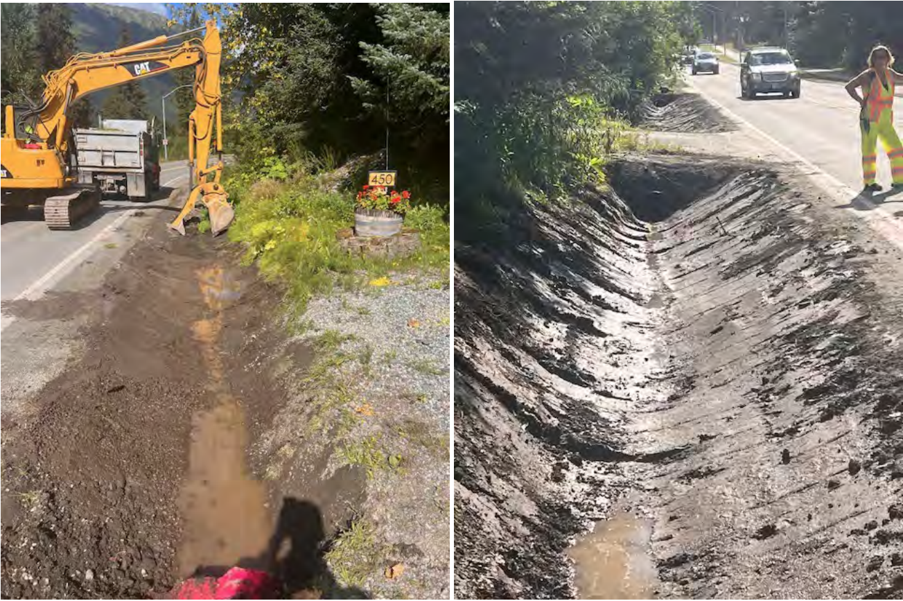
Arlberg Ditch cleaning and reshaping
