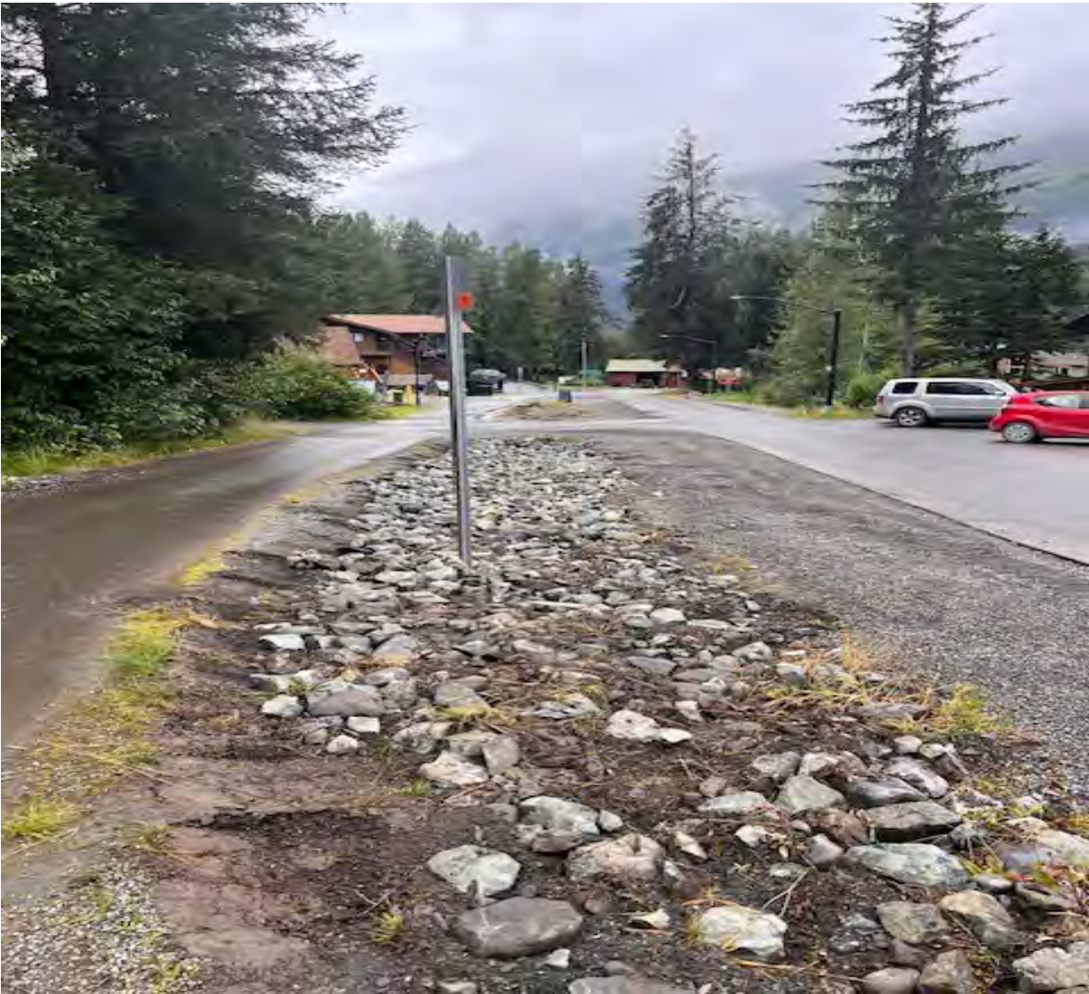
Olympic Mountain Loop Ditch vegetation removal and reshaping of Rip Rap rock
