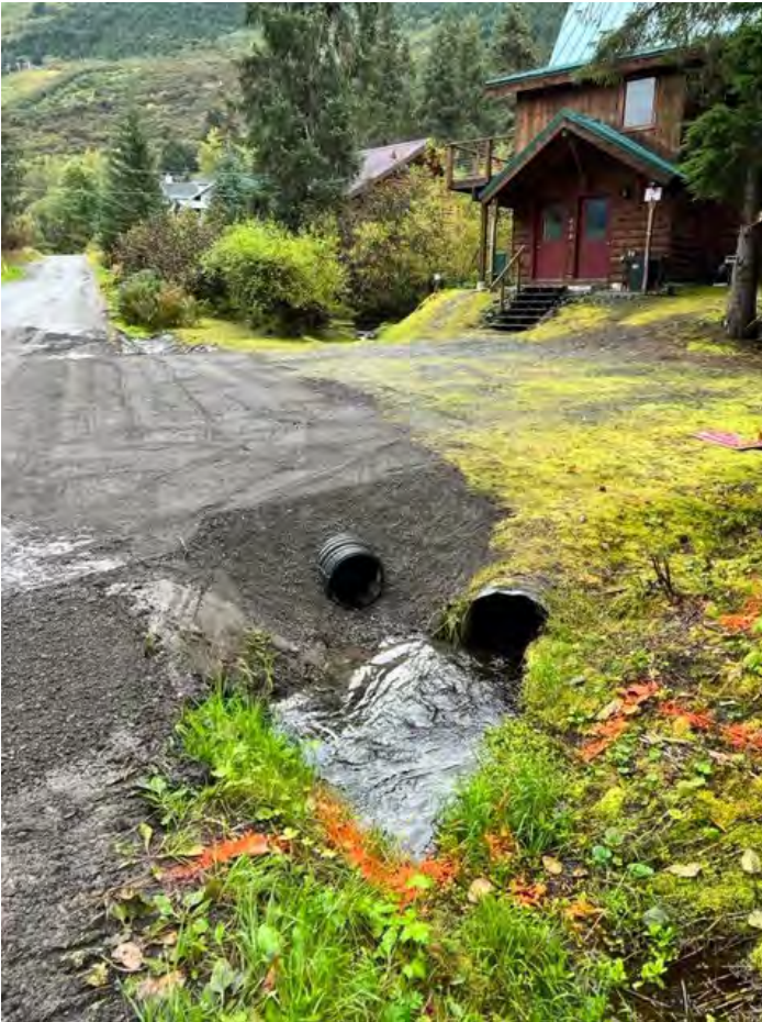
New driveway culvert at 173 Megeve
