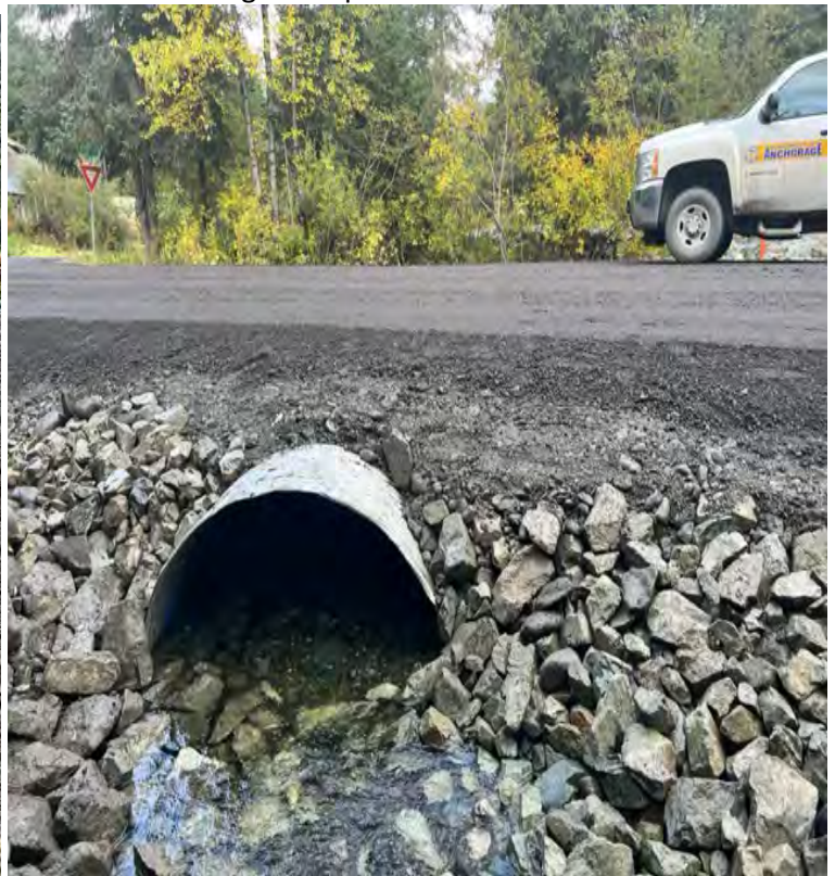
Final new fish passage culvert on Stowe
