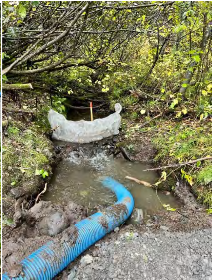
Mesh screening to keep fish out of Stowe construction area
