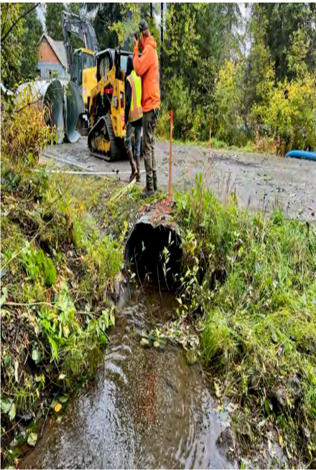
Old cross-culvert on Stowe
