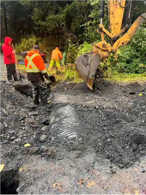
Removing old culvert
