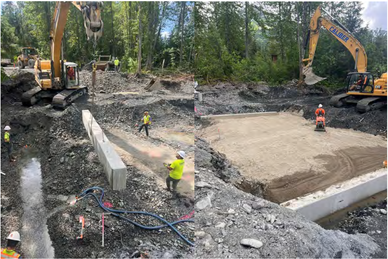
Installing the foundation and abutments for the new box culverts
