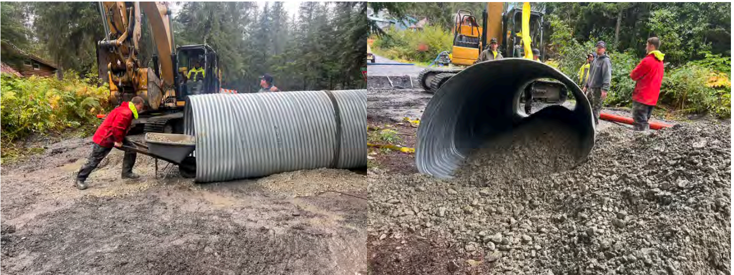
Preloading the culvert with gravel to create a natural bottom for fish to pass over
