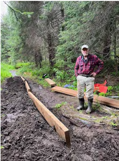
Paul Crews leads first work party of the season adding turnpike to Beaver Pond Trail
