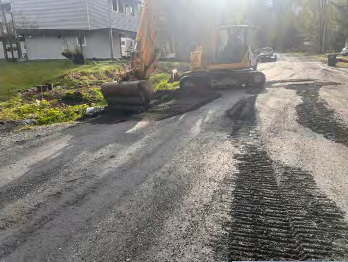
Drainage improvements on Davos Road:
