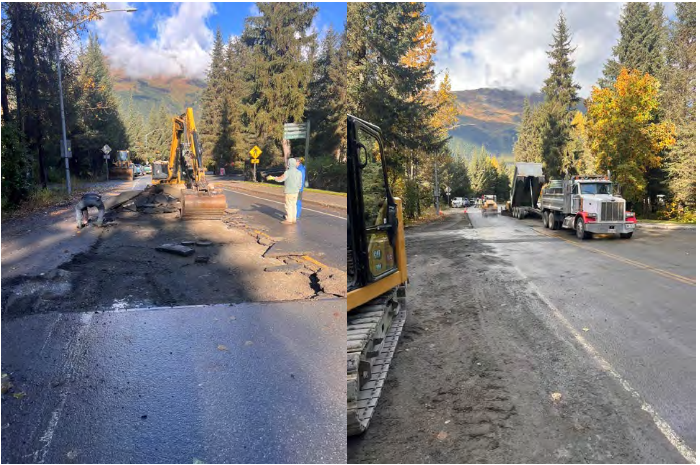
Pavement replacement on Arlberg
