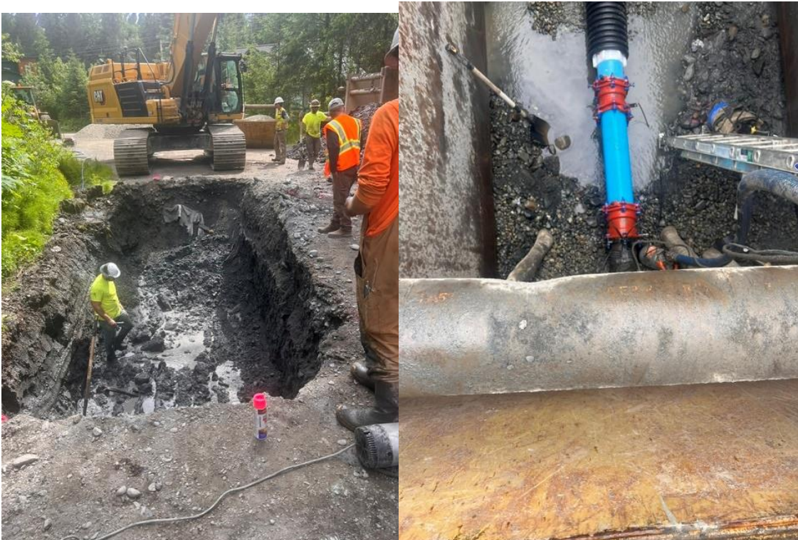
Lowering the water line for the new culvert installation
