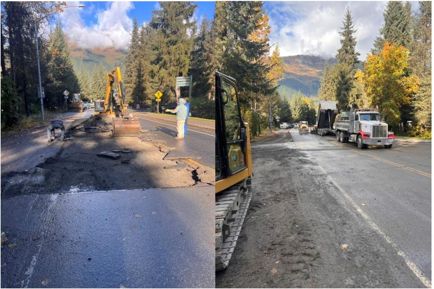
Pavement replacement on Arlberg
