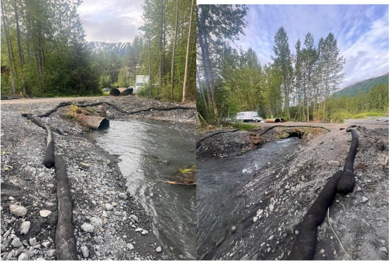
Alyeska Creek at Davos new Fish Passage project: Original culverts
