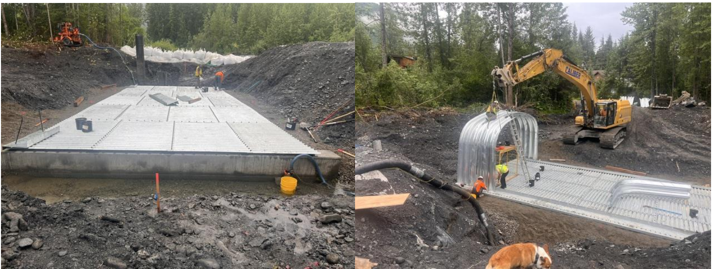
Box culvert floor and start of the structure
