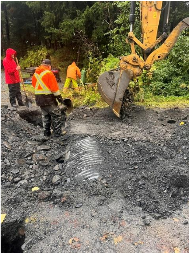
Removing old culvert
