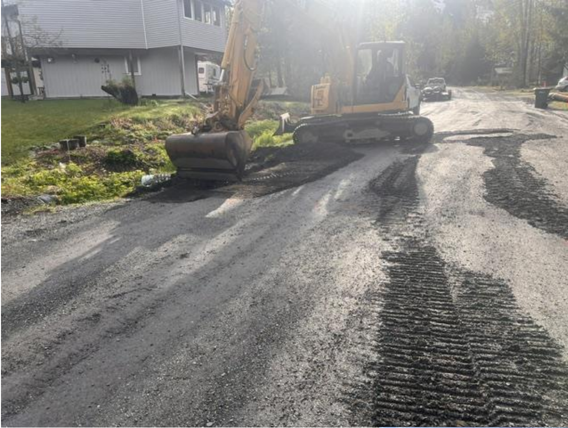
Drainage improvements on Davos Road:
