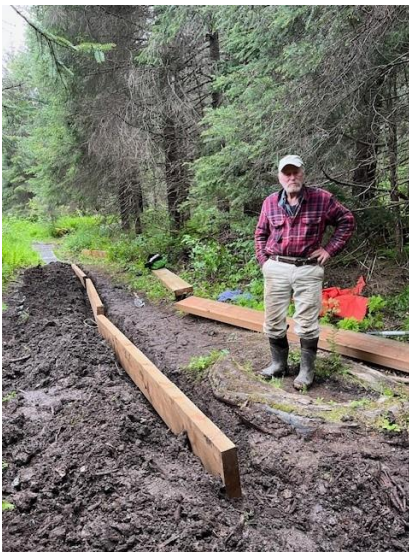
Paul Crews leads first work party of the season adding turnpike to Beaver Pond Trail
