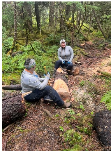
Alaska Trails Crew peeling logs for turnpike
