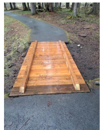
Summer Parks Crew kicked off the season with a new bridge in Forest Fair Park
