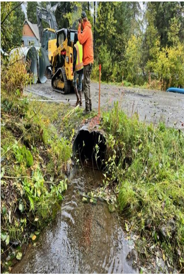
Old cross-culvert on Stowe
