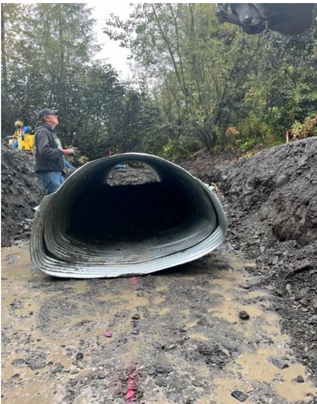
New pipe being installed with in-fill already installed
