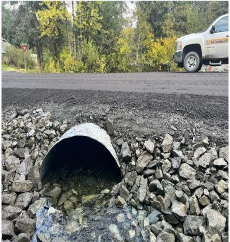
Final new fish passage culvert on Stowe
