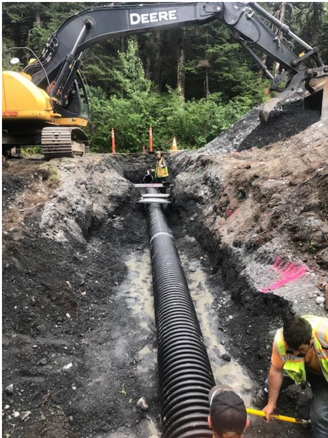
New cross culvert on Arlberg
