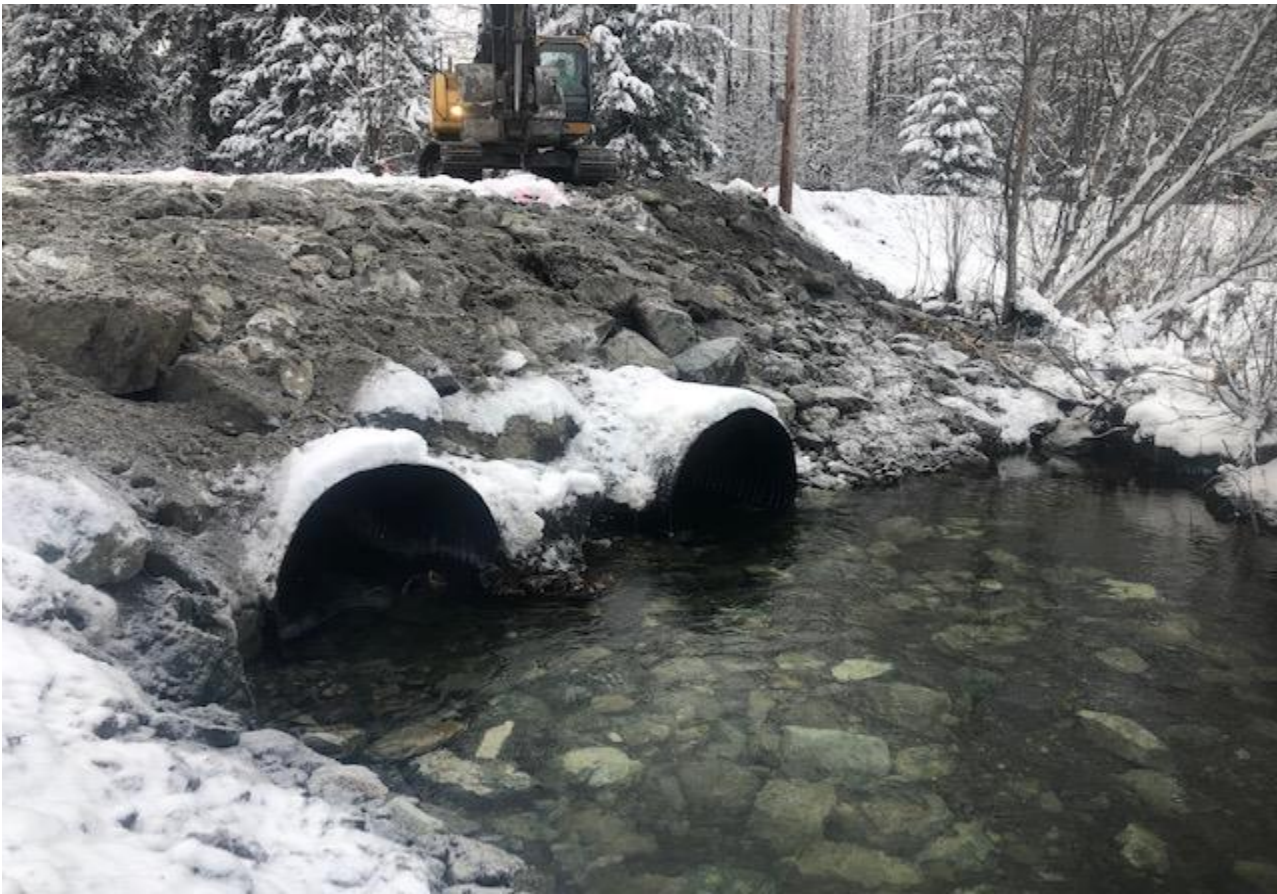
New culverts installed on Ruane
