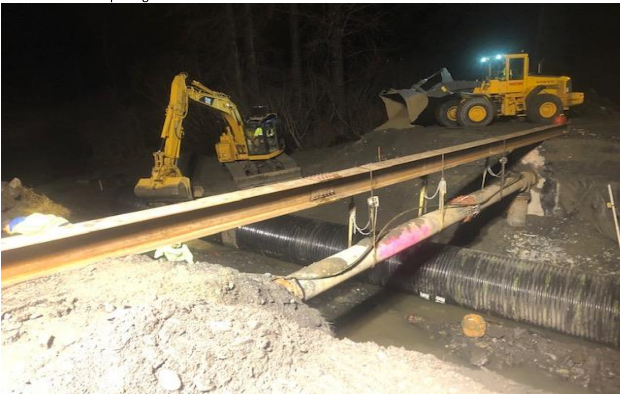
Late night operations to get new culvert in to access AWWU
