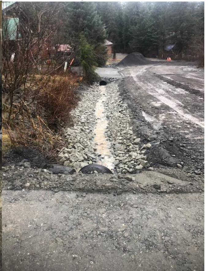
Echo Ridge new Armored Ditch and 24" culverts
