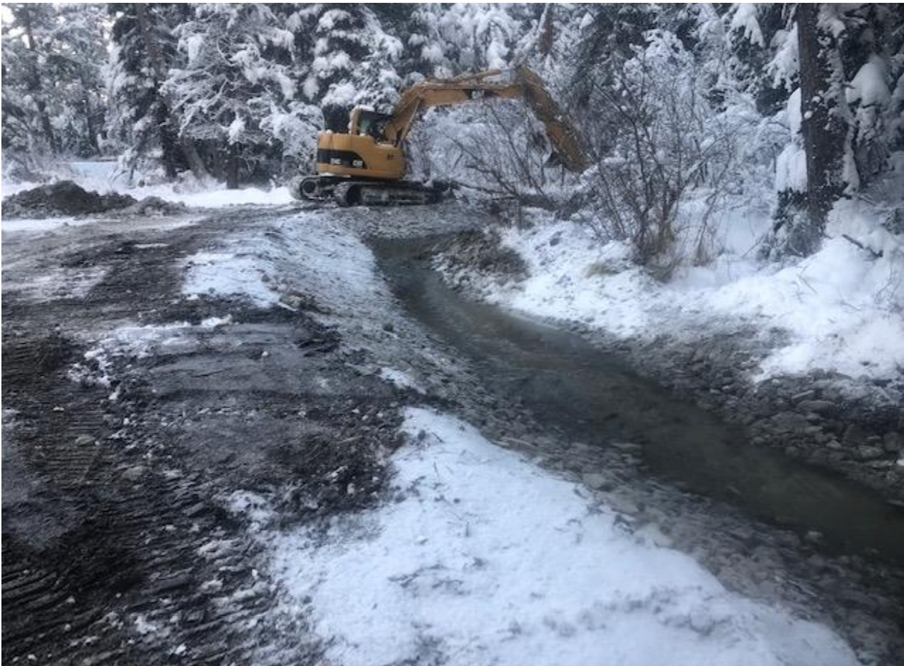
Arlberg 5k parking lot stream cleaned out of storm debris and channel was rebuilt and armored.
