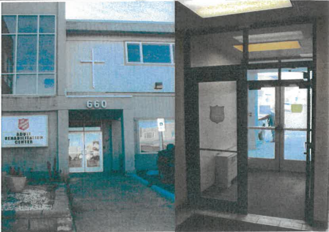
Photograph 10.2-3 – Main entry doors, in fair condition
