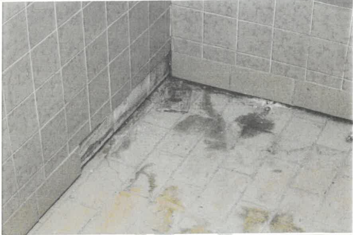
Photograph 17.3-1 – Ceramic tile floor and walls in level 2 bathrooms
