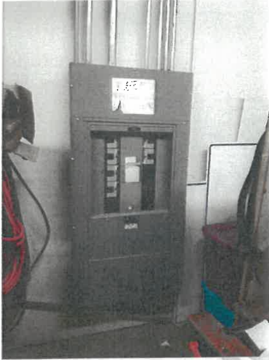
Photos 14.0-9 & 10: 480V MDPH and Warehouse Branch Panels
