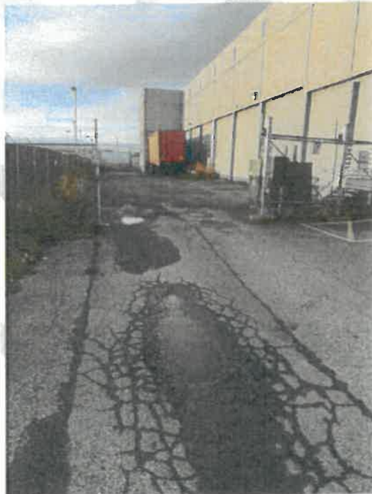
Photograph 5.1-1: East Driveway, Security Gate, Loading Dock
