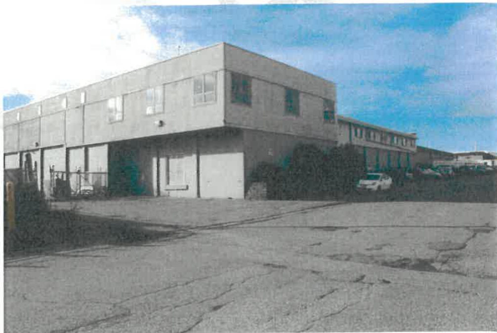
Photograph 10.1-1 – Building exterior, northeast corner
