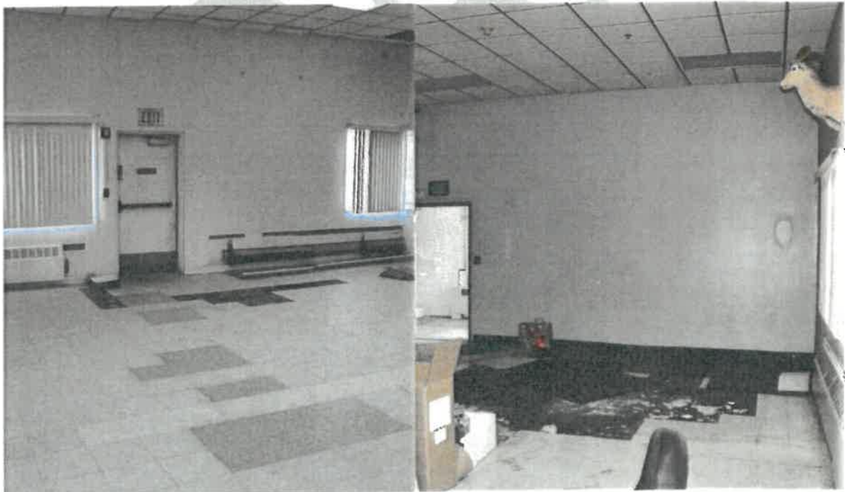
Photograph 17.3-2 – VCT flooring in Dining room (left) and Day/Billiard room (right)
