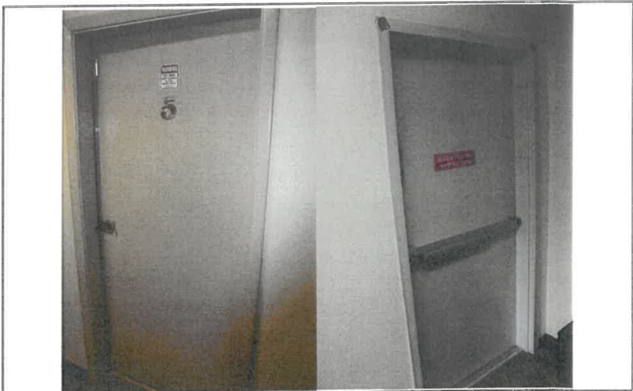
Photograph 17.5-1 – Dormitory doors are missing hardware (left), metal doors in fair condition (right)
