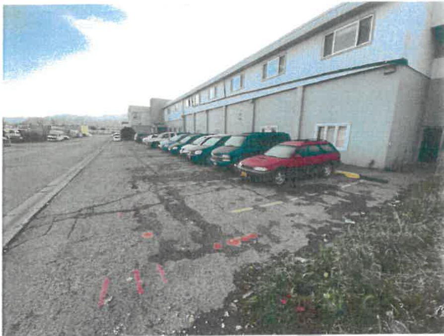
Photograph 4.0-1 – E. 48 th Ave. frontage
