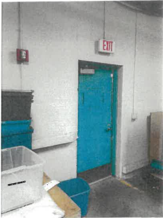
Photos 16.0-6 & 7: Warehouse Exit Signs and Warehouse EM Lights
