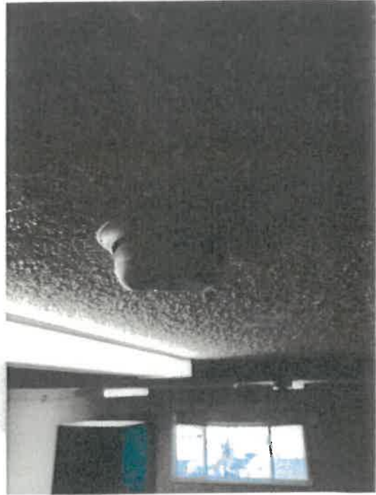
Photos 16.0-3 & 4: Fire Alarm System Smoke Detector and Residential Smoke Alarm
