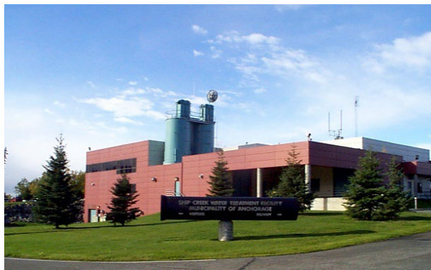
Ship Creek Water Treatment Facility
