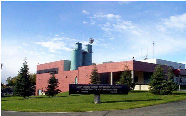
Ship Creek Water Treatment Facility
