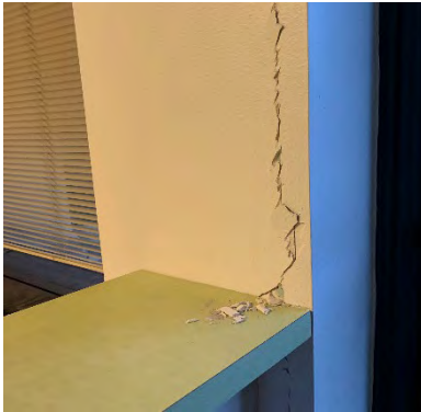
Figure 5.38. University of Alaska, Eagle River campus, partition and nonstructural wall damage. The top left photo shows an unstable partition wall with out-of-plane deformation. The building is flexible steel-moment frame, and the nonstructural wall components were not compatible with withstanding the large frame deformations (photos: Wael Hassan).
