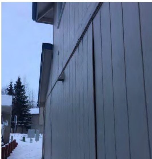
Figure 4.35.a. Shear wall damage in wood-frame residential buildings in Eagle River (photos: PND Engineers 17 ).
