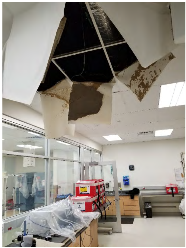
Figure 7.25. Laboratory ceiling damage due to water flooding at BBA (photos: BBA).
