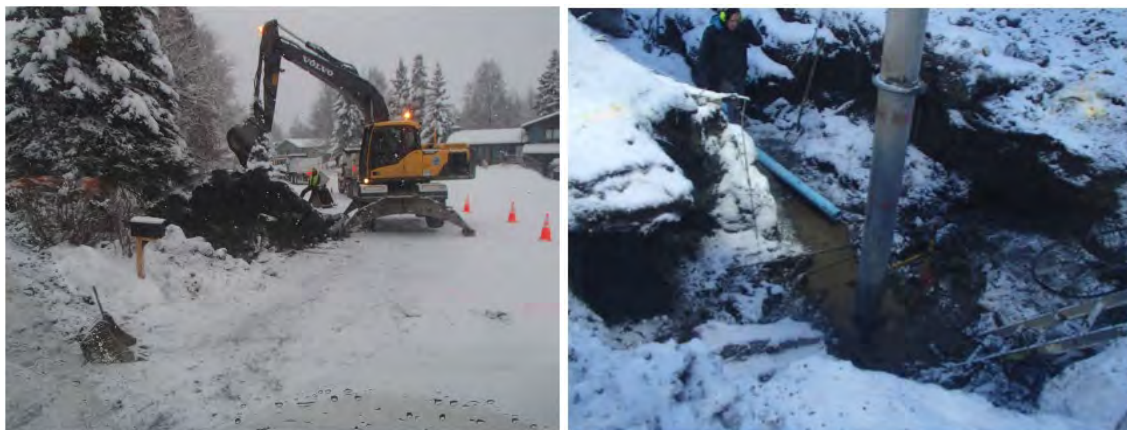
Figure 9.9. Emergency excavation to damaged sewer service (photos: AWWU).
