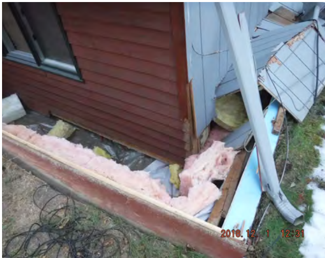
Figure 4.38.b. Residential single-family housing severe shear wall and nailed-connection sliding/uplift from foundation damage in a residential building in Anchorage (photos: MOA).
