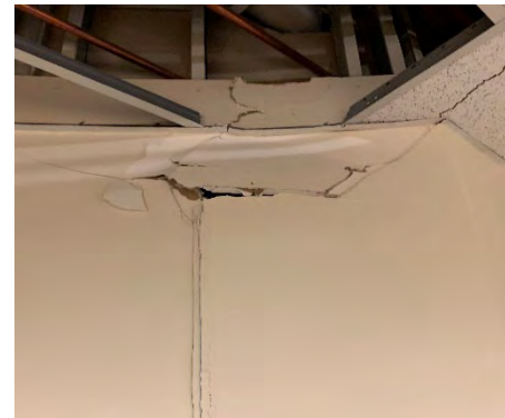
Figure 5.38. University of Alaska, Eagle River campus, partition and nonstructural wall damage. The top left photo shows an unstable partition wall with out-of-plane deformation. The building is flexible steel-moment frame, and the nonstructural wall components were not compatible with withstanding the large frame deformations (photos: Wael Hassan).
