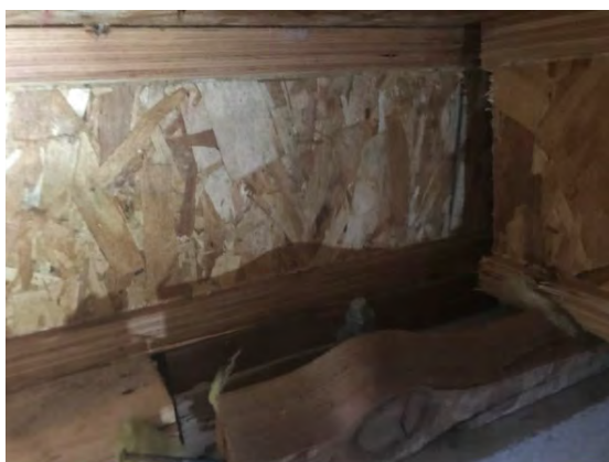
Figure 4.35.b. Shear wall damage in wood-frame residential building in Eagle River (photos: PND Engineers).
