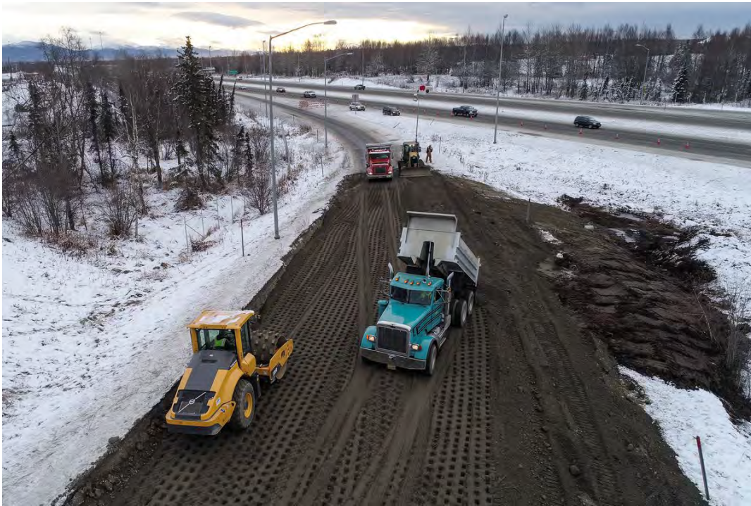
Figure 8.24. Repair of off-ramp from Minnesota Drive to International Airport Road (photo: Anchorage Daily News).
