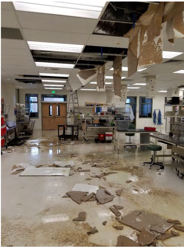
Figure 7.25. Laboratory ceiling damage due to water flooding at BBA (photos: BBA).
