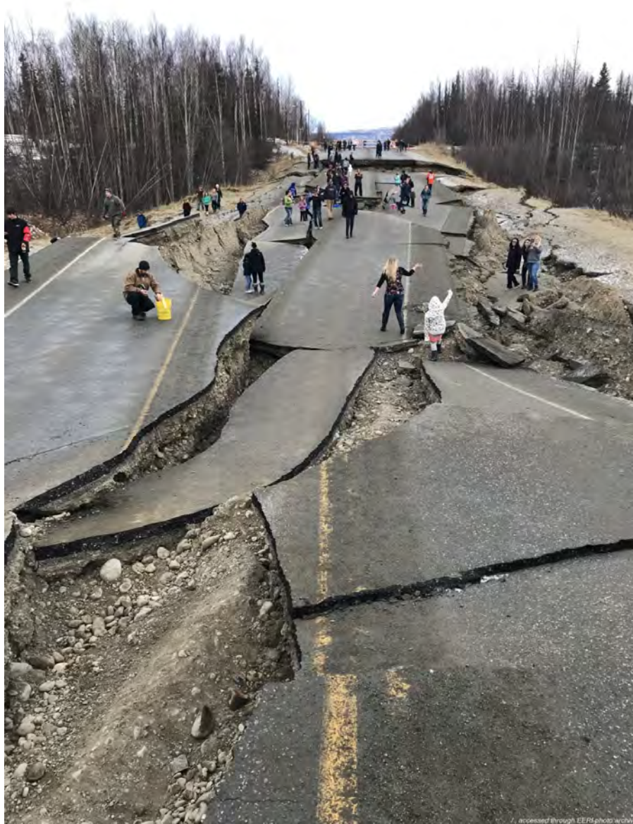
Figure 8.20. Vine Road earthquake damage (photo: EERI Clearinghouse).
