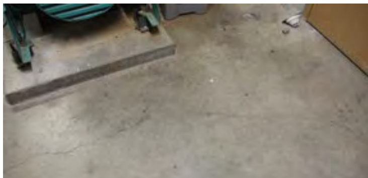
Figure 6.9. Cracking in reinforced concrete basement floor at Eagle River Elementary (photos: Chris Motter).
