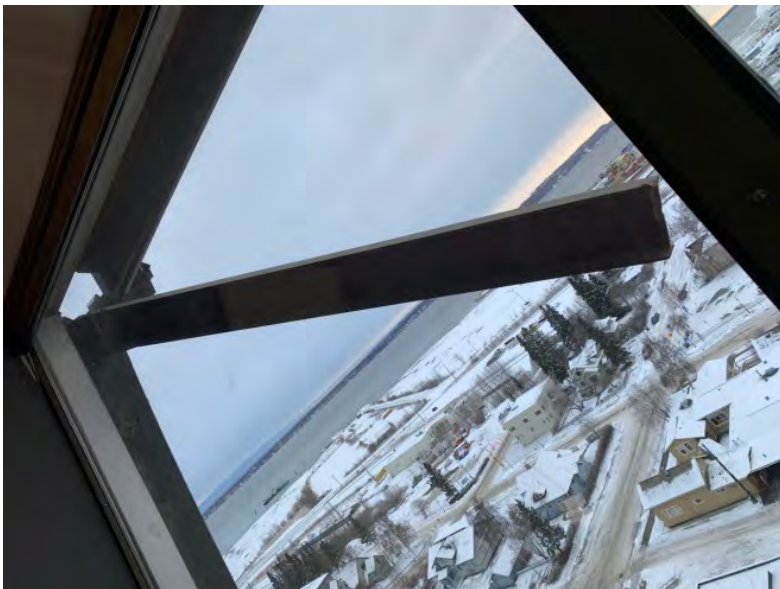
Figure 4.44. (a) Girdwood Wastewater Treatment Facility operations building with a sheared steel crane beam not connected at one end (photo: AWWU); (b,c) Hilton Anchorage steel soffit-beam failure (photo: PND Engineers).
