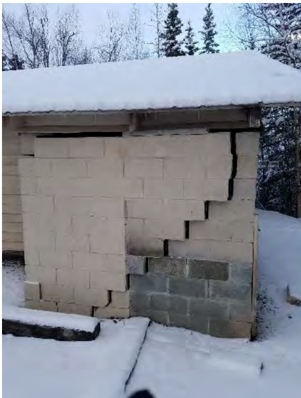
Figure 4.33. Severe masonry heater housing unit damage in Mat-Su (Photos Janise Rodgers).
