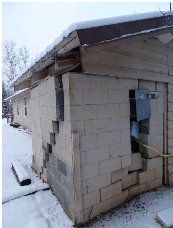
Figure 4.33. Severe masonry heater housing unit damage in Mat-Su (Photos Janise Rodgers).
