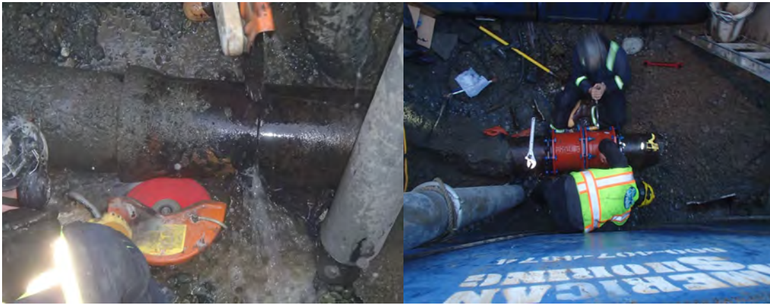
Figure 9.6. Emergency excavation to repair a damaged water main on Airport Drive (photos: AWWU).
