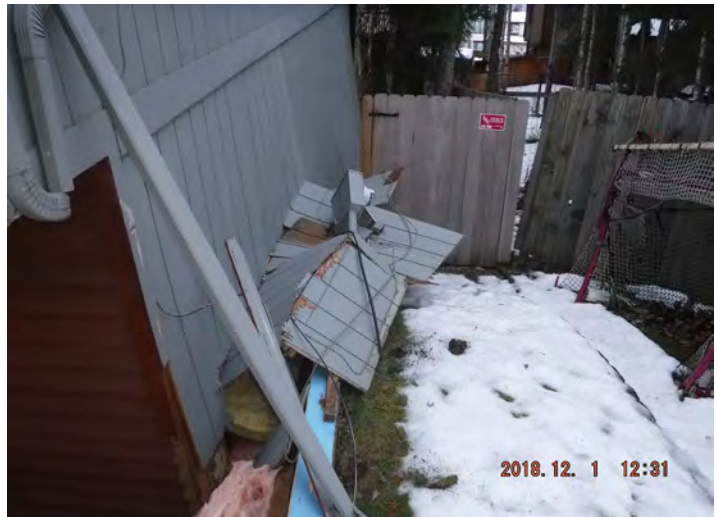
Figure 4.38.b. Residential single-family housing severe shear wall and nailed-connection sliding/uplift from foundation damage in a residential building in Anchorage (photos: MOA).
