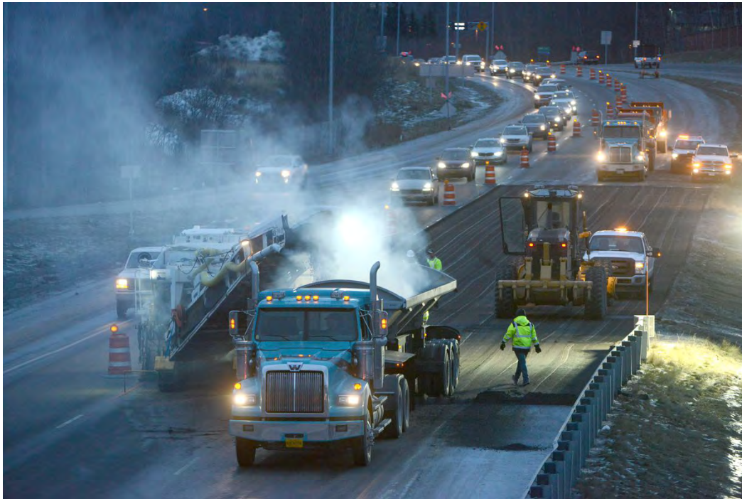
Figure 8.23. Repair of buckled pavement on Seward Highway between 36th Avenue and Tudor Road (photo: Anchorage Daily News).
