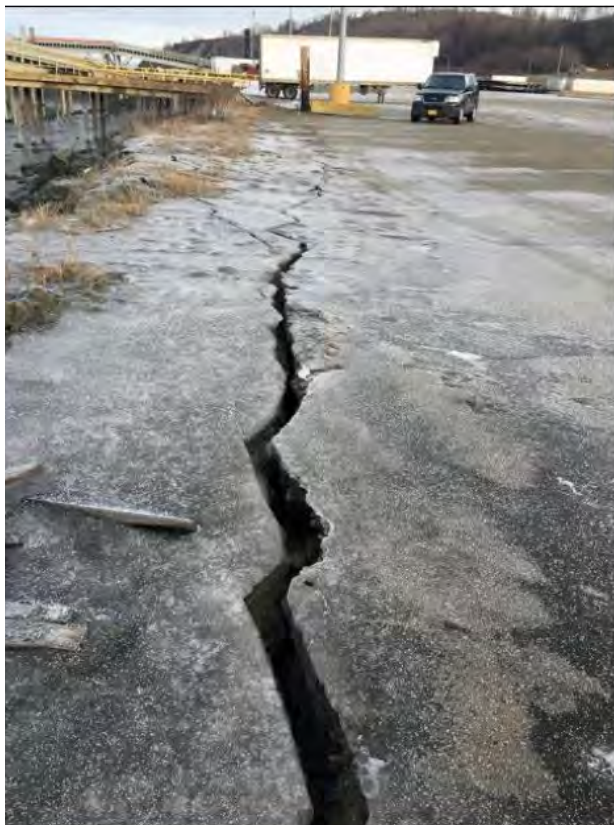
Figure 9.22. Slope failures along the length of container docks (photos: Port of Alaska).
