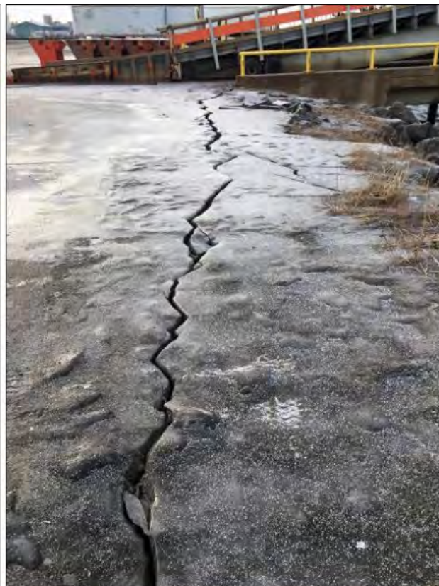
Figure 9.22. Slope failures along the length of container docks (photos: Port of Alaska).
