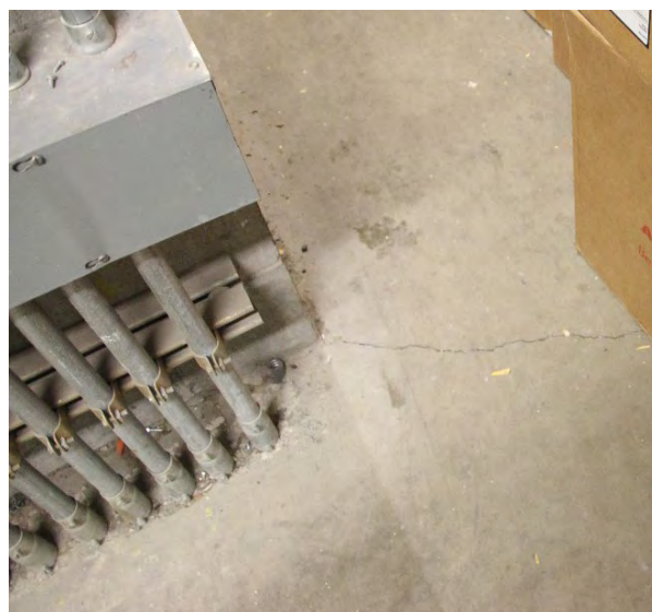
Figure 6.9. Cracking in reinforced concrete basement floor at Eagle River Elementary (photos: Chris Motter).
