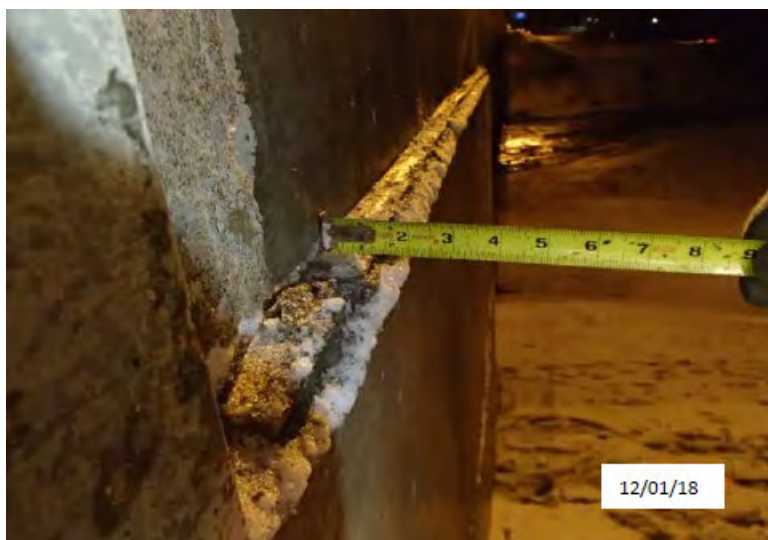
Figure 8.11. Culvert damage (photo: Jesse Escamilla and Ben Fetterhoff).
