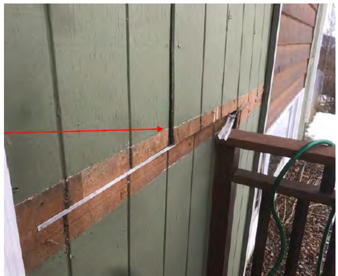
Figure 4.35.a. Shear wall damage in wood-frame residential buildings in Eagle River (photos: PND Engineers 17 ).
