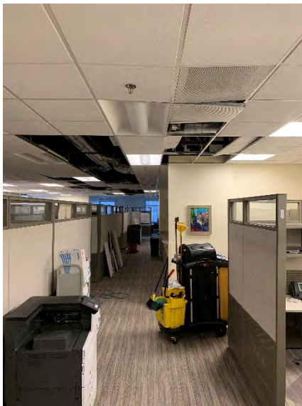
Figure 7.28. VA Hospital in Anchorage, nonstructural ceiling damage (photos: Erol Kalkan).
