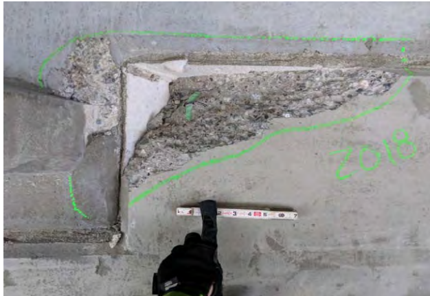
Figure 8.9. Shear key damage (photos: ADOT&PF).
