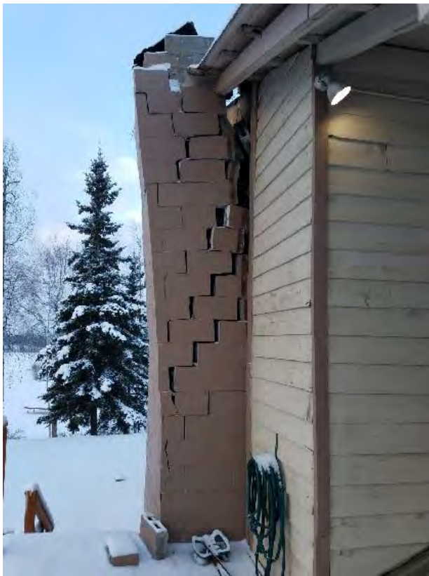
Figure 4.32. Masonry chimney partial collapse (photos: Janise Rodgers).
