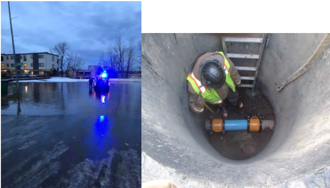
Figure 9.7. Emergency excavation to repair a damaged water main on Second Street, Cordova (photos: AWWU).
