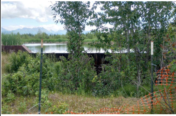
View of the sheet pile dam and man-made wetlands located approximately 800ft southeast of the subject property. View is to the southeast.
