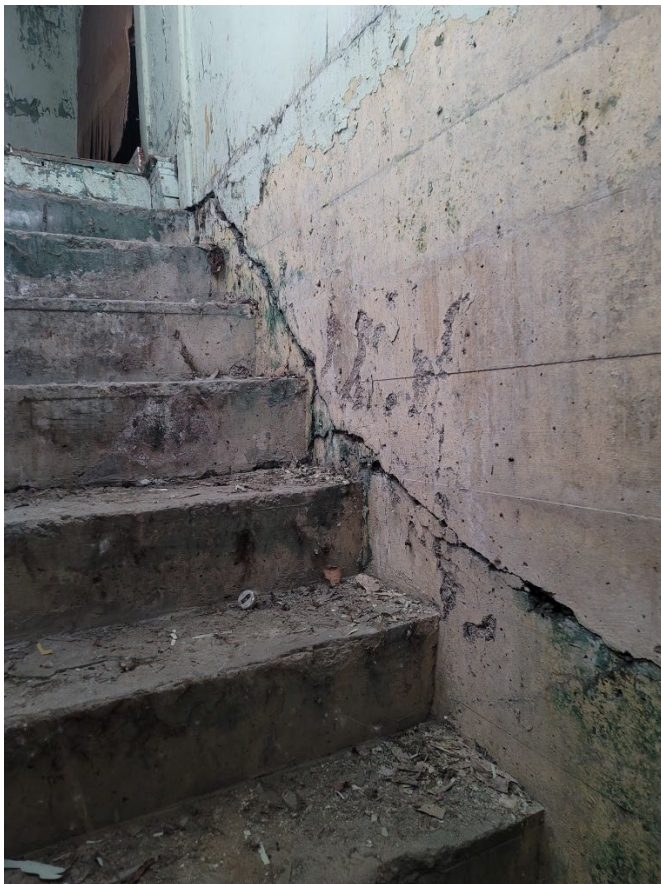
Figure 14. The stairwell to the basement in the south addition of Building A. A crack parallels the stair slope as well as spalling, vegetative growth, and staining from water infiltration (2023).
