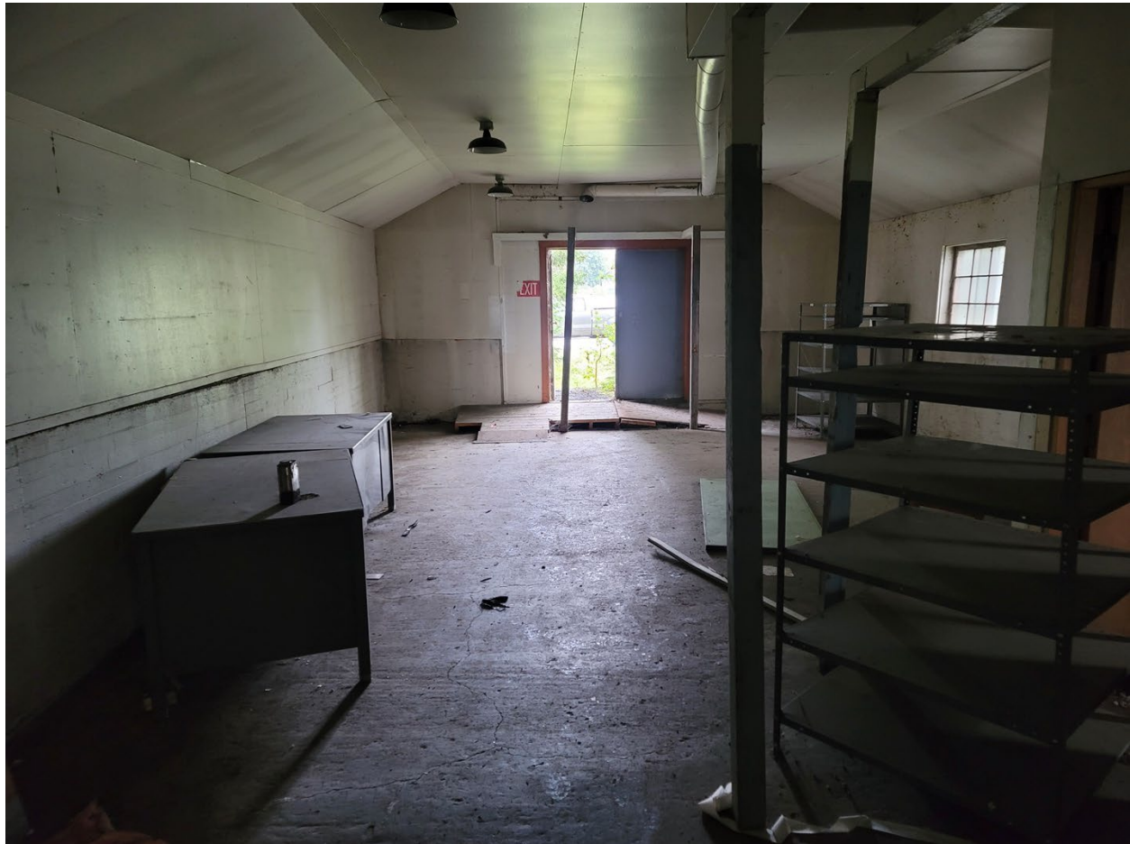
Figure 20. Bare concrete foundation serves as the floor in the northernmost section of Building B (2023).
