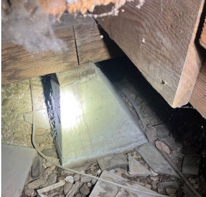
Figure 13. One of the pyramidal concrete piers below the central portion of Building A (2023).)
