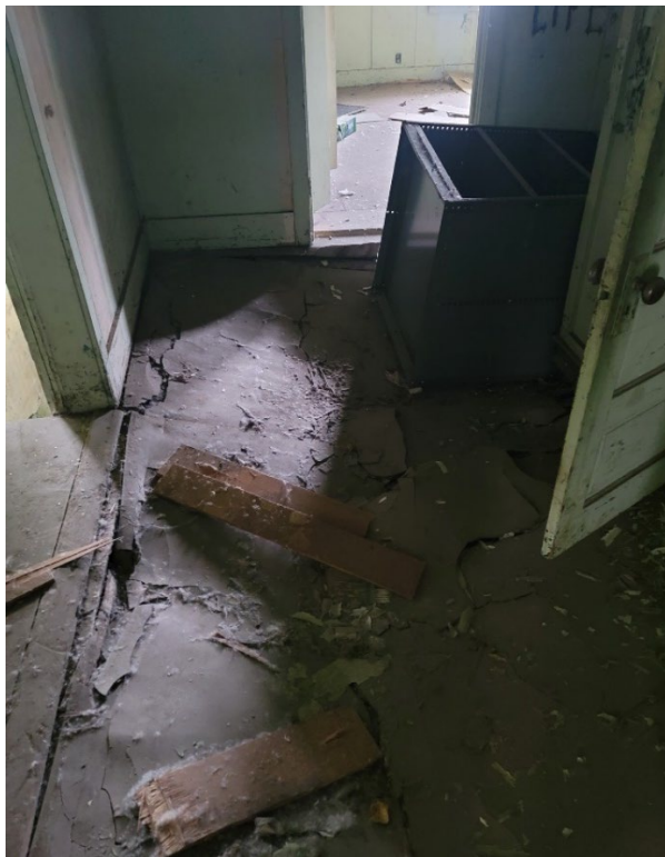
Figure 13. A collapsed floor in Building A (2023)
