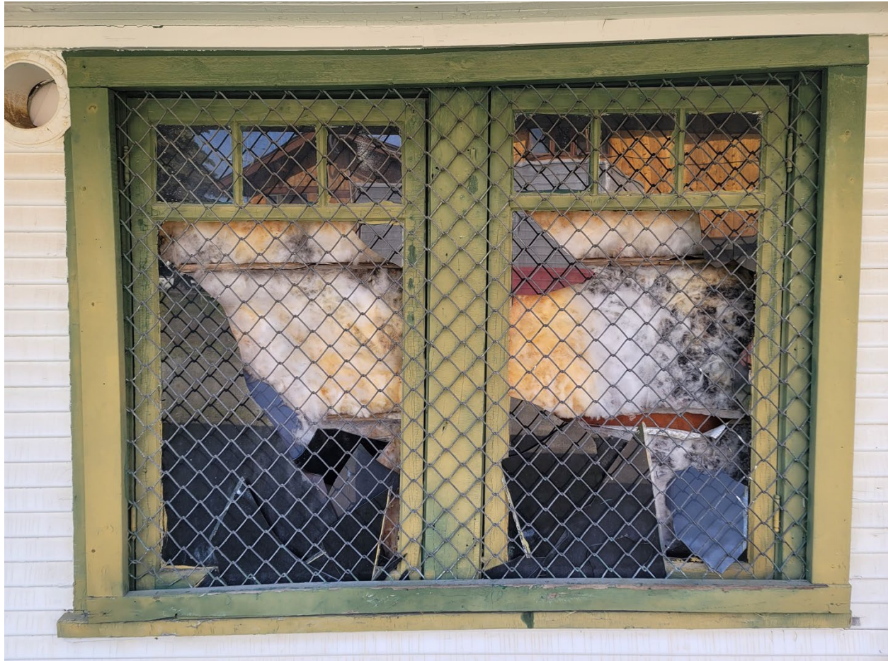
Figure B27. The southernmost window on the west façade of Building A. The photograph shows the broken glazing as well as the misalignment of the window framing due to the building's uneven settlement over time (©TNSDS 2023).
