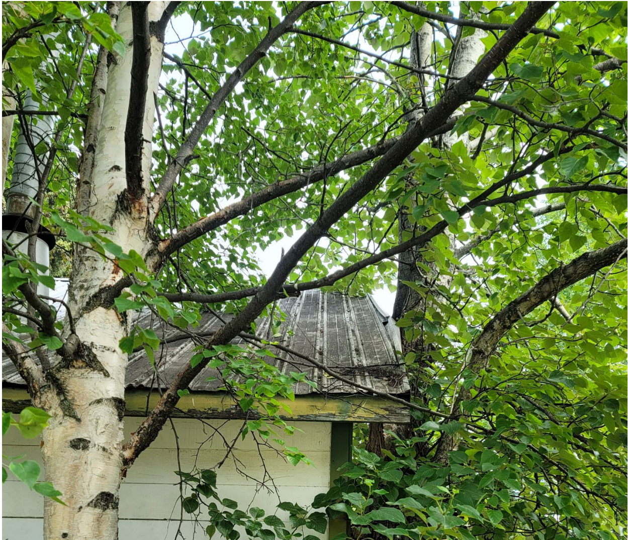
Figure B20. Detail photograph of Building C. The photo shows how the birch tree that has grown against the southeast façade of the building has begun to displace the roofing materials (©TNSDS 2023).
