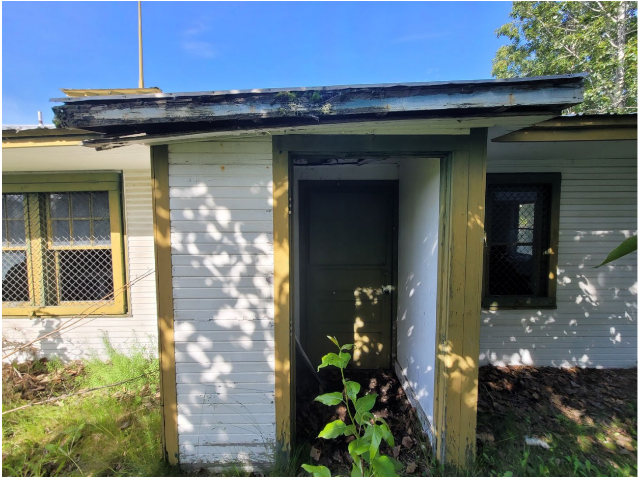
Figure B33. Arctic entry in the east façade of Building A (©TNSDS 2023).
