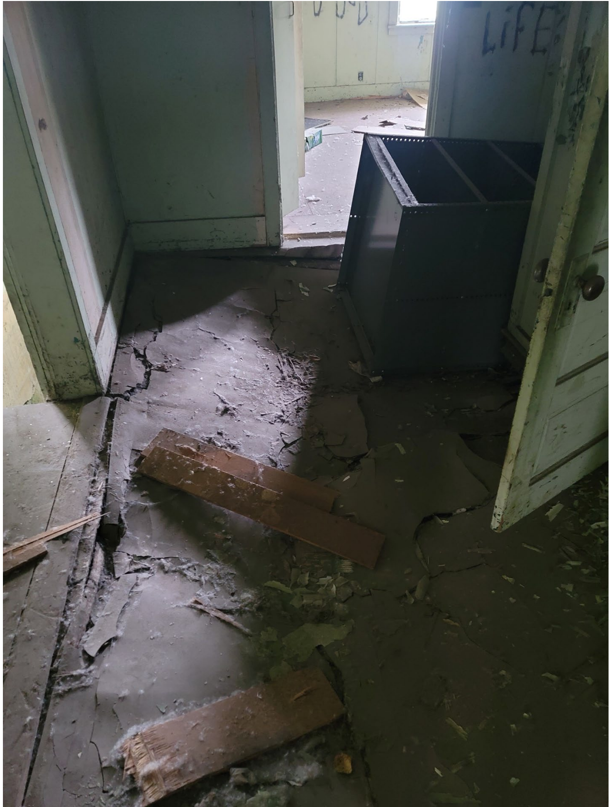
Figure B54. Photograph of one of the collapsed floors in Building A (©TNSDS 2023).
