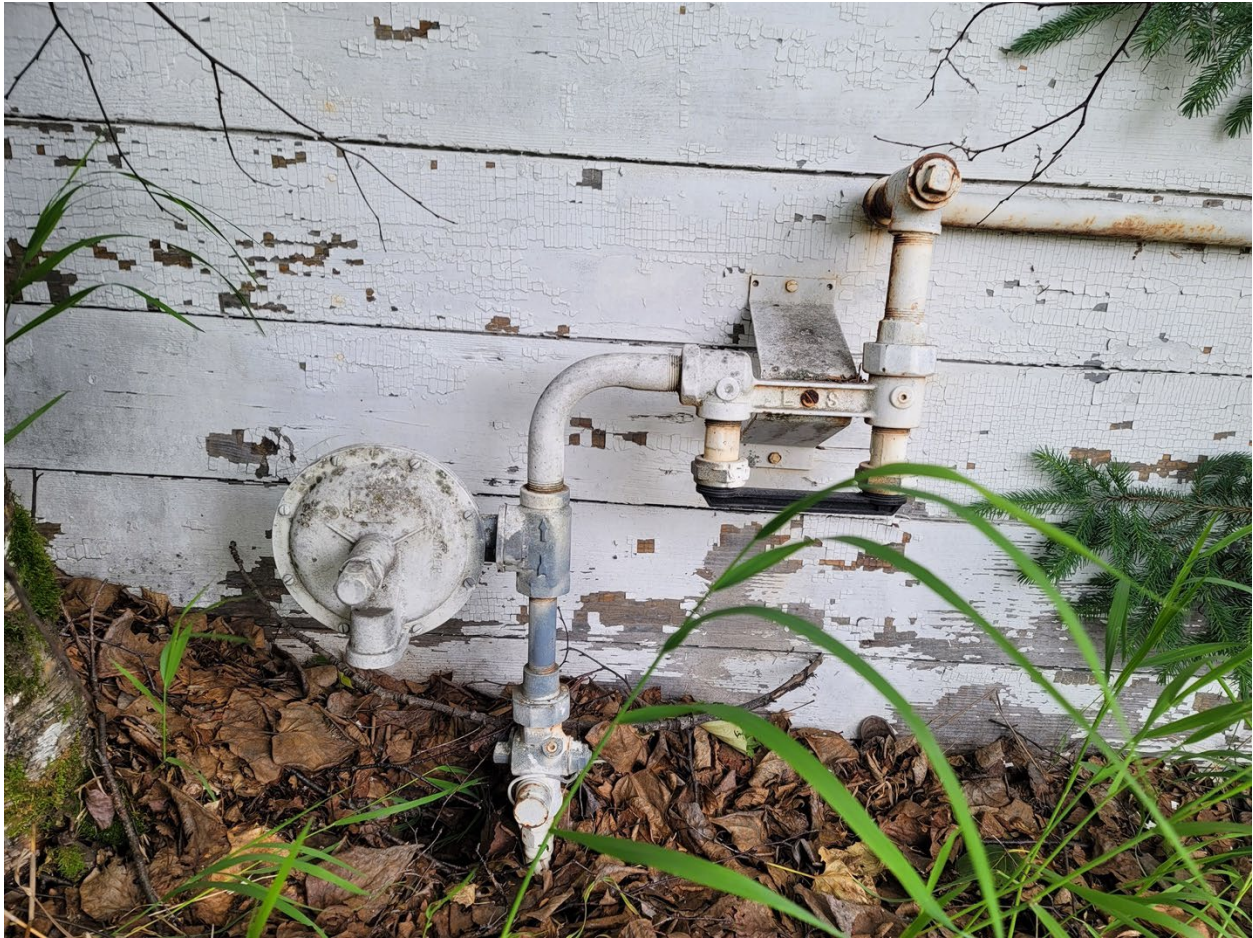
Figure B22. Detail photograph of the utilities installed on the southwest façade of Building C. The photograph shows the deterioration of the paint along the bottom boards of the building. It also demonstrates the crazing and cracking of the older paint as well as sections where the older paint has been removed and reapplied such that no cracking or crazing is present (©TNSDS 2023).
