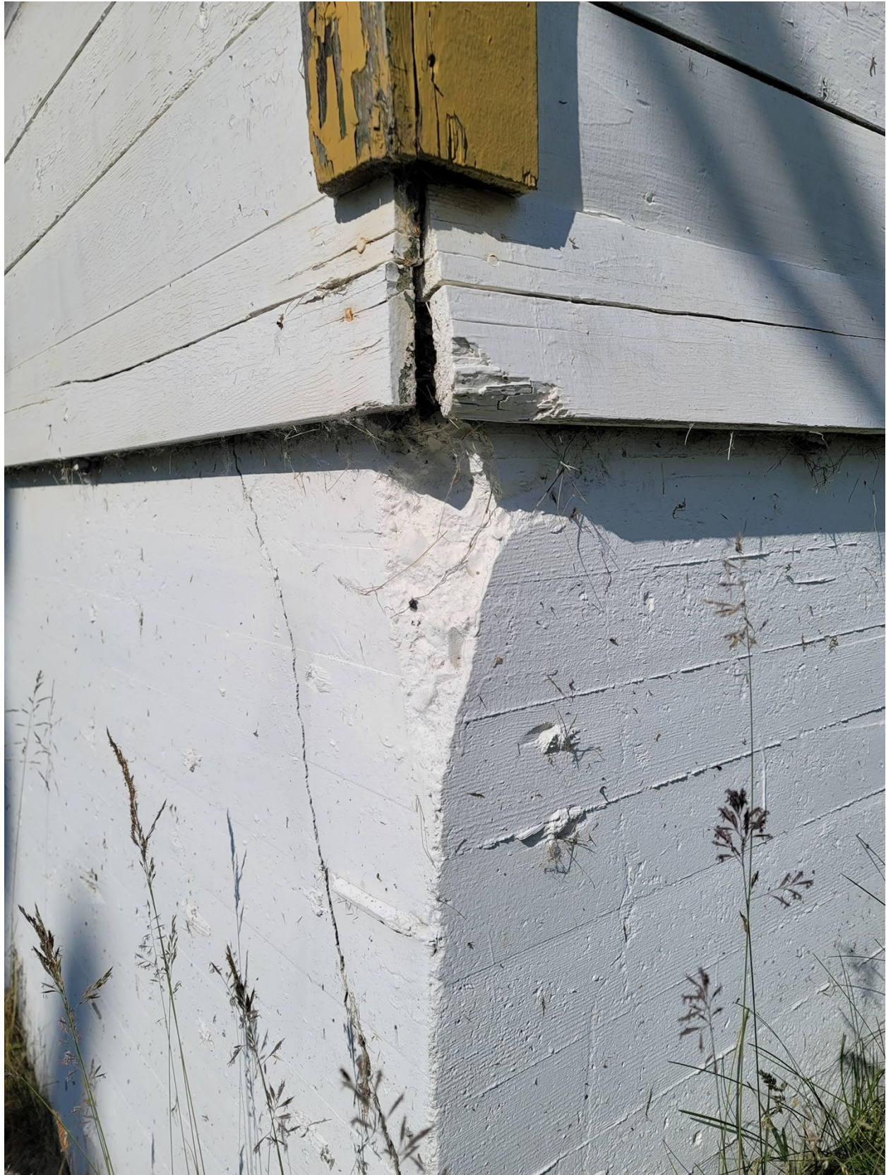
Figure B16. Detail photograph of the southeast corner of Building B. The photograph shows the concrete foundation, lap siding, and skirtboard and demonstrates the spalling happening to the foundation (©TNSDS 2023).
