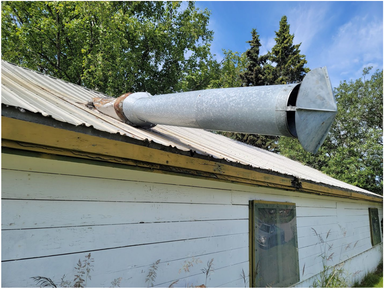
Figure B47. Detail photograph of the collapsed chimney on Building B (©TNSDS 2023).
