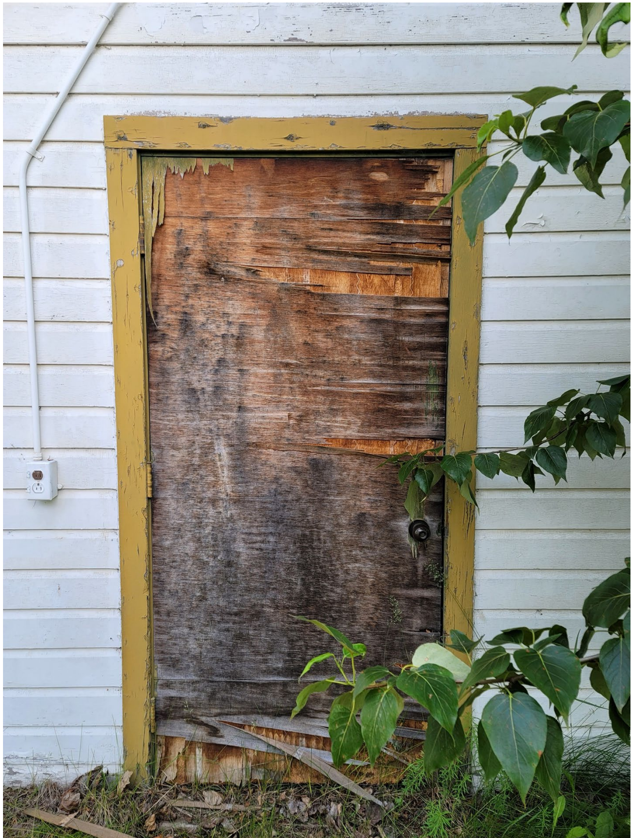
Figure B36. Detail photograph of the door in the southwest facade of the addition of Building B. The photograph shows the significant deterioration of the door material (©TNSDS 2023).
