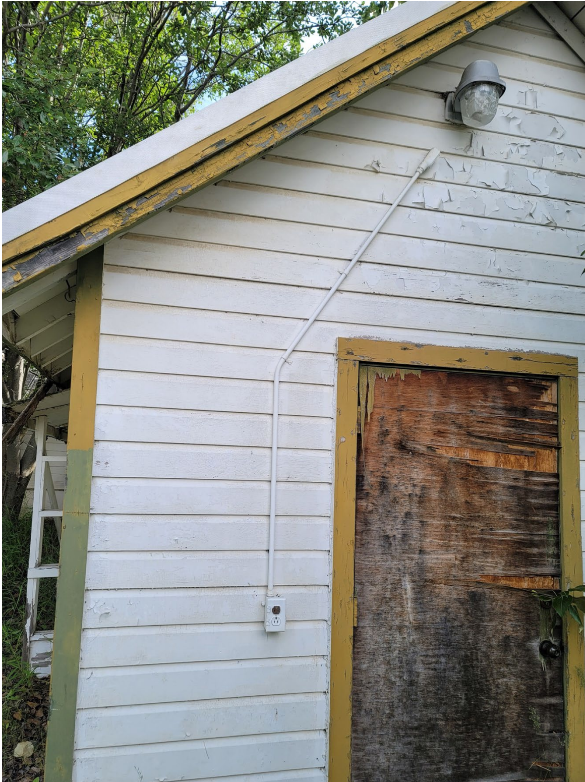
Figure B19. The southwest façade of the addition to Building B, showing the cracking, crazing, and peeling of the paint on the siding (©TNSDS 2023).
