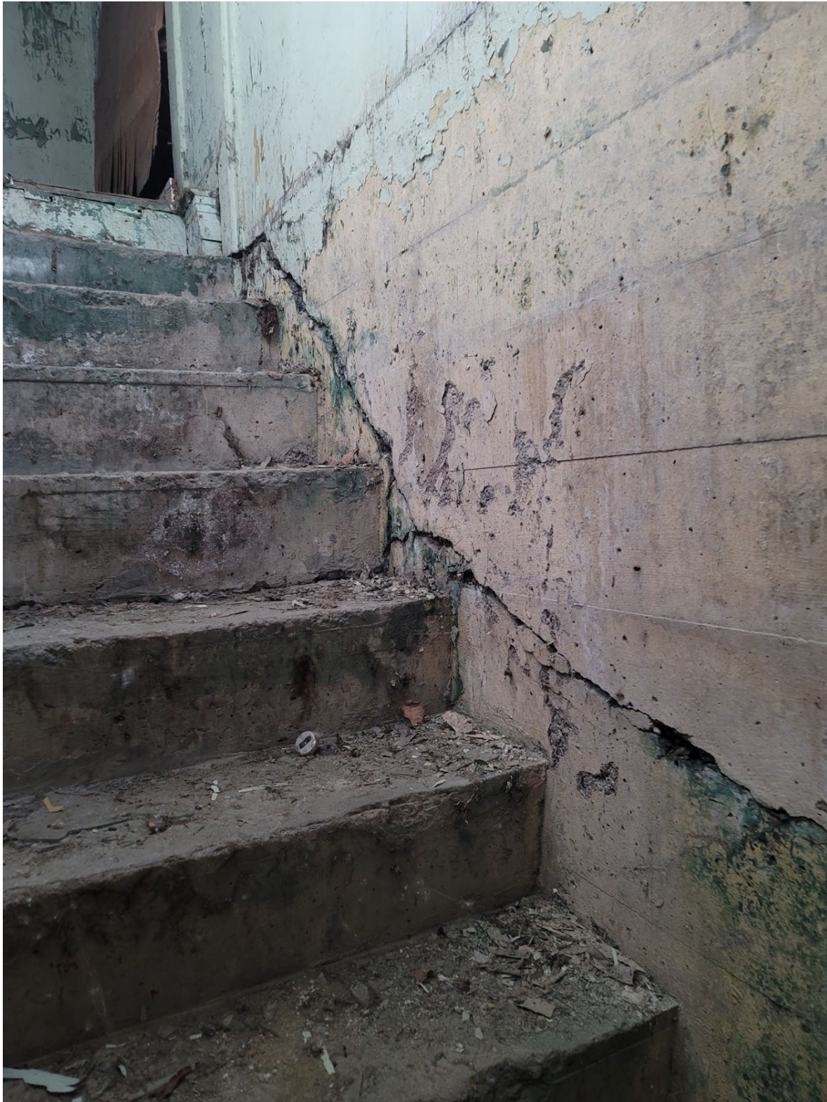
Figure B56. Detail photo of the stairs that lead from the interior of Building A to the basement in the south addition. The photograph shows the slope of the crack paralleling the stair slope as well as spalling, vegetative growth, and staining from water infiltration (©TNSDS 2023).
