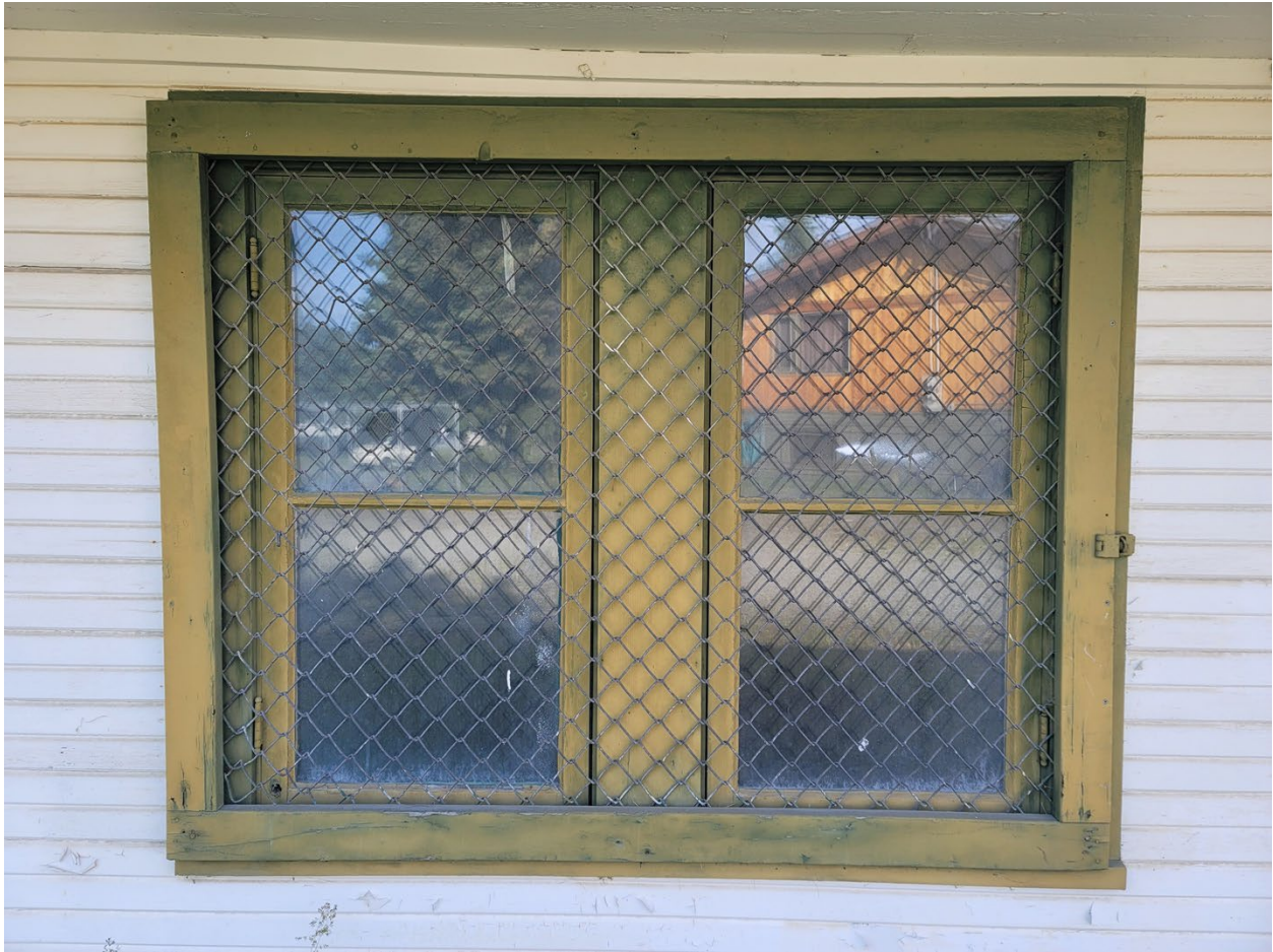
Figure B23. Detail photograph of one pair of one-over-one sash windows in the west façade of Building A (©TNSDS 2023).
