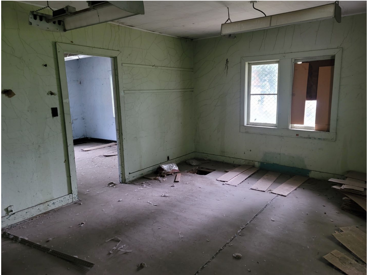
Figure B51. Interior of the northernmost rooms in Building A. The photograph shows the holes and cracks in the flooring and wall finishes (©TNSDS 2023).
