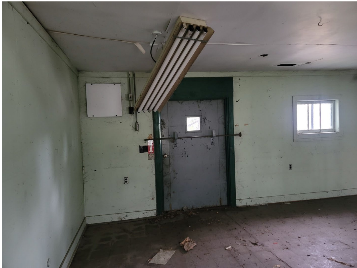
Figure B42. Interior view of the doorway in the southwest façade of Building C. The photograph shows the metal bar installed on the door to prevent it from being opened fully (©TNSDS 2023).
