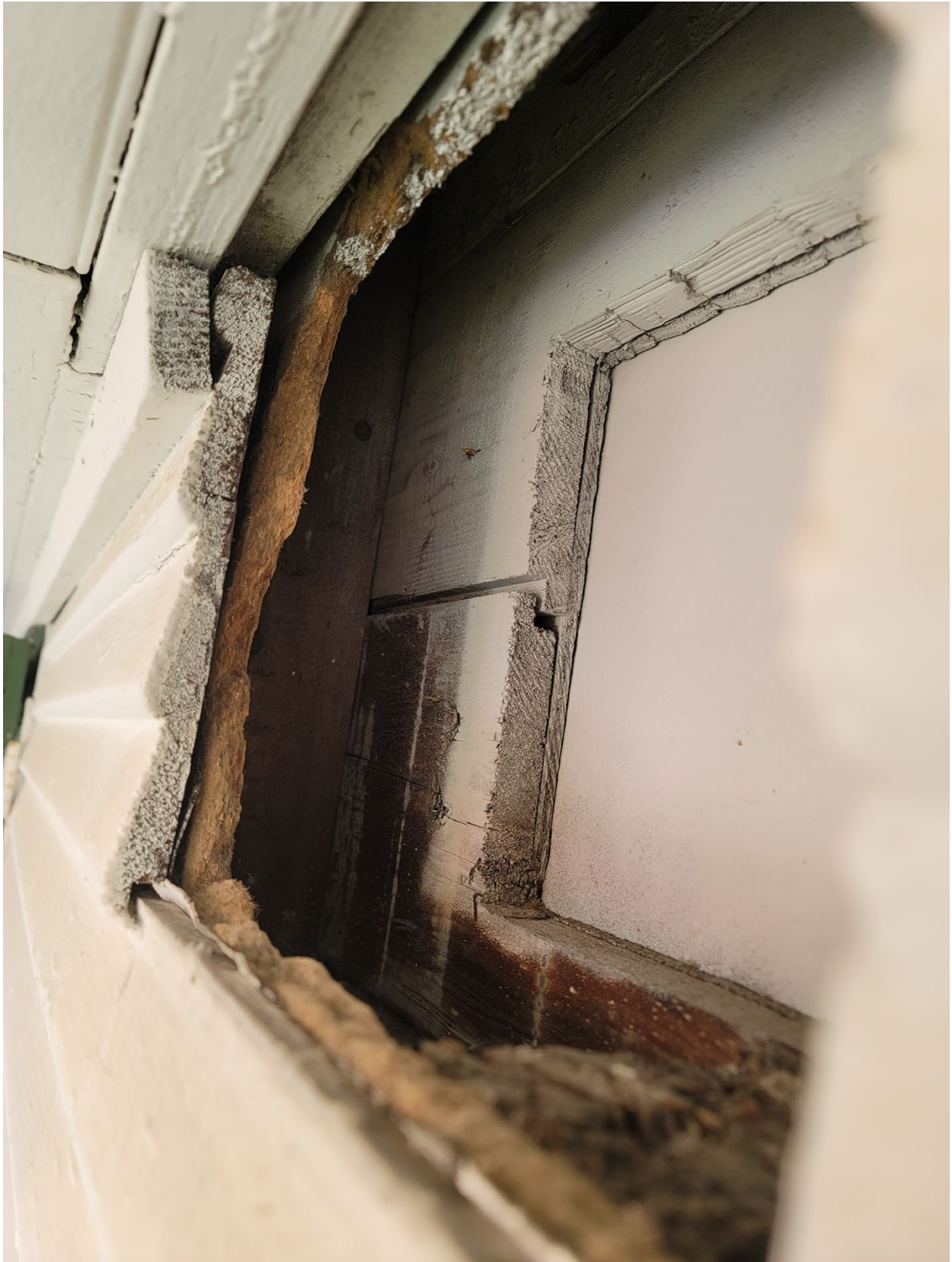
Figure B17. Detail photograph showing the current siding overlaying older siding layers on Building A (©TNSDS 2023).
