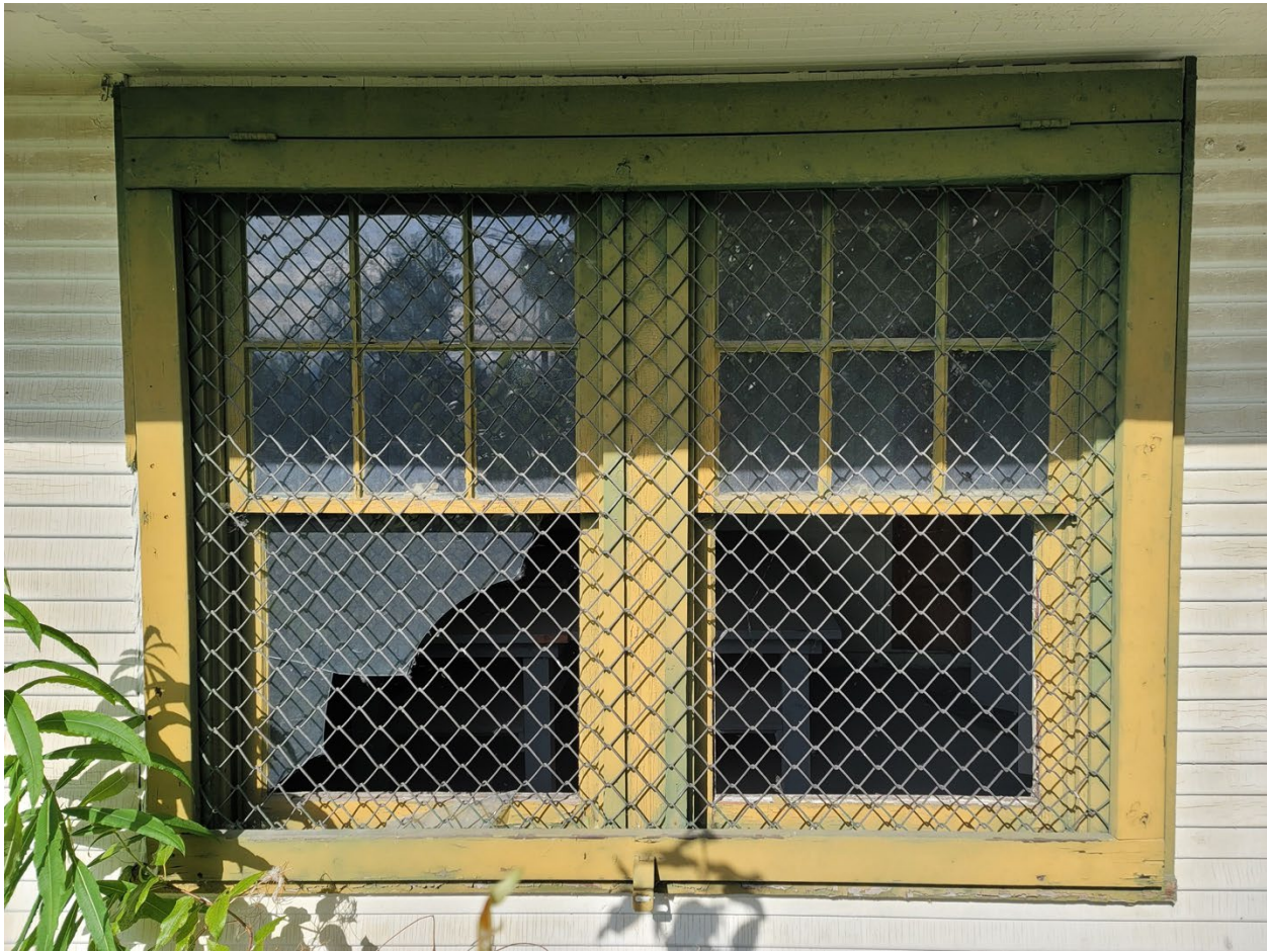
Figure B25. Detail photograph of the six-over-one sash windows in the east façade of Building A (©TNSDS 2023).
