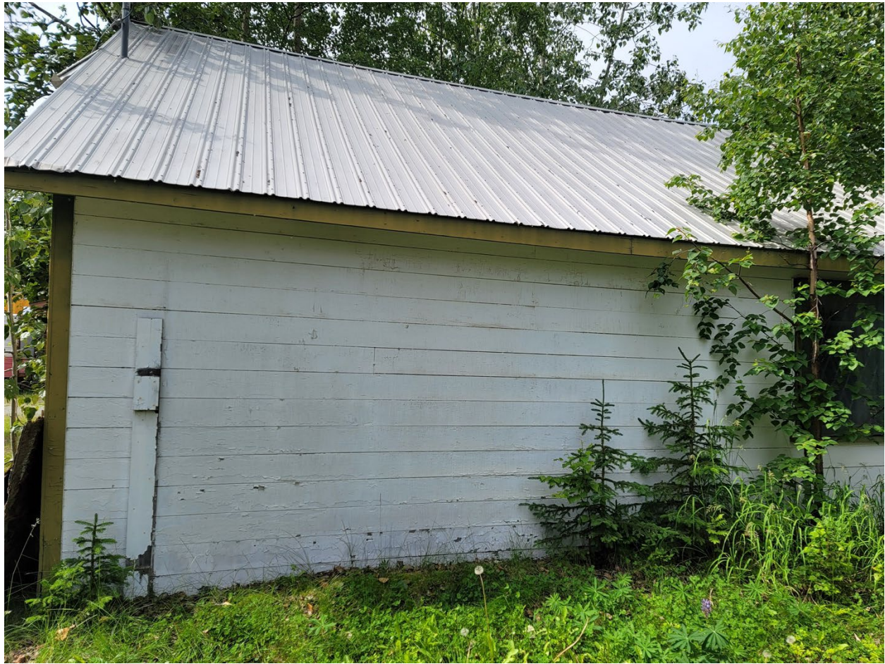
Figure B50. Photograph of the northeast façade of Building C, showing the onion corrugated polycarbonate or PVC roofing material (©TNSDS 2023).
