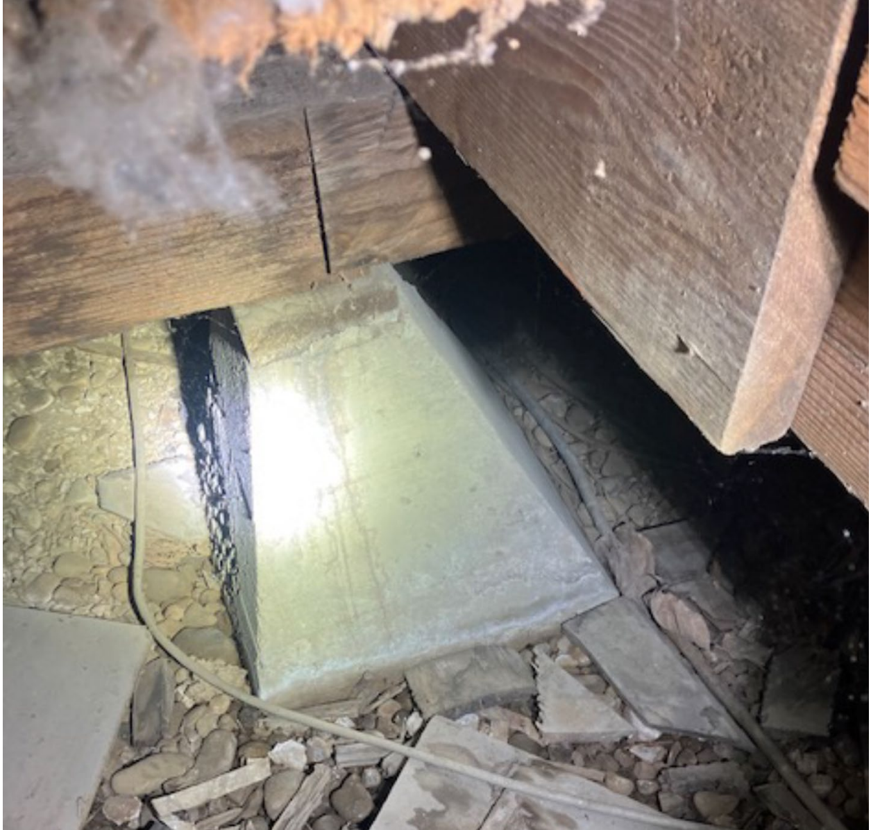
Figure B14. Detail photograph of one of the pyramidal concrete piers below the central portion of Building A (©TNSDS 2023).
