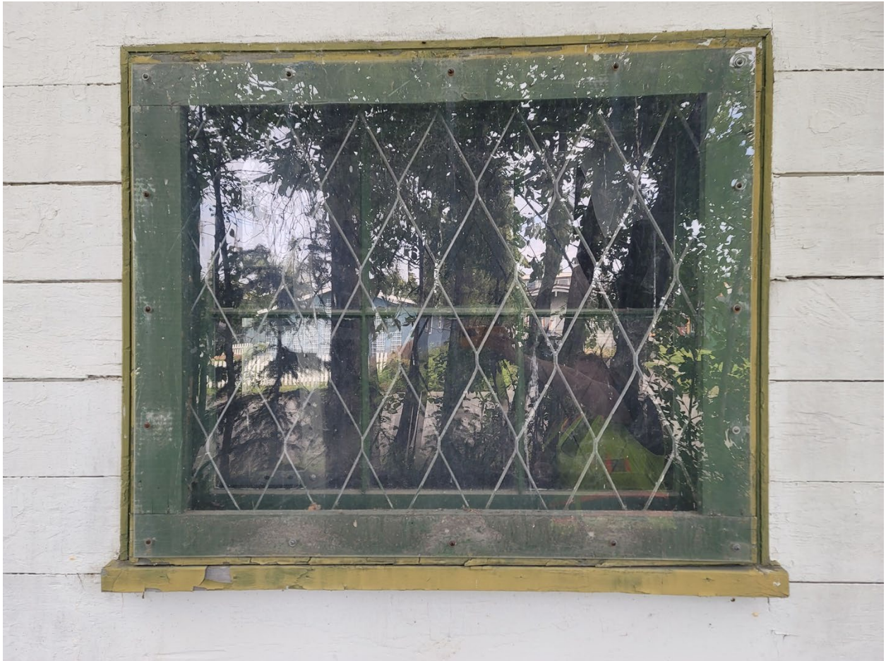
Figure B39. One of the three-over-three wood framed windows on Building C (©TNSDS 2023).
