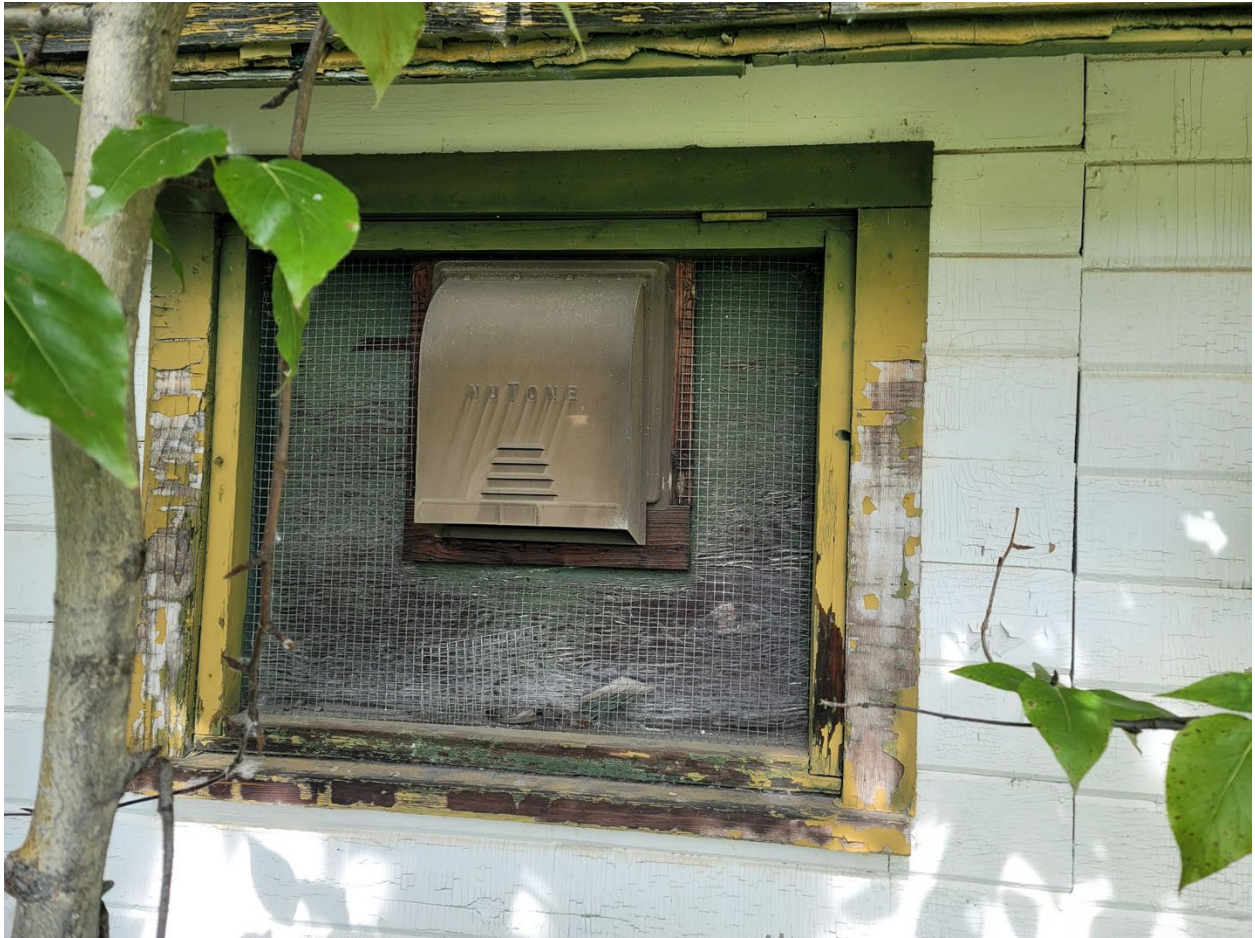
Figure B35. Infilled window in the southeast façade of the addition on Building B (©TNSDS 2023).
