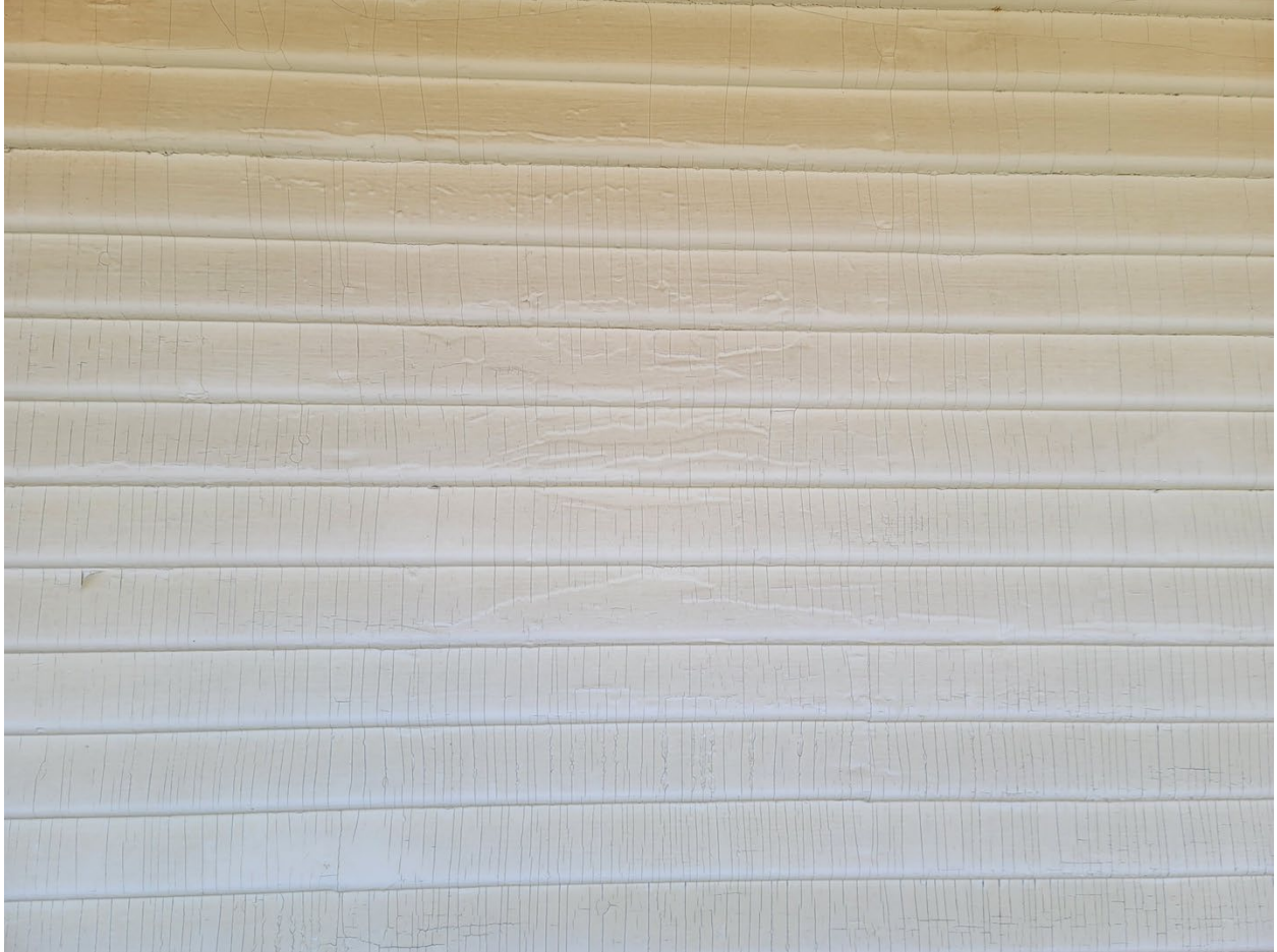
Figure B18. The wrinkling, crazing, and peeling in the paint on the west façade of Building A (©TNSDS 2023).
