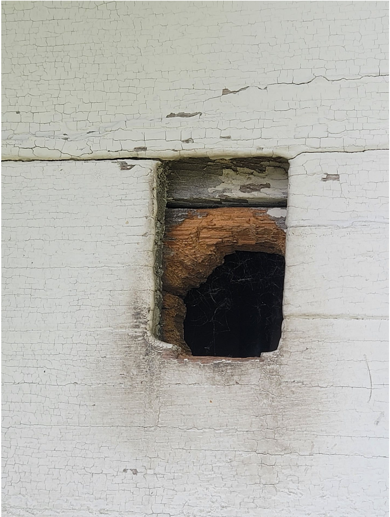
Figure B21. Detail photograph of an opening the siding of Building C, exposing the interior wood planks (©TNSDS 2023).
