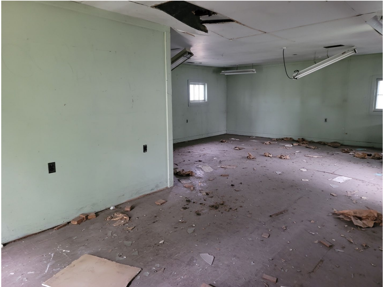
Figure B55. View of the interior of Building C, showing the flooring, wall finishes, and deteriorating ceiling (©TNSDS).
