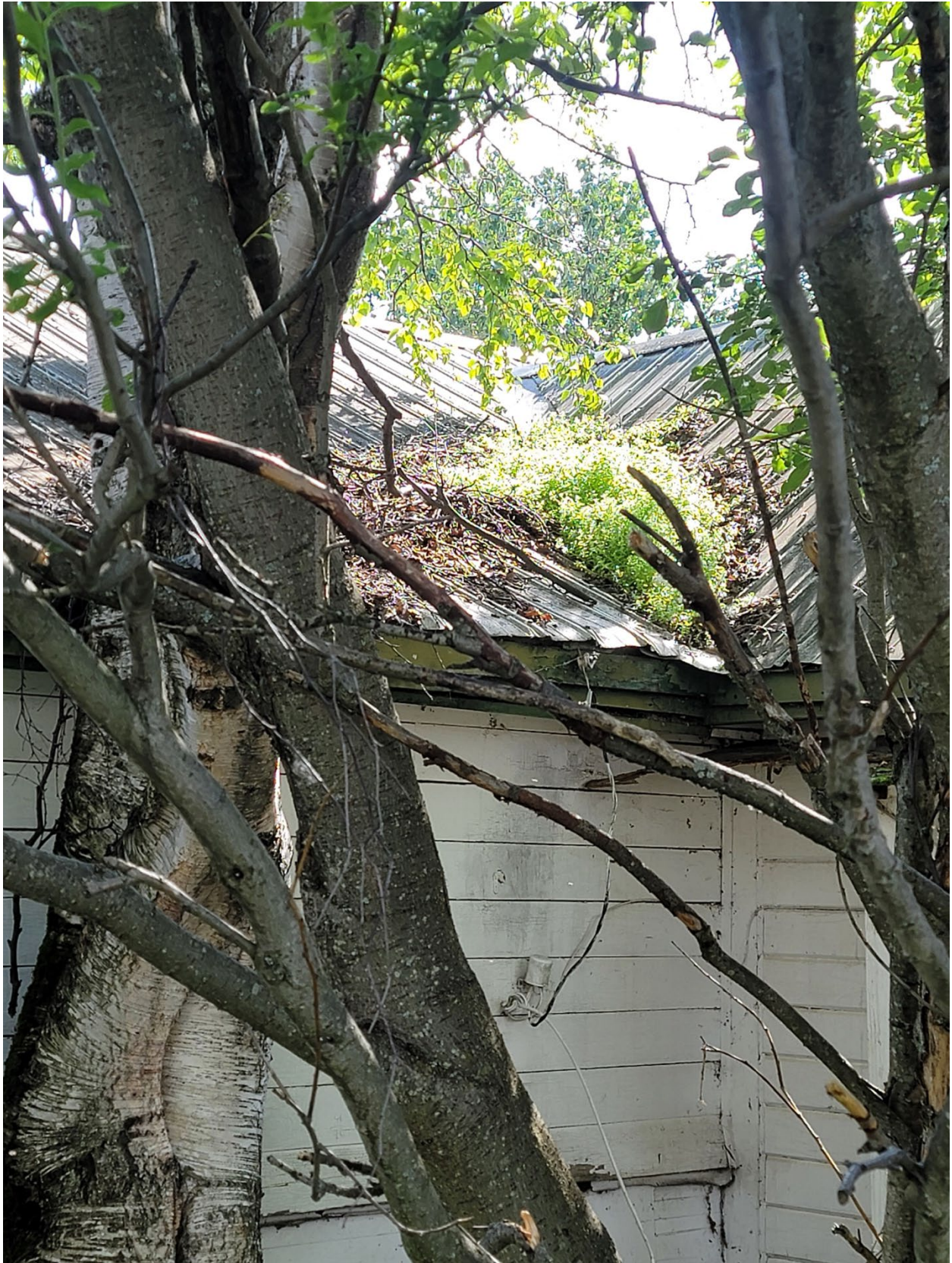
Figure B49. Detail photograph of the junction of the two sections of Building B. The photograph shows the roofing material, surrounding vegetation, and the vegetative debris growing on the roof valley (©TNSDS 2023).
